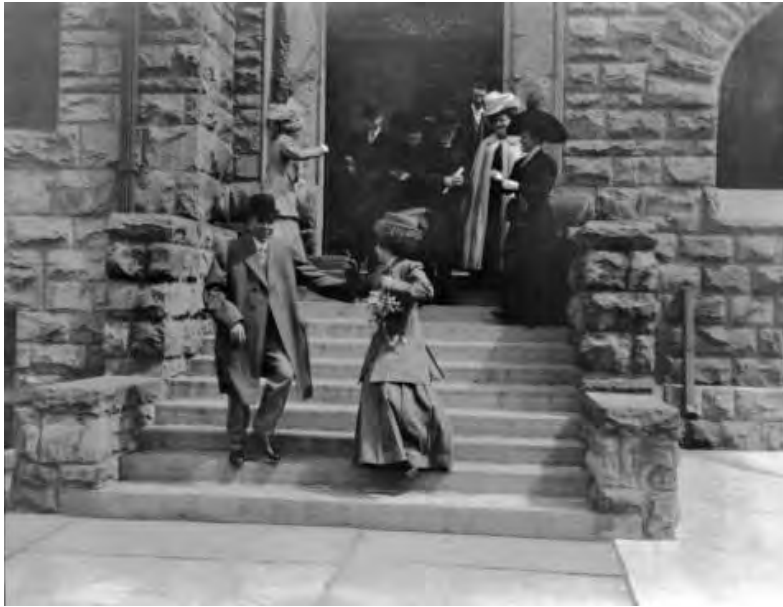
H3: Original stair to main entrance configuration, as seen in 1910 following wedding of Hazel Rhoads and Charles C. Gates. Photo by Harry Mellon Rhoads. Source: Denver Public Library, Western History.
