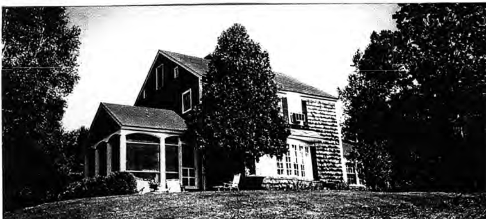
Facing northeast toward the Dickison House in its original form (#87). c. 1960
