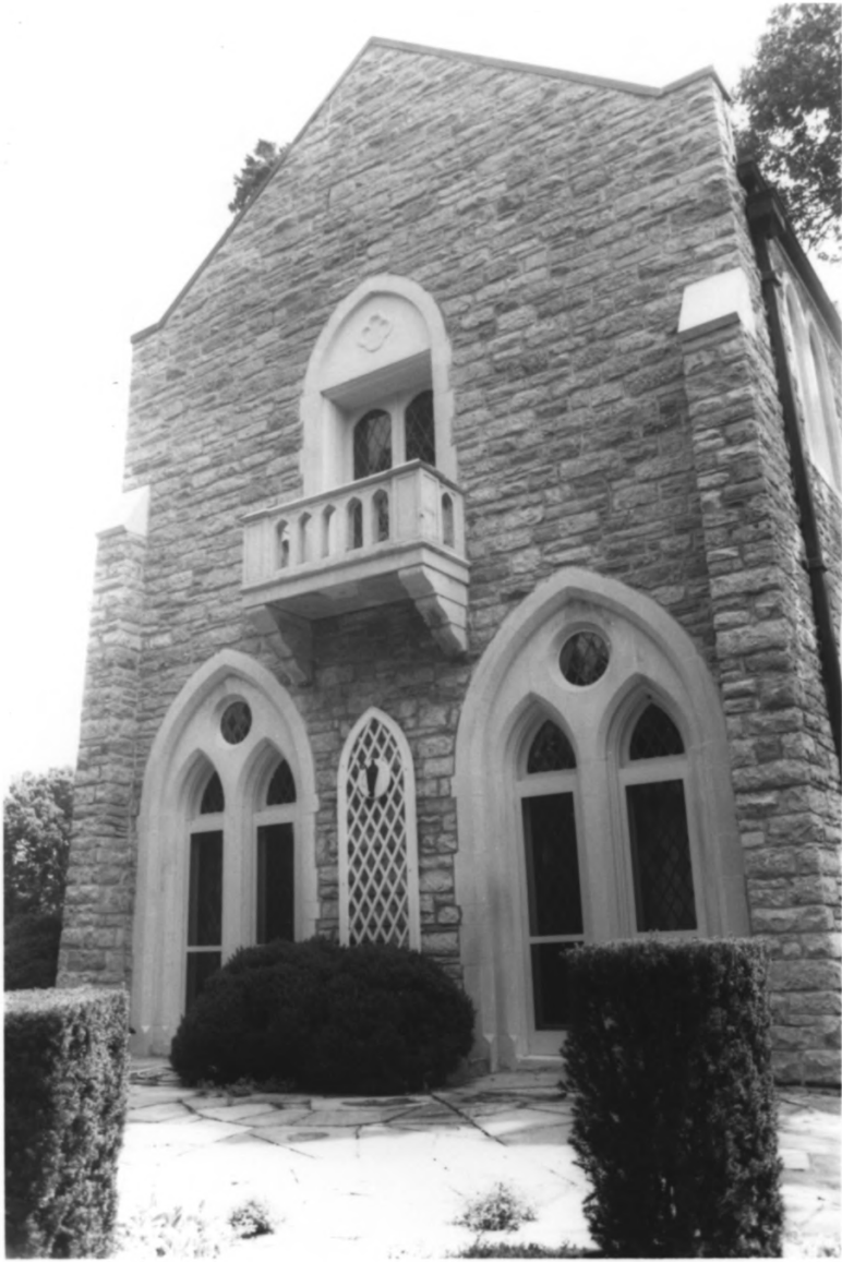
Dudley, Guilford, Sr. and Anne Dallas, House Davidson County TN
