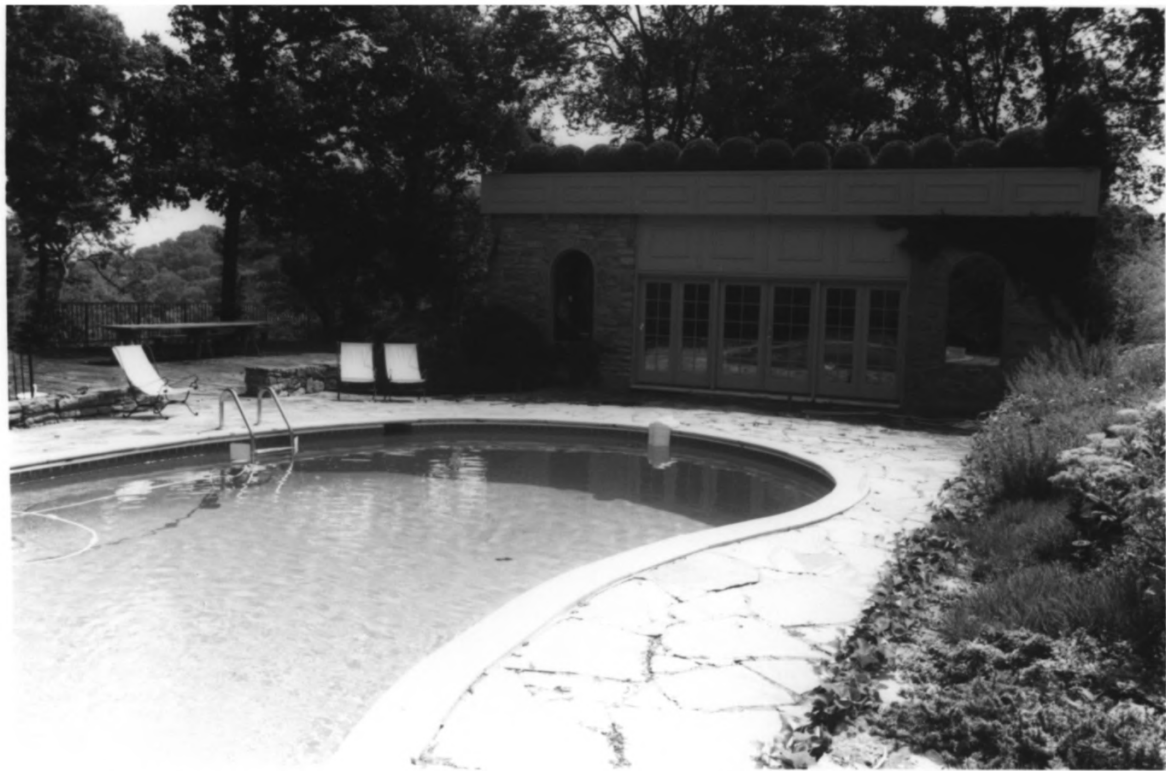
Dudley, Guilford, Sr. and Anne Dallas, House Davidson County TN
