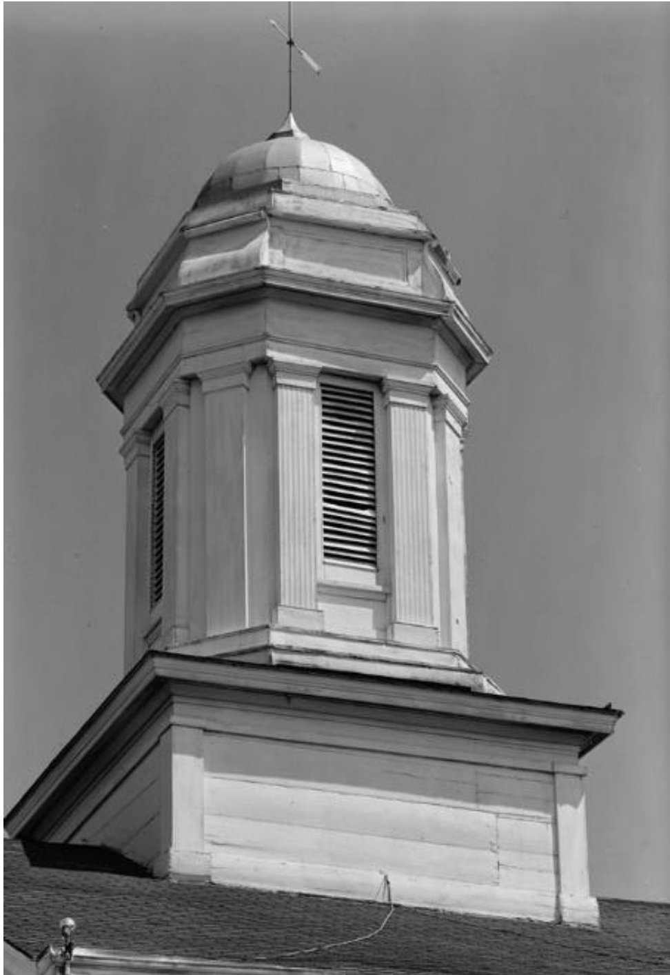
Photograph of the tower and spire from the 1983 Historic American Buildings Survey.
