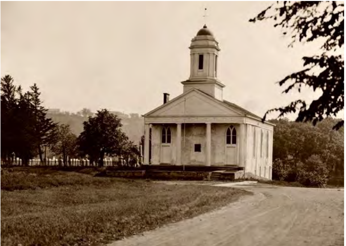
First Presbyterian Church, Lewiston, New York. Undated historic photo looking southeast. This picture shows the church after the 1844 renovation that relocated the central entrance to two doors at either end of the front façade and added a Doric-columned portico, tower and spire.
