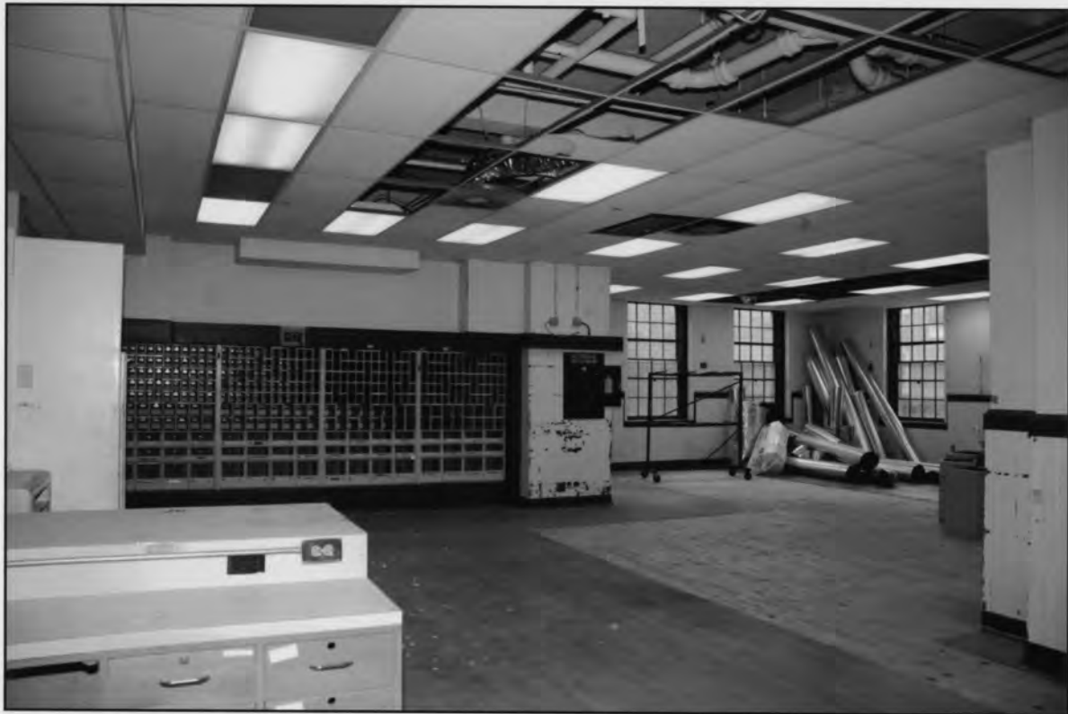
Guntersville Post Office Building Guntersville, Marshall County, AL David B. Schneider October 2009 411 E. 6th St., Anniston AL 36207
