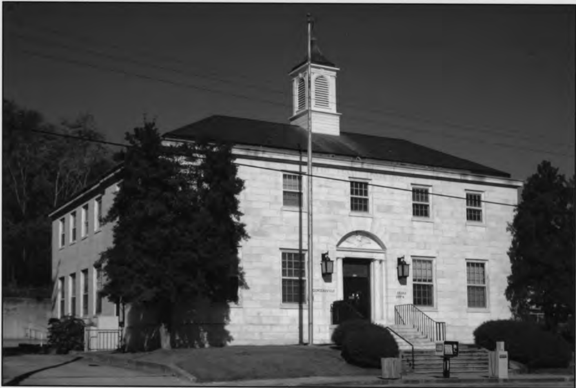
Guntersville Post Office Building Guntersville, Marshall County, AL David B. Schneider October 2009 411 E. 6th St., Anniston AL 36207
