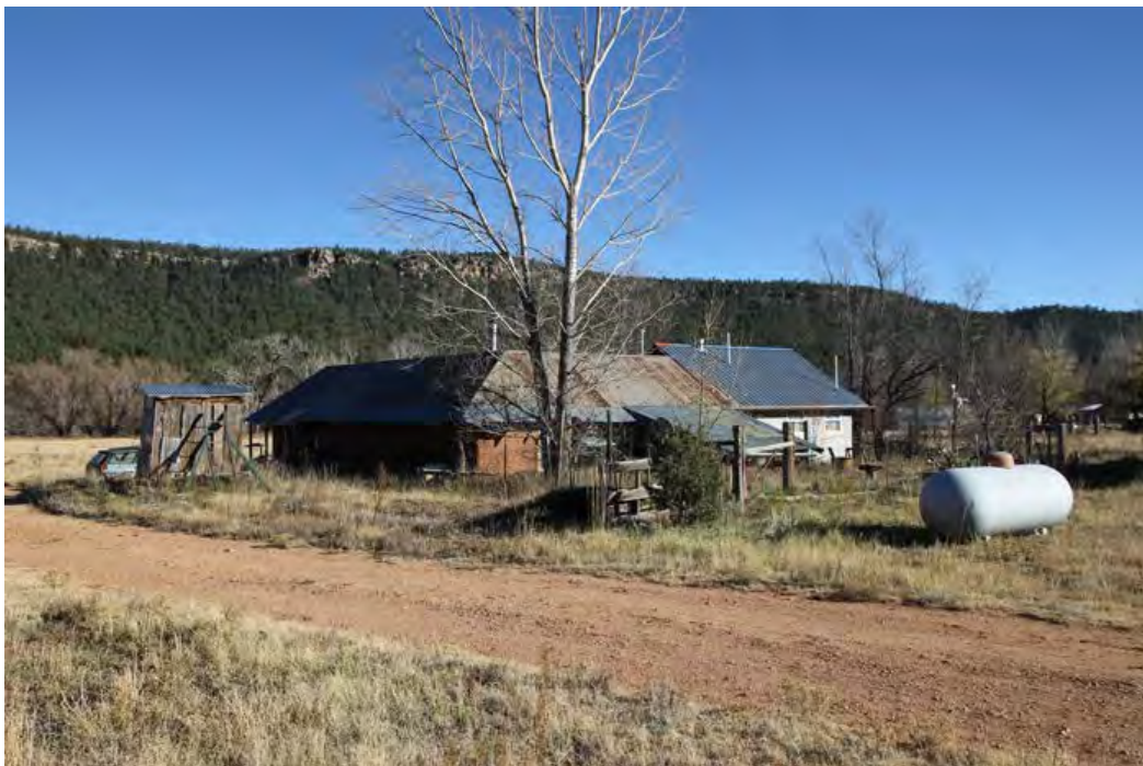
38 of 68. Joseph Ranch, main house and privy, photographer facing southeast.
