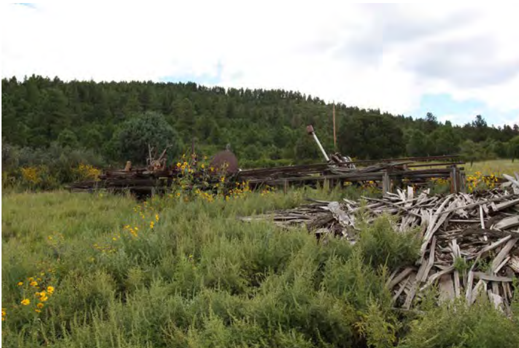
8 of 68. Billy Ortega Lumber Mill near State Route 434, photographer facing north. (Karla McWilliams 2015)
