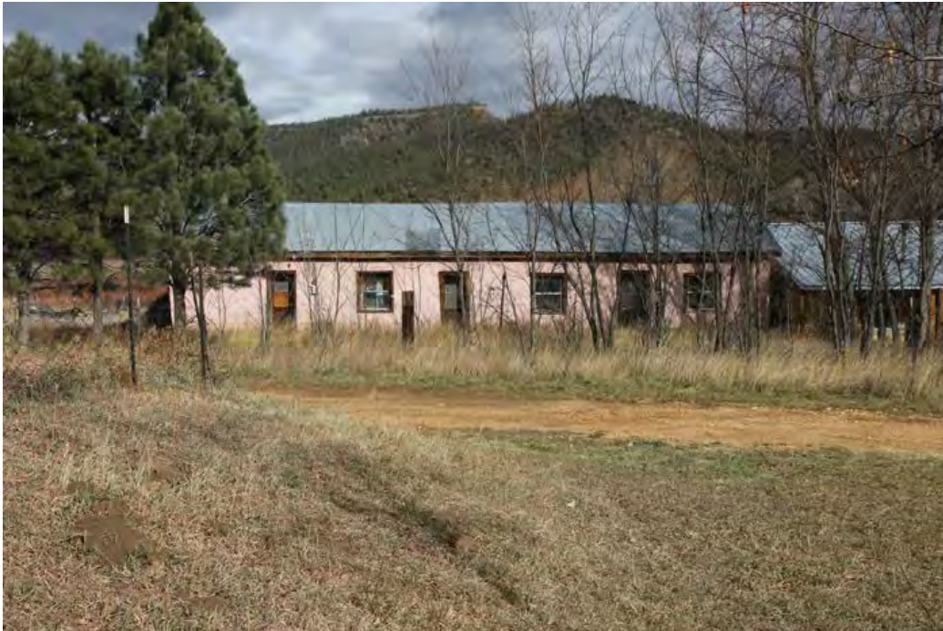
19 of 68. La Ran-Herrera House, Guadalupita, photographer facing east.
