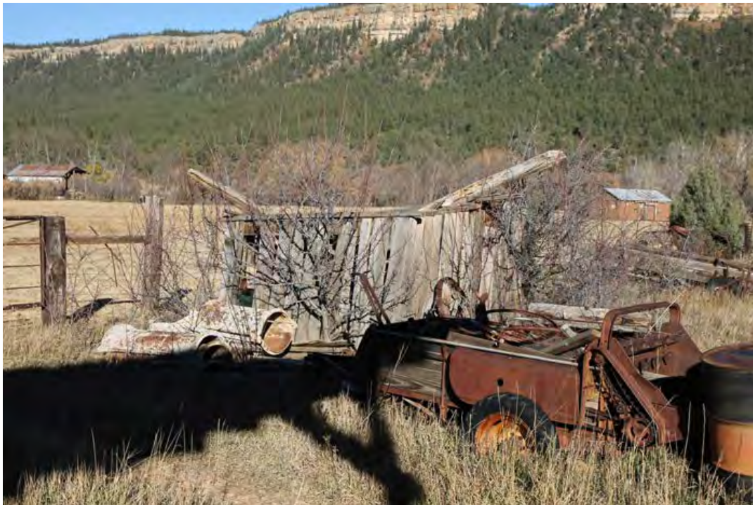
42 of 68. Joseph Ranch, jacal shed, photographer facing northeast.
