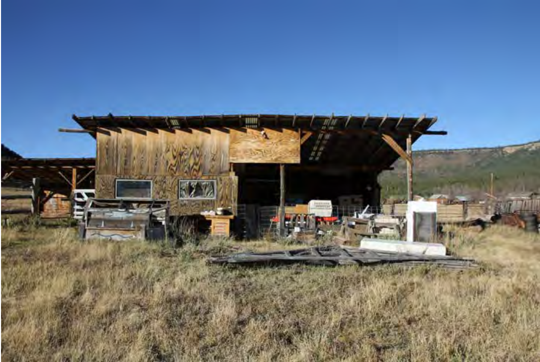
41 of 68. Joseph Ranch, pole barn, photographer facing north.
