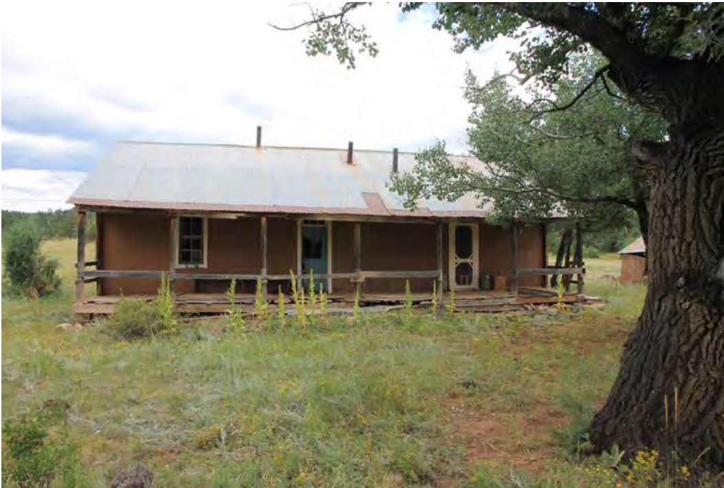
27 of 68. Blas Medina, Sr., House, photographer facing northeast.
