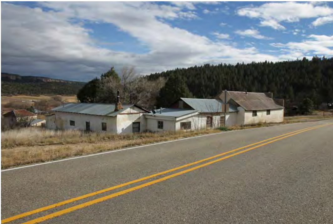
16 of 68. Delfino Griego House and Meeting Hall, Gaudalupita with view to Coyote Creek Valley (left), photographer facing southeast.
