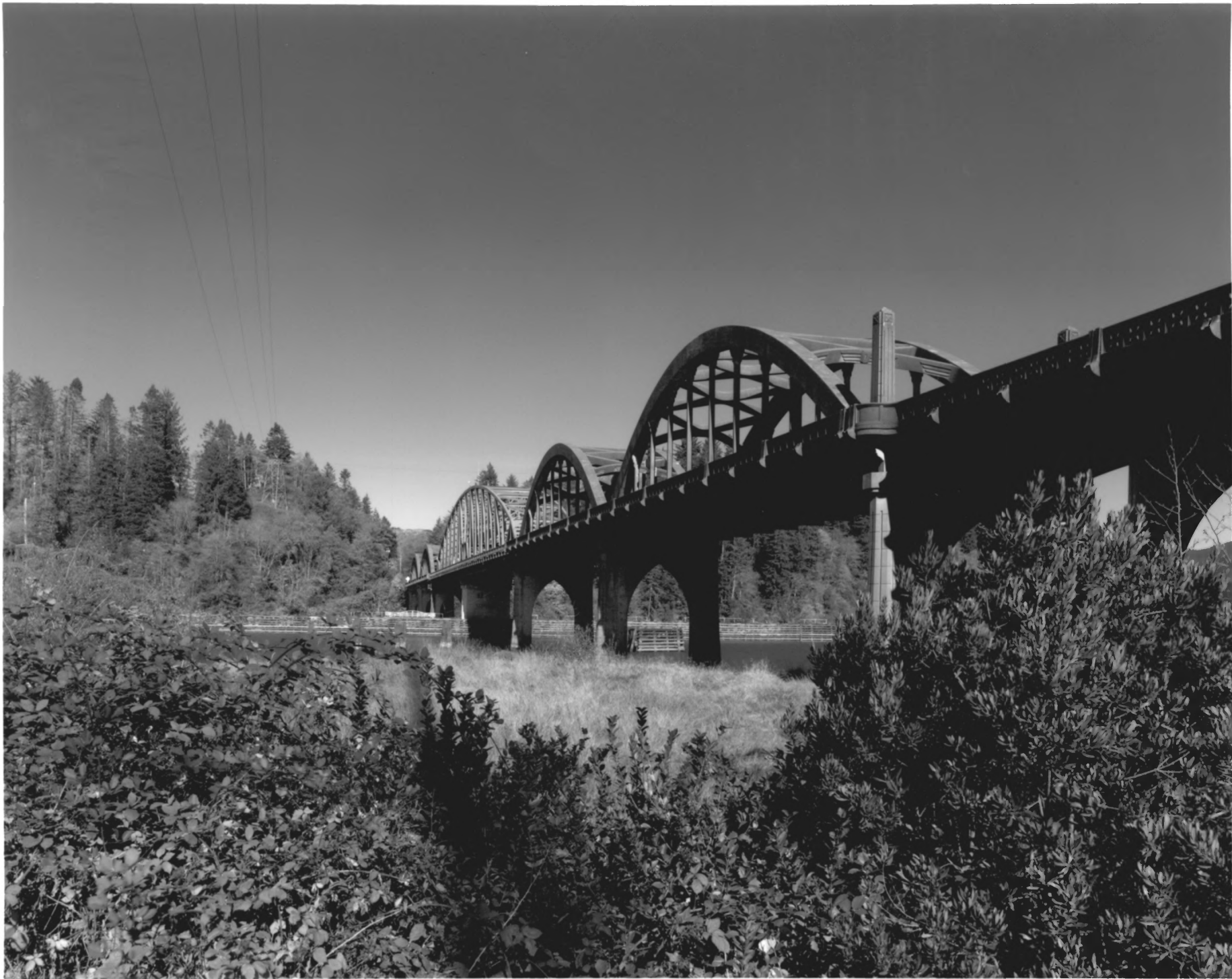
WAPOVA RIVER BRIDGE, REEDSPORT, OREGON
