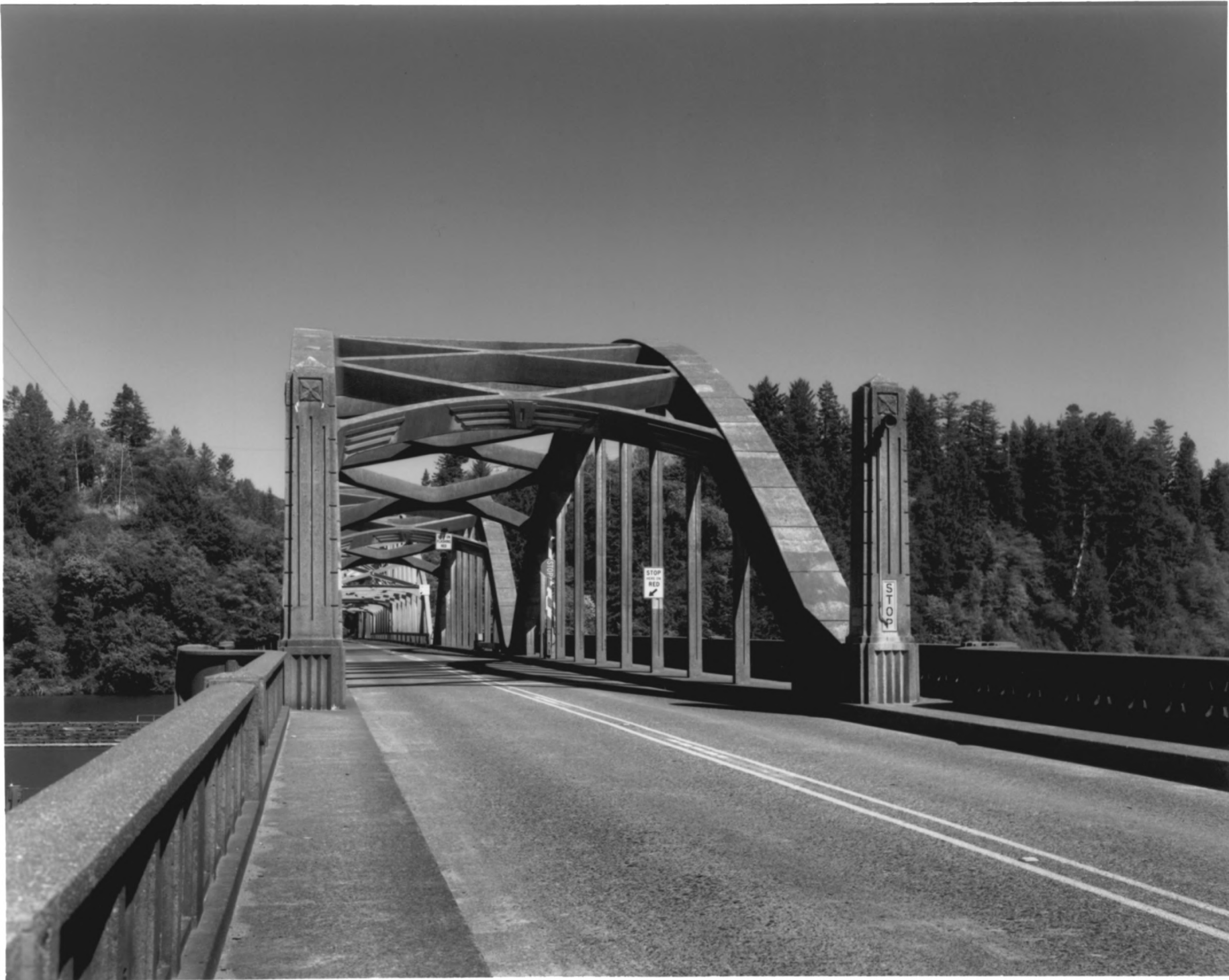
UMPUQA RIVER BRIDGE, REEDSPORT, OREGON
