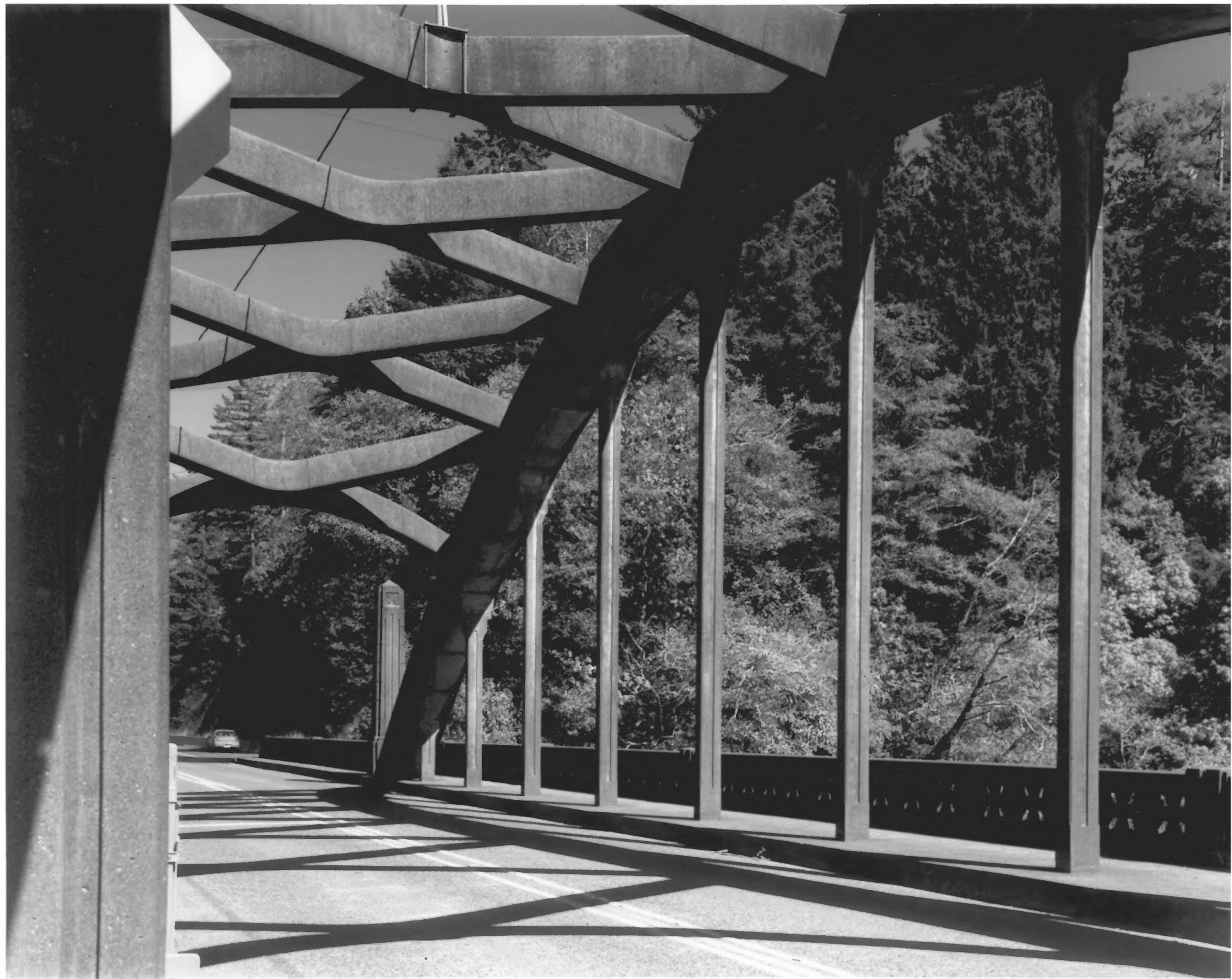
UMPUWA RIVER BRIDGE RECONSTRUCTION #9
