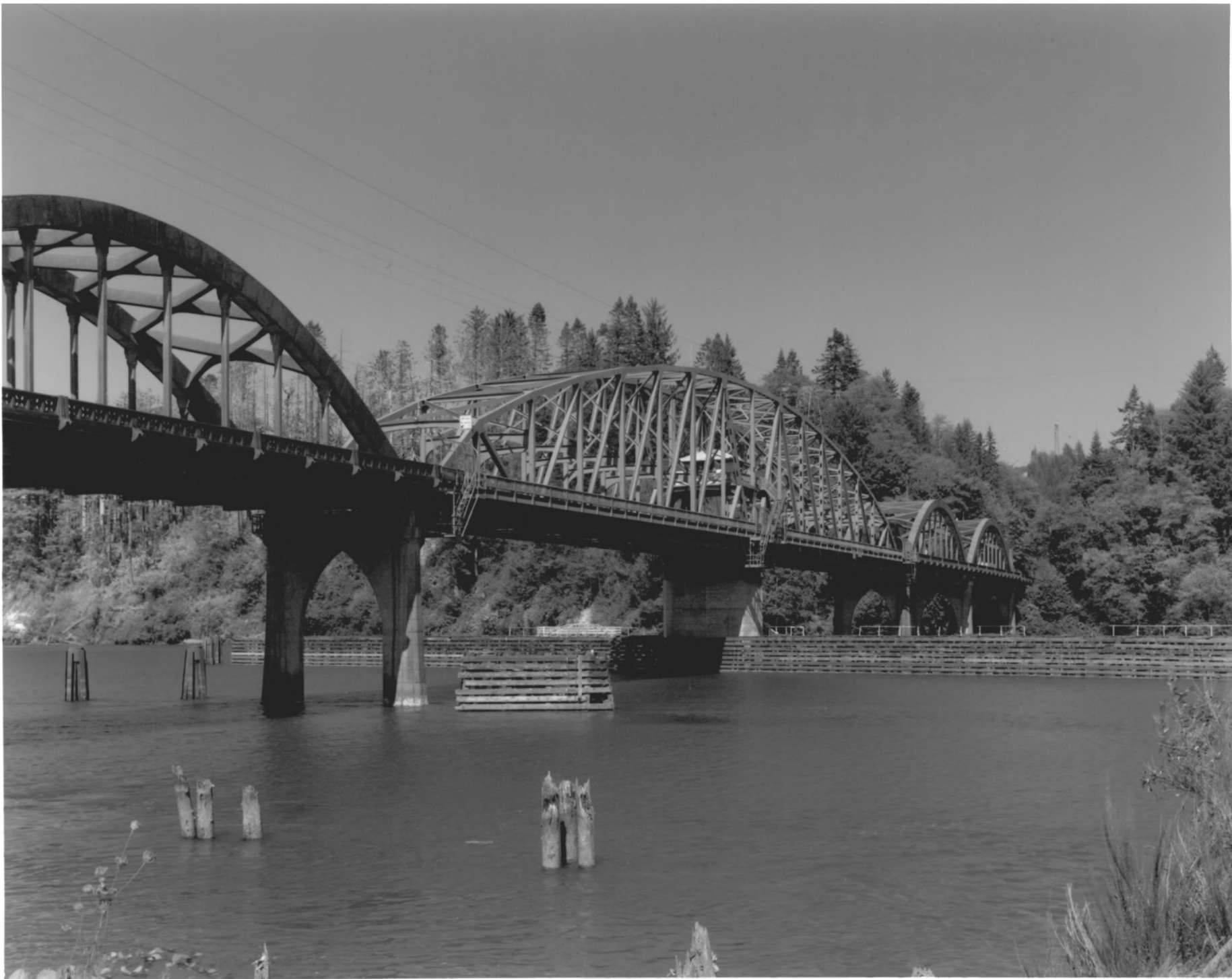
UMPUQA RIVER BRIDGE, REEDSPORT, OREGON #16
