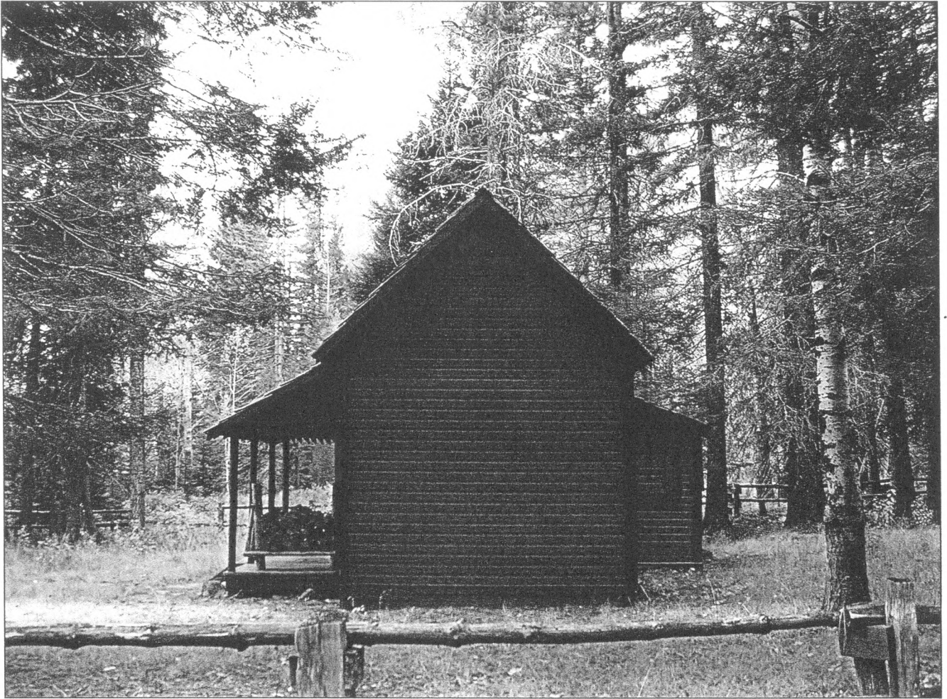
Gotchen Creek Ranger Station Gifford Pinchot National Forest East elevation, with front porch visible at left, enclosed rear porch visible at right, pole fence in foreground, color digital photograph. October 26, 2006 Richard McClure, photographer, USDA Forest Service
