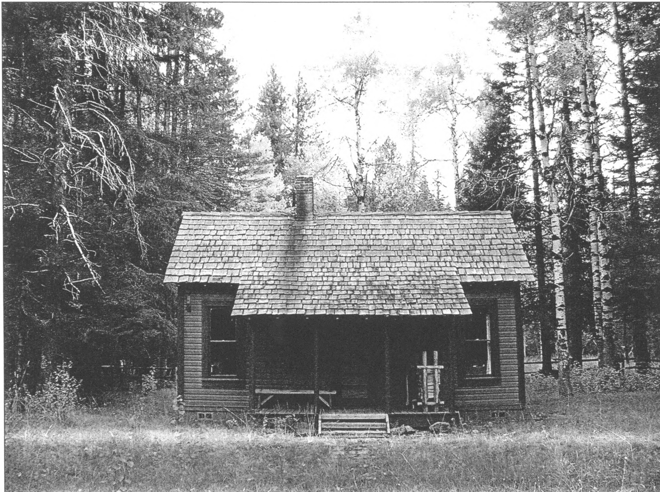
Gotchen Creek Ranger Station Gifford Pinchot National Forest Main façade (south elevation), color digital photograph. October 26, 2006 Richard McClure, photographer, USDA Forest Service
