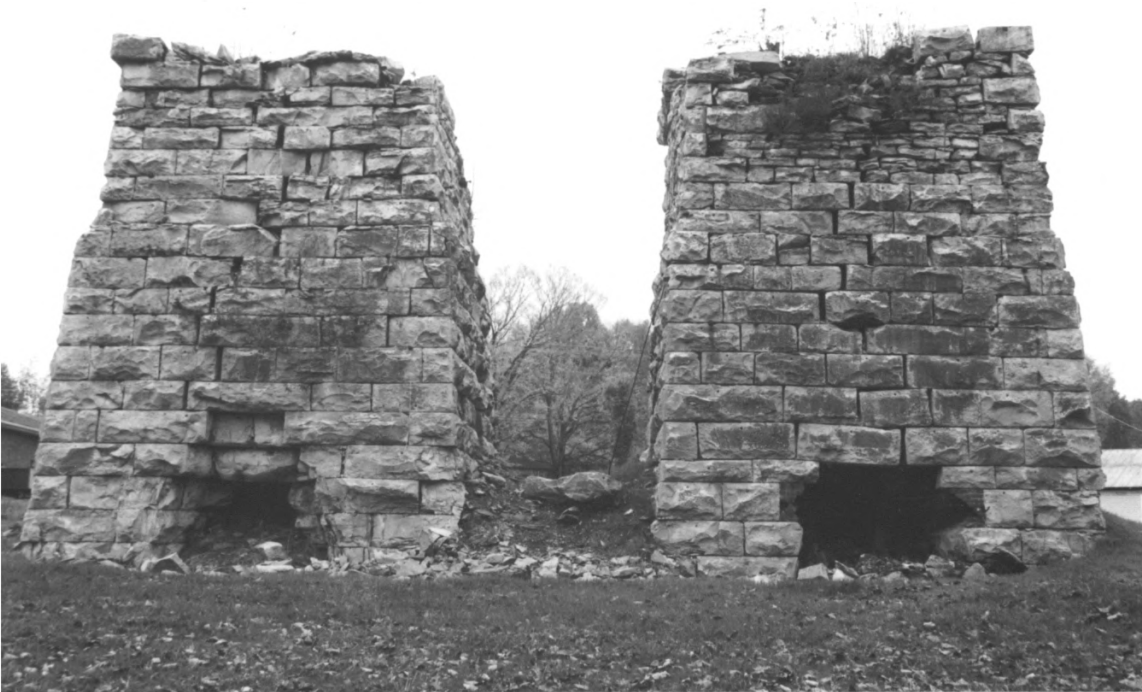
ERIN LIMEKILNS HOUSTON COUNTY TN
