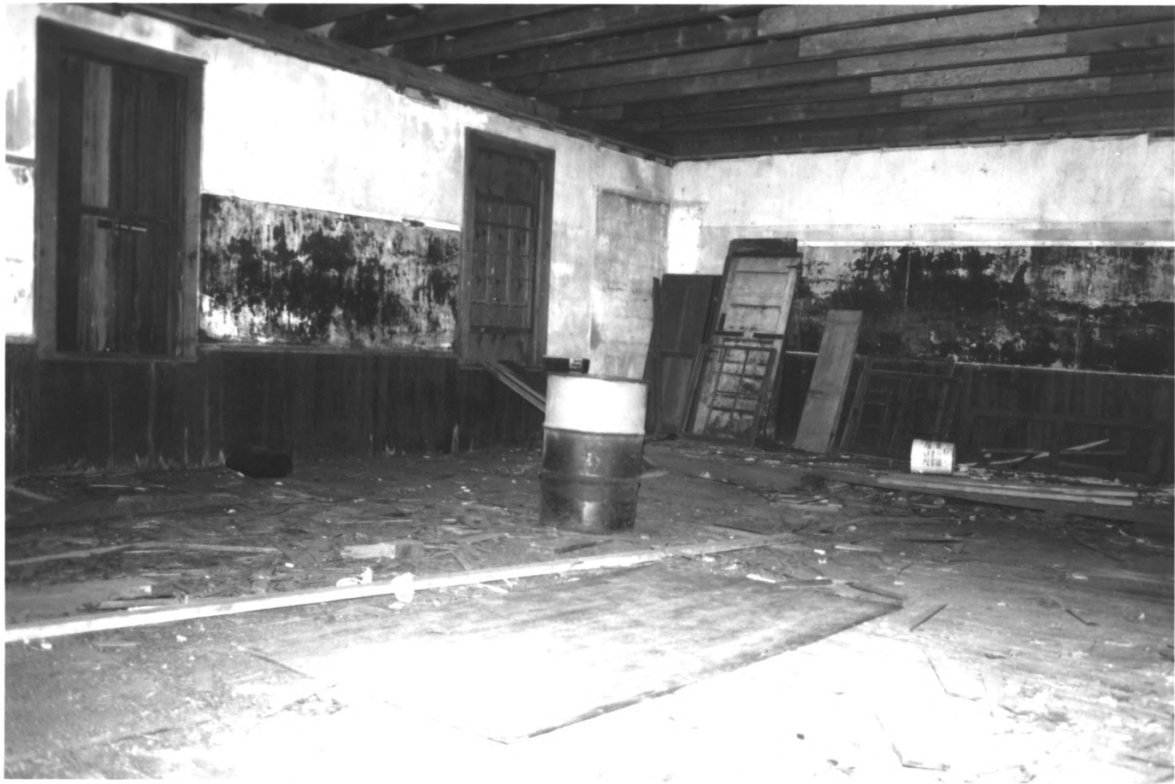
BIRMINGHAM SCHOOL, BURLINGTON COUNTY, NJ PHOTO # 6 OF 8
