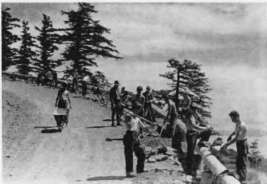
Constructing guardrails on Mt. Constitution Road (ID#58). WSPRC Photo 75-SP1-216.
