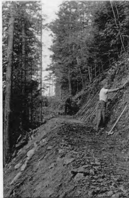
Hand scaling slopes on Mountain Lake Trail, 1934. WSPRC Photo 75-SP1-150.
