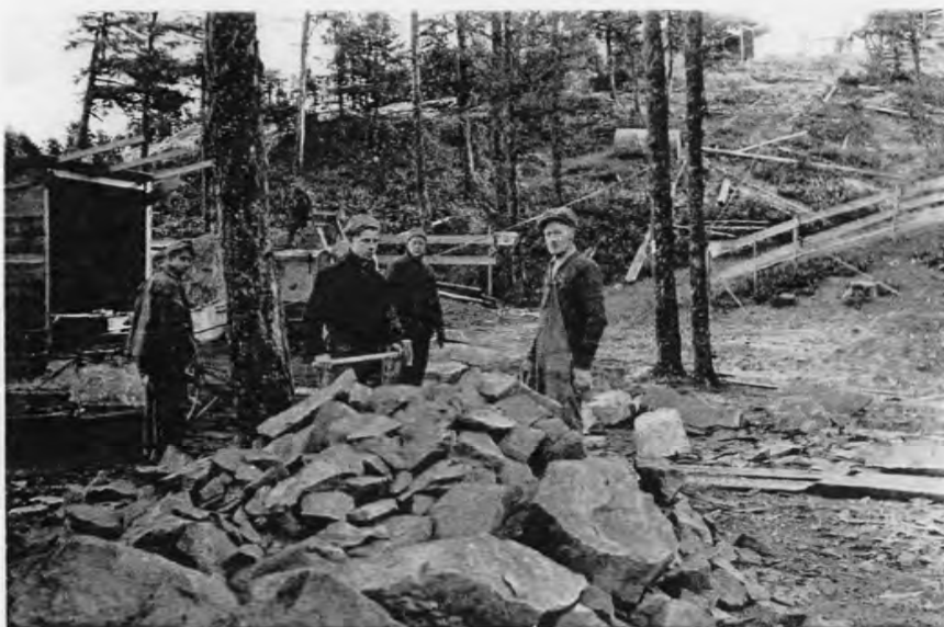
Shaping stone for the Mt. Constitution Tower, November 1935. WSPRC Photo 75-SP1-254.
