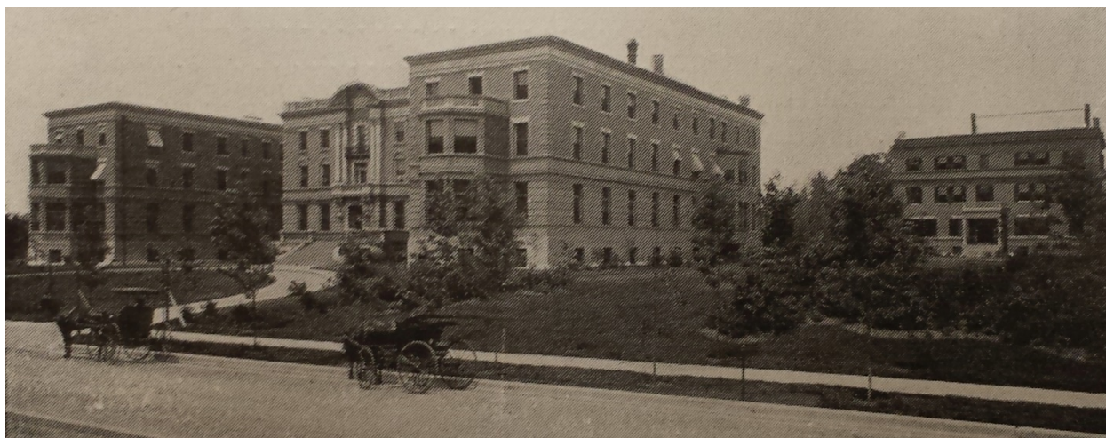
Figure 10: St. Luke's Hospital (left) and original Nurses' Home (right, demolished) after 1904 move to 5535 Delmar Boulevard. Source: St. Luke's Hospital Annual Report, 1913.
