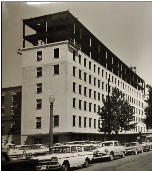
Figure 30: the differentiation of old and new brick above the fifth story is clear in this 1961 photo of the upper story addition to the Fowler Wing. Source: St. Luke's Hospital photo files.
