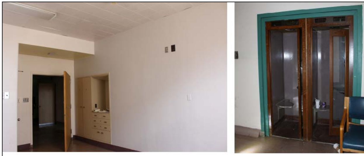
Figure 33: North Building patient room, left, and telephone booths. Federal guidelines did not go so far as to lay out specifications for phone booths... but they do mention that there should be phone booths ( Design and Construction of General Hospitals , 49), Photos by Elyse McBride, March 2017.
