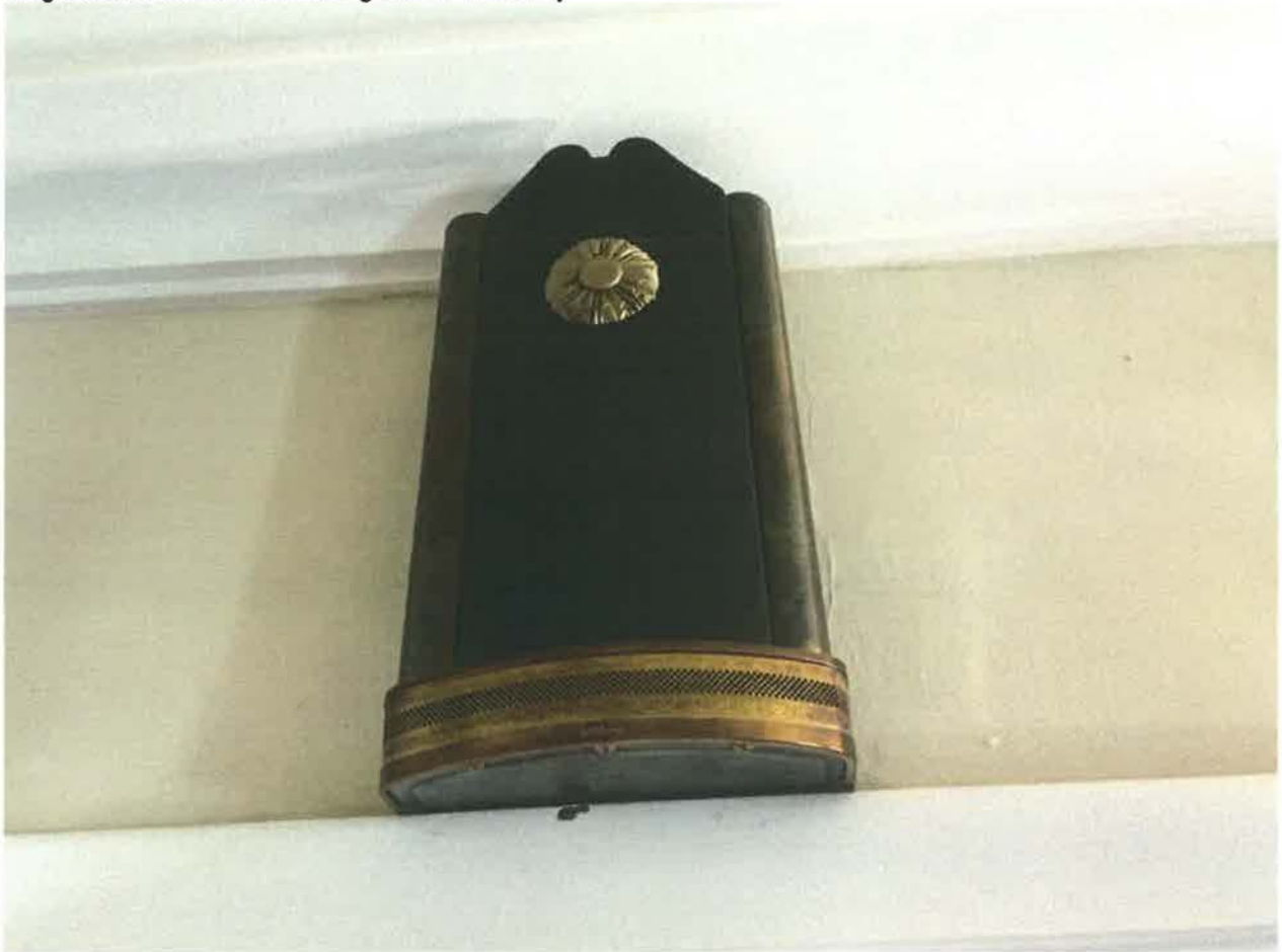
Photo 18 The Borah House Maricopa County, Arizona Original Doorbell above Dining Room Doorway
