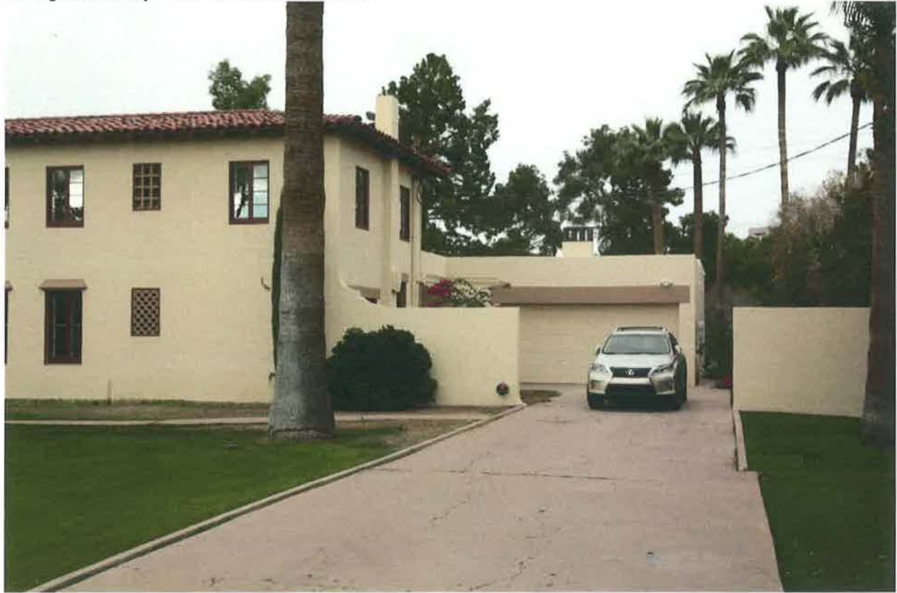
Photo 2 The Borah House Maricopa County, Arizona Garage/Driveway – Camera Direction North
