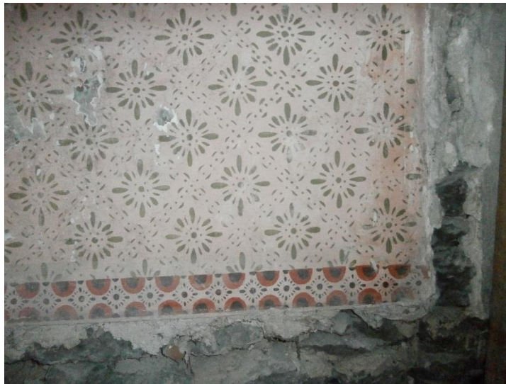
Figure 2. Early nineteenth-century stenciling on exterior parged wall of formal dining room
