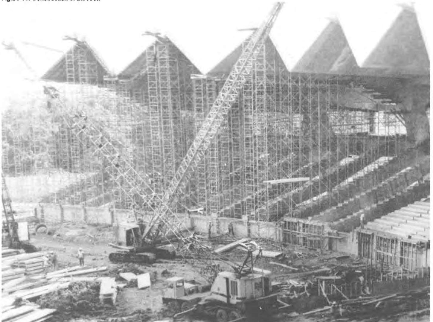
Figure 13. Construction of the roof.
