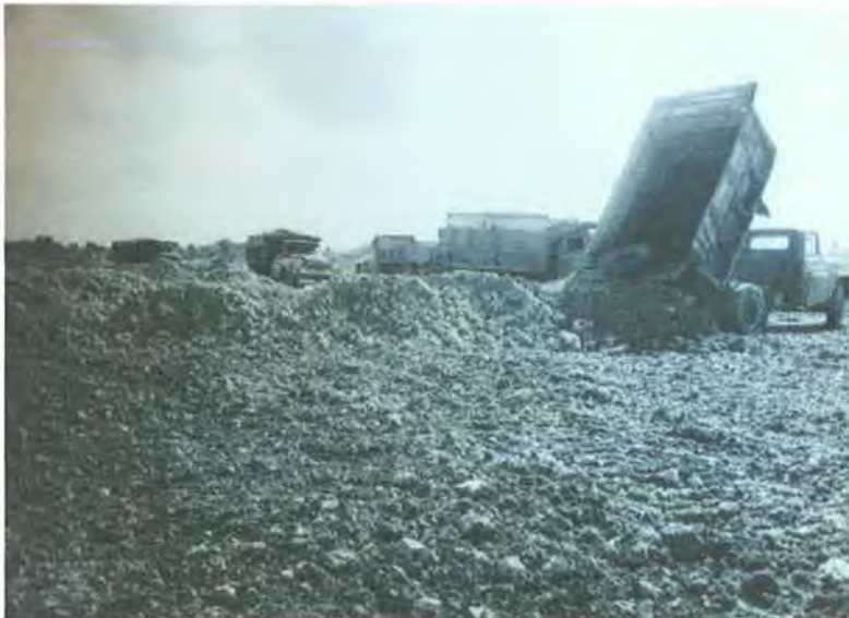
Figures 10/ 11. Filling and leveling the site.
