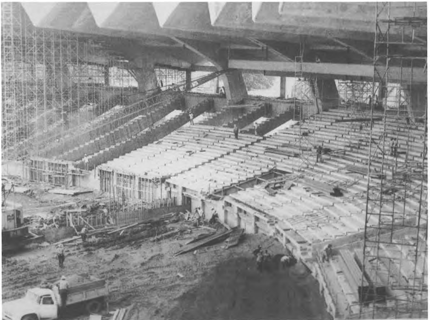
Figure 14. Installation of the prefabricated stands.
