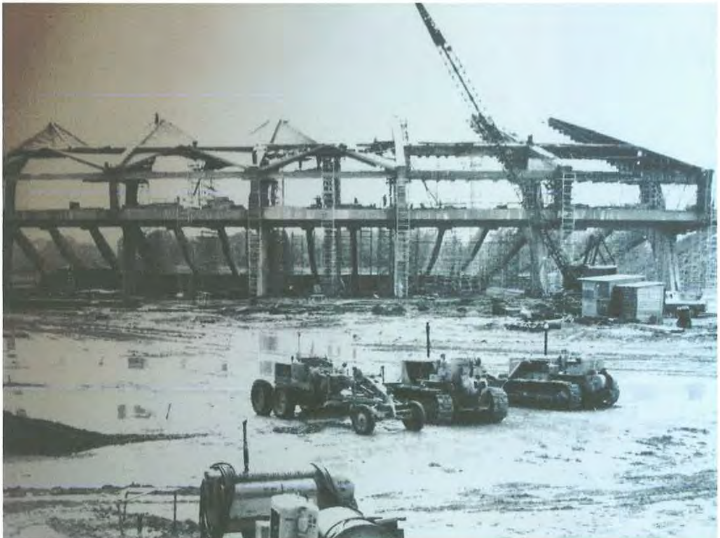
Figure 12. Joining the foundation and supporting elements frames with the concrete beams.
