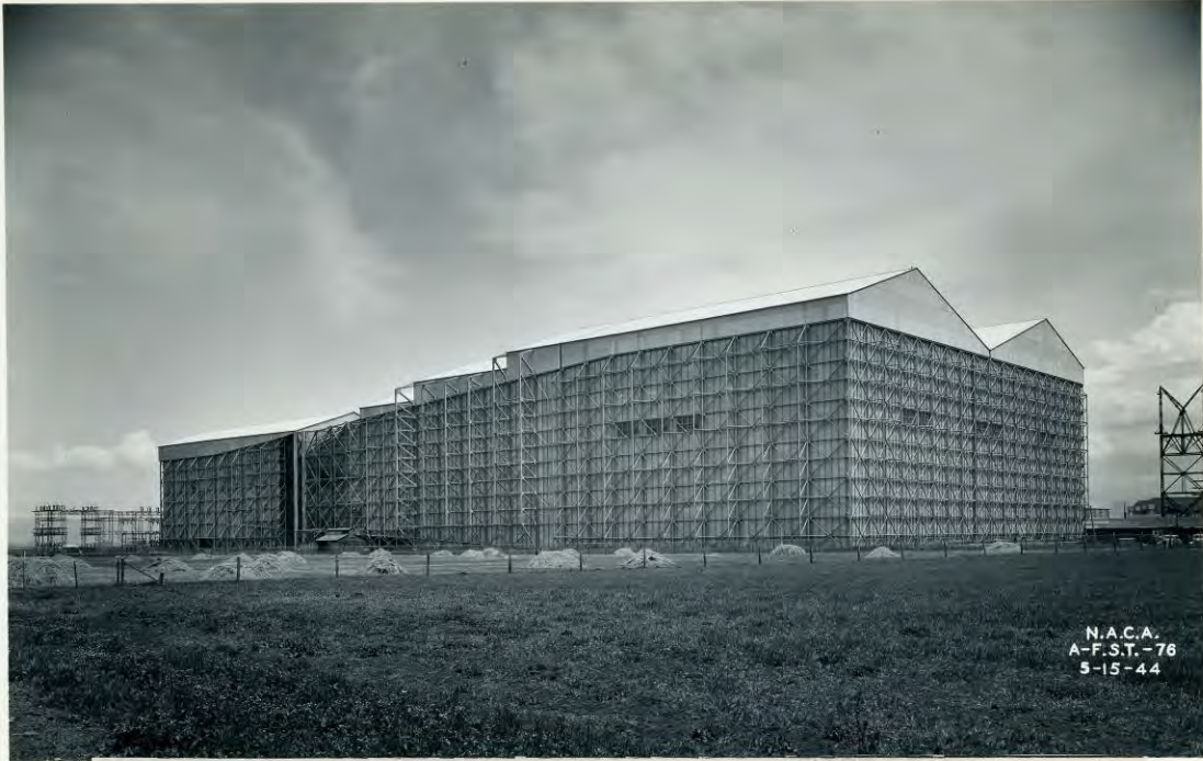
Outside view of the 40 x 80 Foot tunnel at Ames. This is the world's largest wind tunnel, is powered by six 6,000 hp. motors--provides speeds up to 250 mph.
