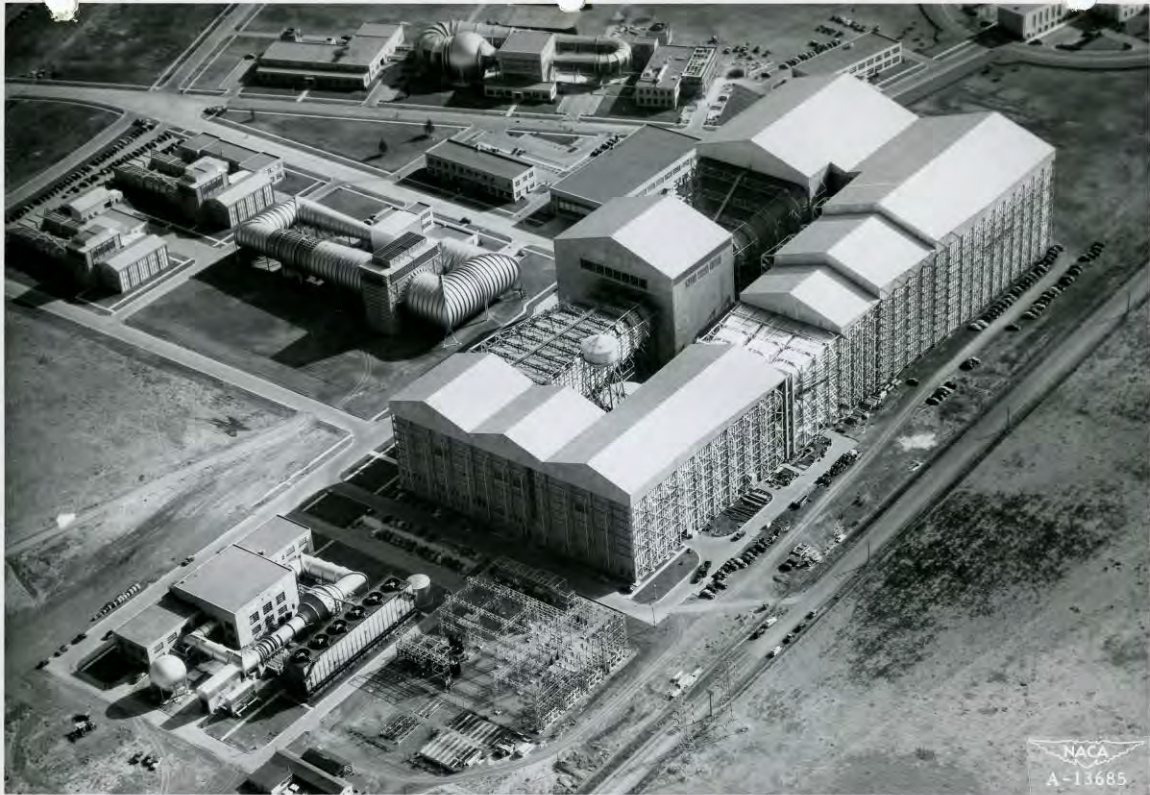
The new 6- by 6-foot Supersonic Wind Tunnel in the left foreground has recently been placed in operation at the NACA's Ames Aeronautical Laboratory, Moffett Field, California. With a speed range from 1.1 to 1.8 times the speed of sound, it helps to fill an urgent need for larger-scale, supersonic research facilities and will play an important role in the development of tomorrow's supersonic aircraft.
