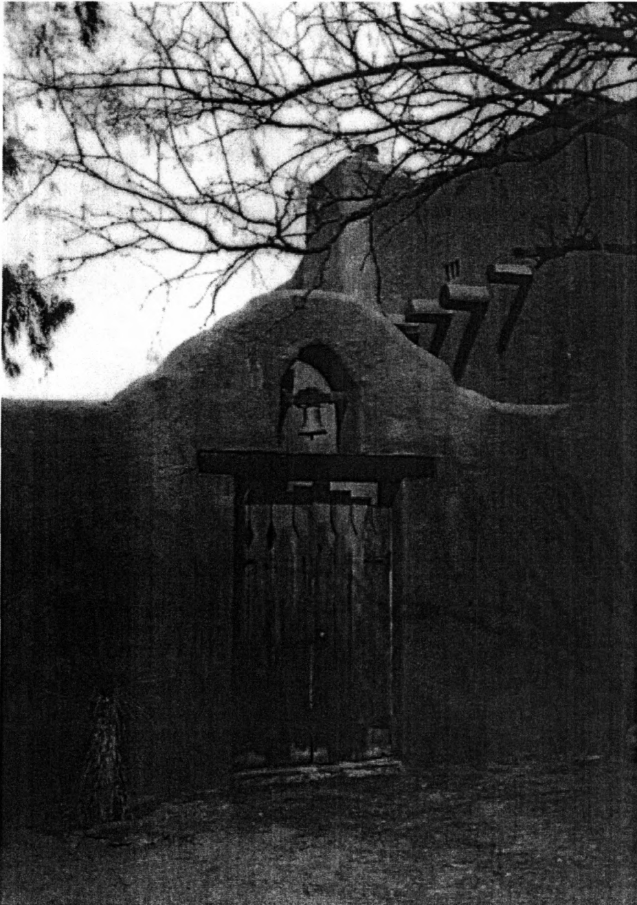
PHOTO #2 (Neg # DWR-29): Patio gate and belfry looking NW
