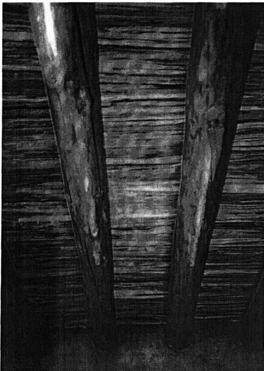
PHOTO #24 (Neg # DWR-25): Interior living room ceiling with vigas and saguaro rib latillas
