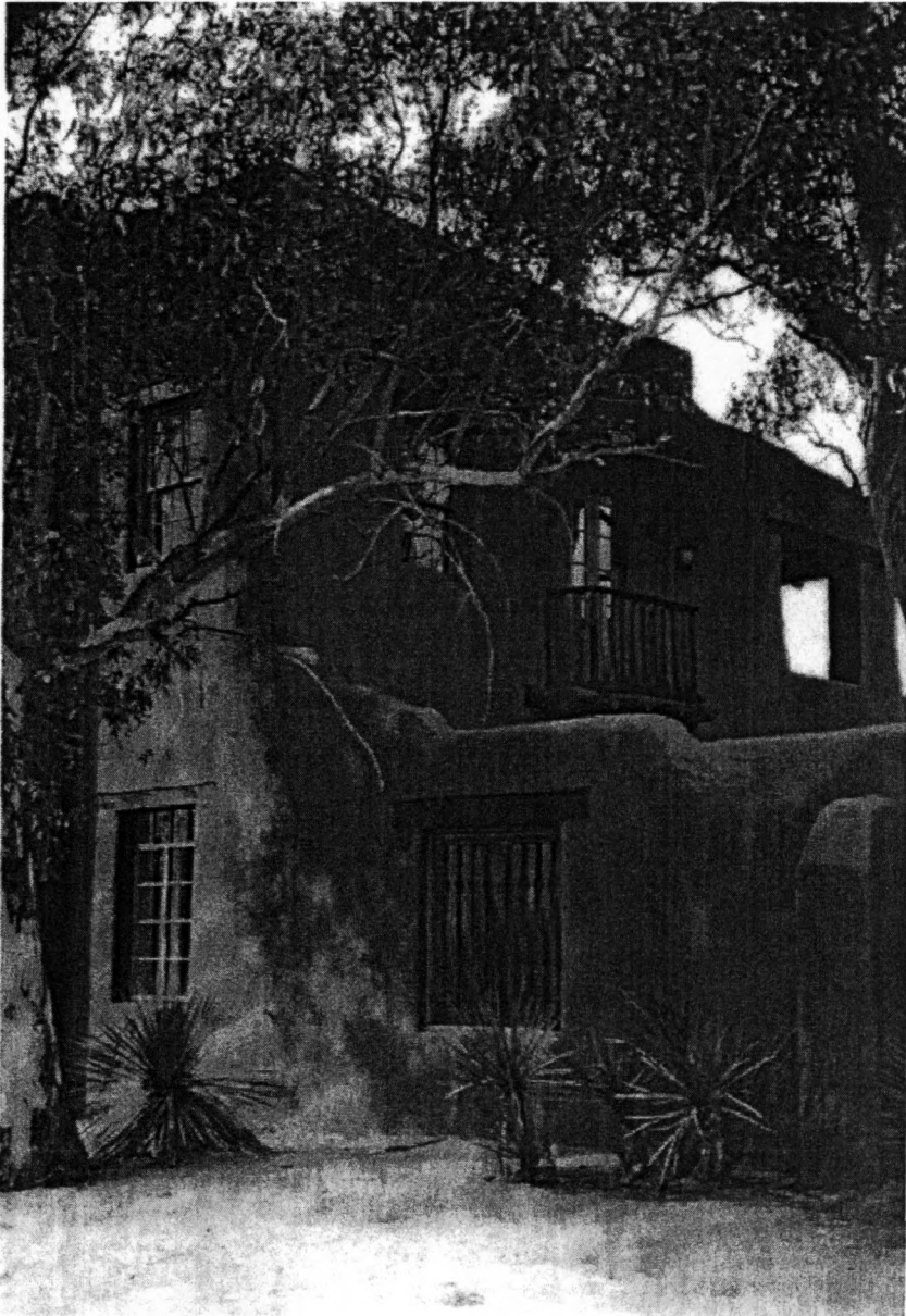
PHOTO #4 (Neg # DWR-30): South and east facades of west building looking NW
