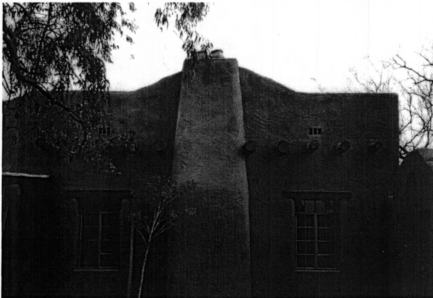
PHOTO #5 (Neg # DWR-14): Partial west façade of East Building from Patio looking East
