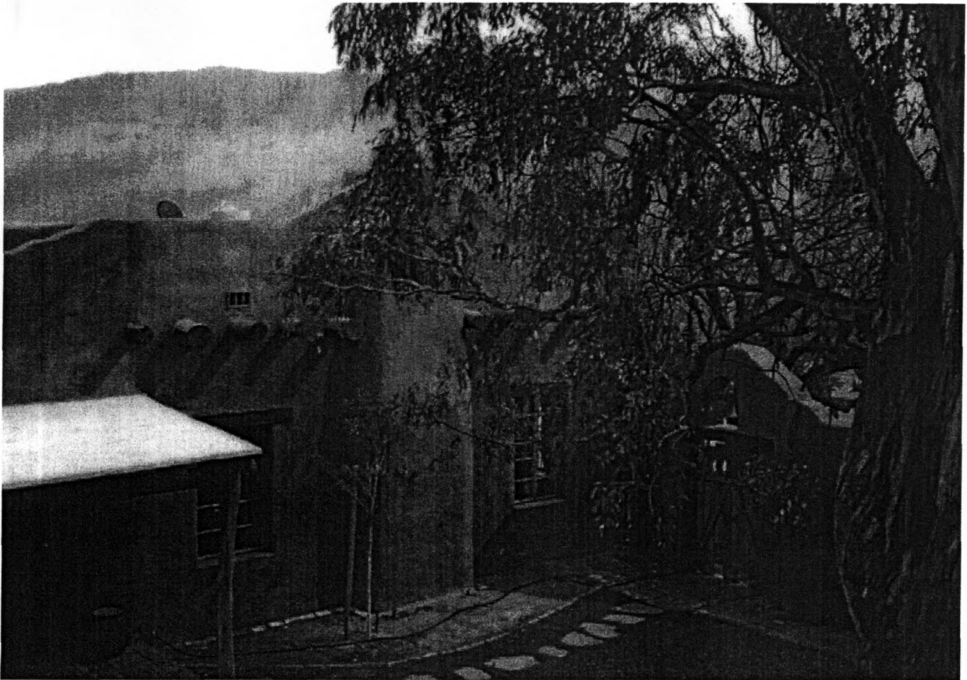
PHOTO #16 (Neg # DWR-5): View of Patio from second story roof deck looking SE
