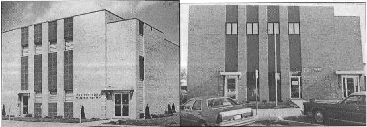
Figure 51: Interior Telephone Building, view northeast (Grinnell Herald-Register , August 6, 1956 and Naumann, 1988, right)
