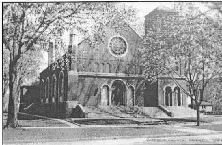
Figure 38: St. Marys Roman Catholic Church, 1000 Broad Street, view southeast
