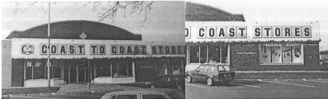
Figure 33: 1013 Broad, view northeast (Naumann, 1988)
