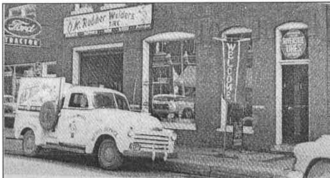
Figure 40: 806-08 Main Street, view southeast (1960 Grinnell City Directory)
