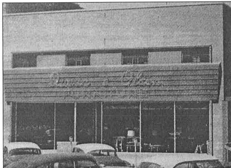
Figure 30: 929 Broad Street, Queen & Olson Furniture, view southwest
