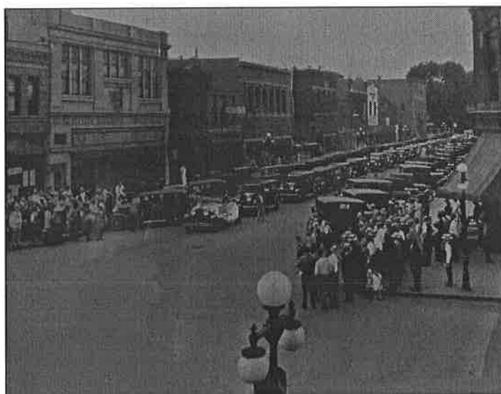
Figure 42: Main Street north of 4 th Avenue, parade of new Whippet Automobiles, 1929, view northwest
