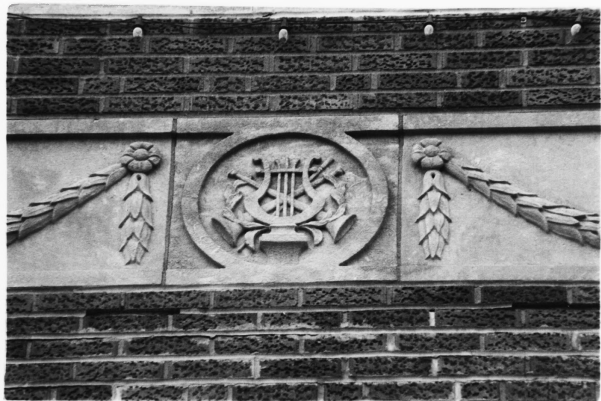
CHARLTON CITY HALL & FIRE STATION LUCAS COUNTY, IA | photo #10
