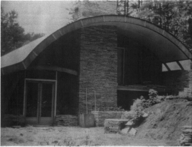
Exterior - north facade
