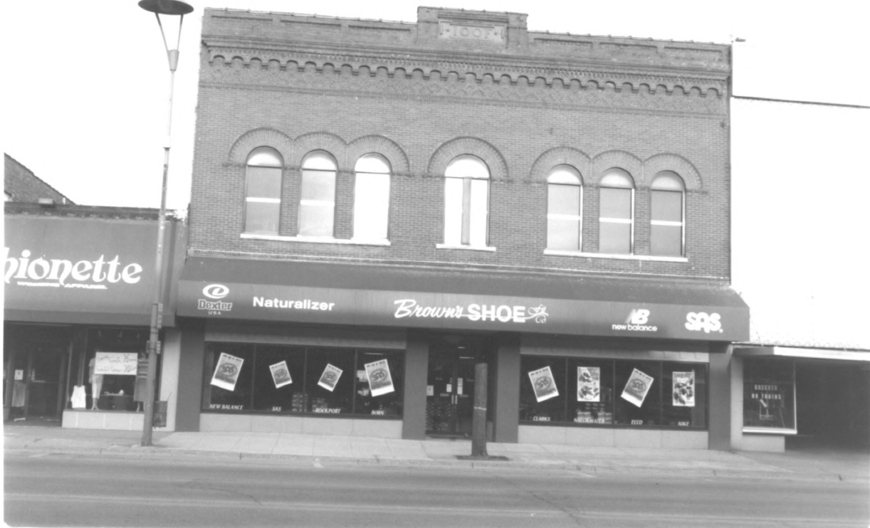
413-415 Grand Av Hist Commercial Dist Clay County, IA PHOTO #13
