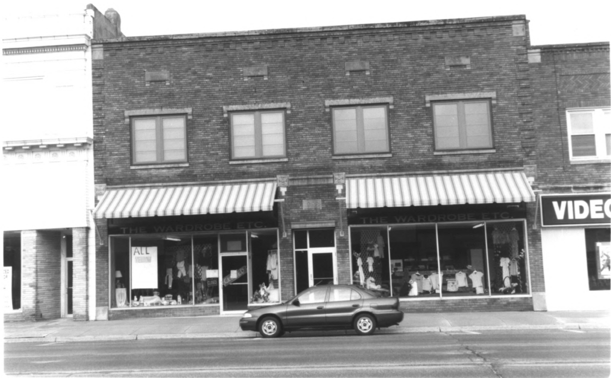
505 Grand Av Hist Commercial Dist Clay County, IA PHOTO # 25
