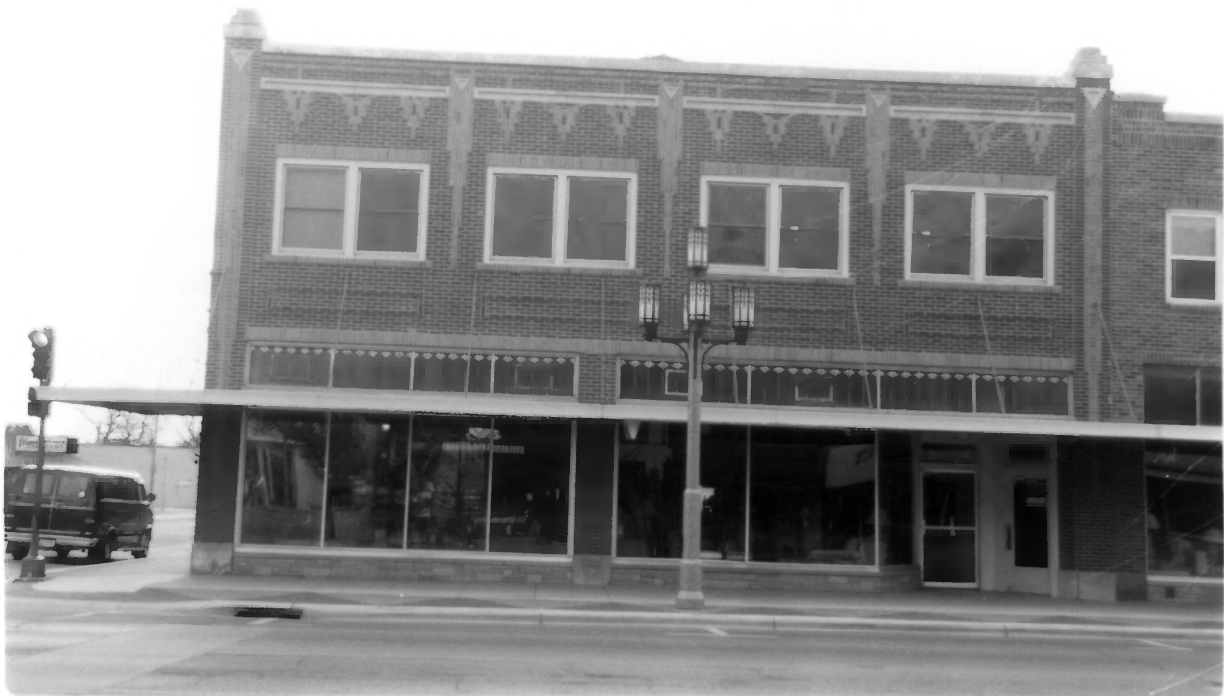
420 Grand Av Hist Commercial Dist Clay County, IA PHOTO # 20
