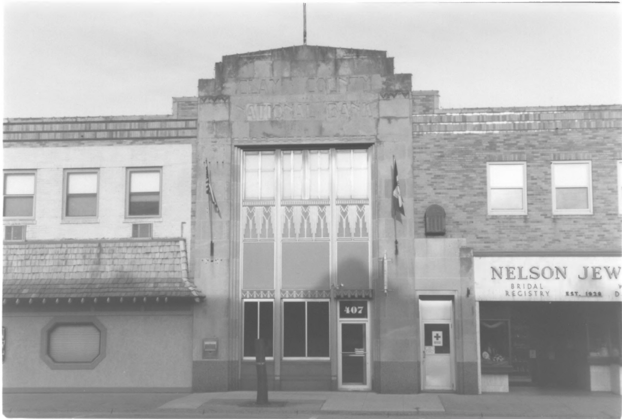
407 Grand Av Hist Commercial Dist Clay County, IA PHOTO # 12
