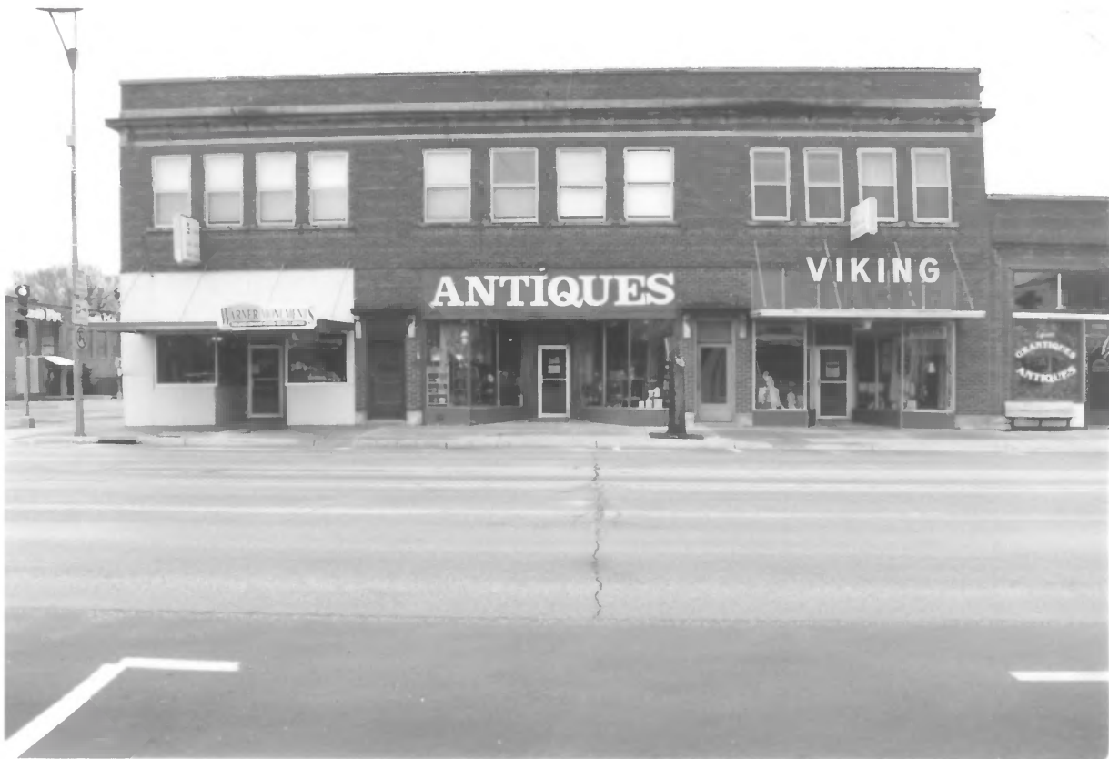
301-305 Grand Av Hist Commercial Dist Clay County, IA PHOTO #3
