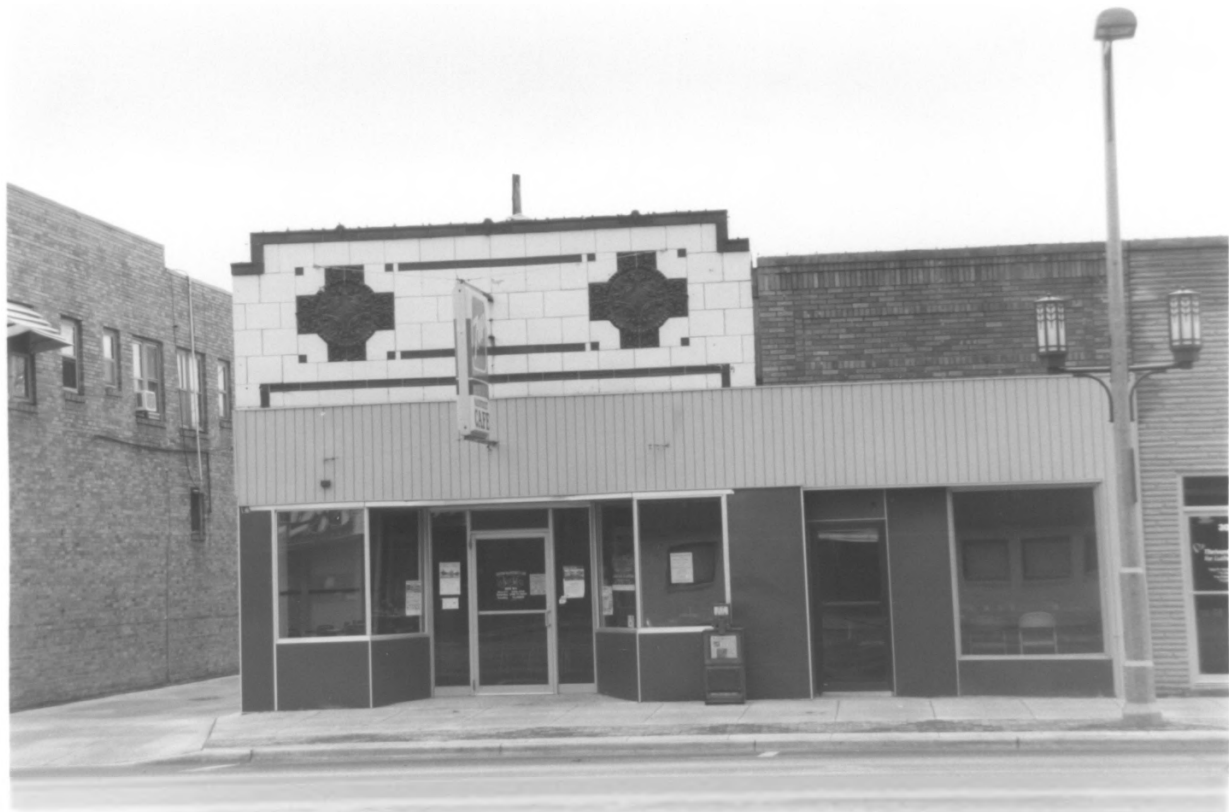
312 Grand Av Hist Commercial Dist Clay County, IA PHOTO # 7
