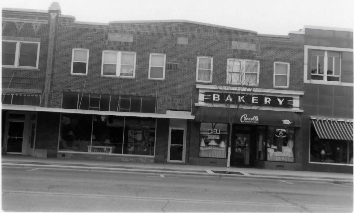
416-418 Grand Av Hist Commercial Dist Clay County, IA PHOTO #19
