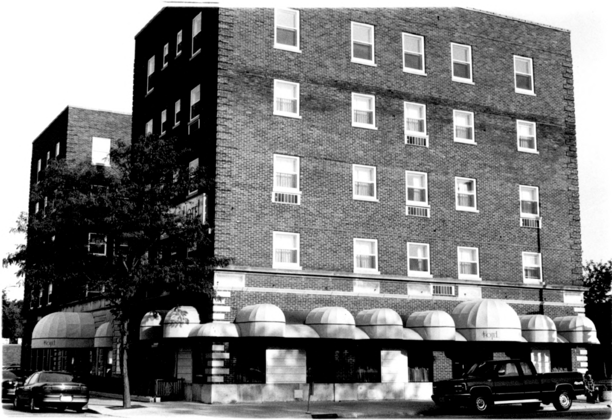
605 Grand Av Hist Commercial Dist Clay County, IA PHOTO #32
