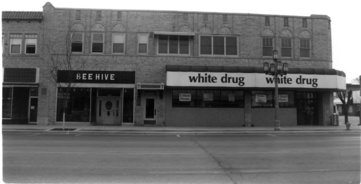
400-404 Grand Av Hist Commercial Dist Clay County, IA PHOTO #16
