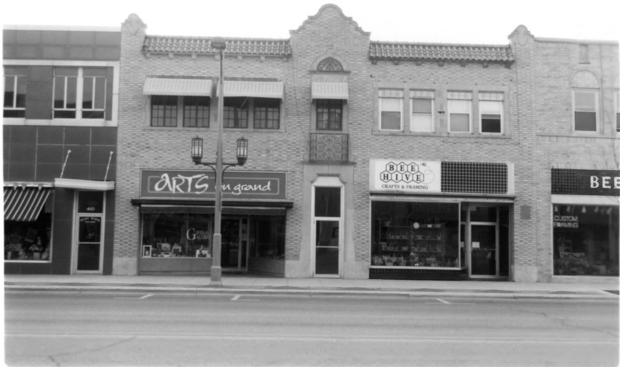
406-408 Grand Av Hist Commercial Dist Clay County, IA PHOTO # 17
