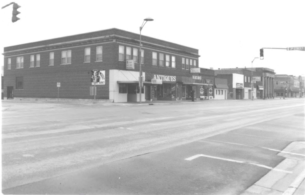
West Side 300 Blk Grand Ave Hist Commercial Dist Clay County, IA PHOTO # 1
