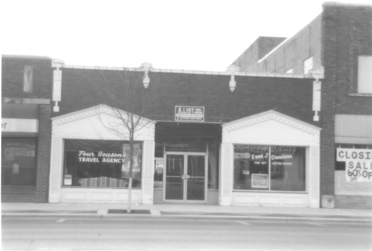
510 Grand Av Hist Commercial Dist Clay County, IA PHOTO # 30
