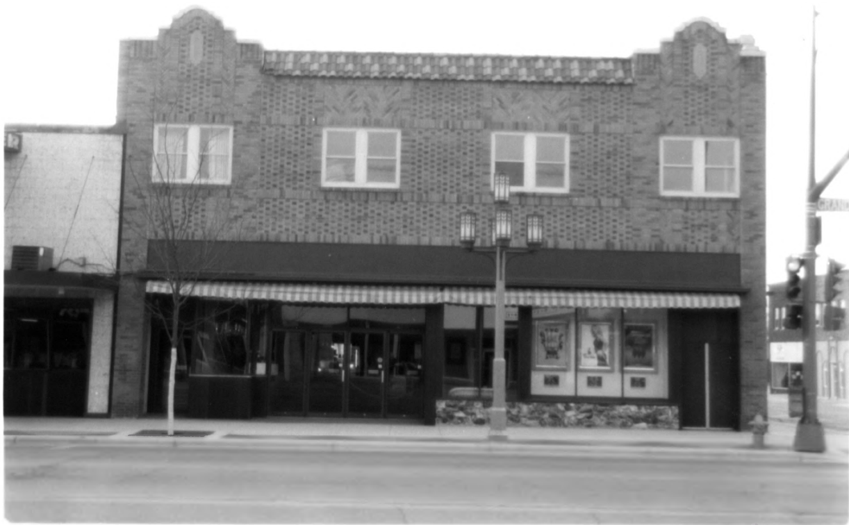
500 Grand Av Hist Commercial Dist Clay County, IA PHOTO #29
