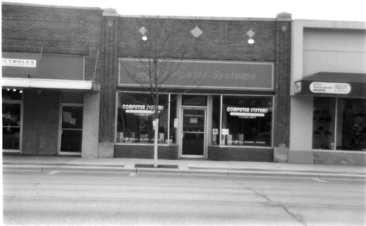
520 Grand Av Hist Commercial Dist Clay County, IA PHOTO #31
