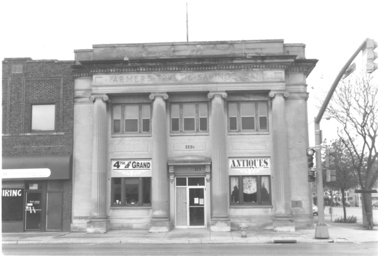
323 Grand Av Hist Commercial Dist Clay County, IA PHOTO #4
