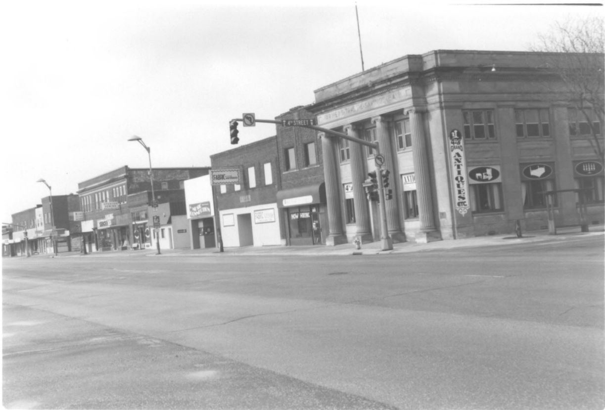
West Side 300 Blk Grand Ad Nist Commercial Dist Clay County, IA PHOTO #2
