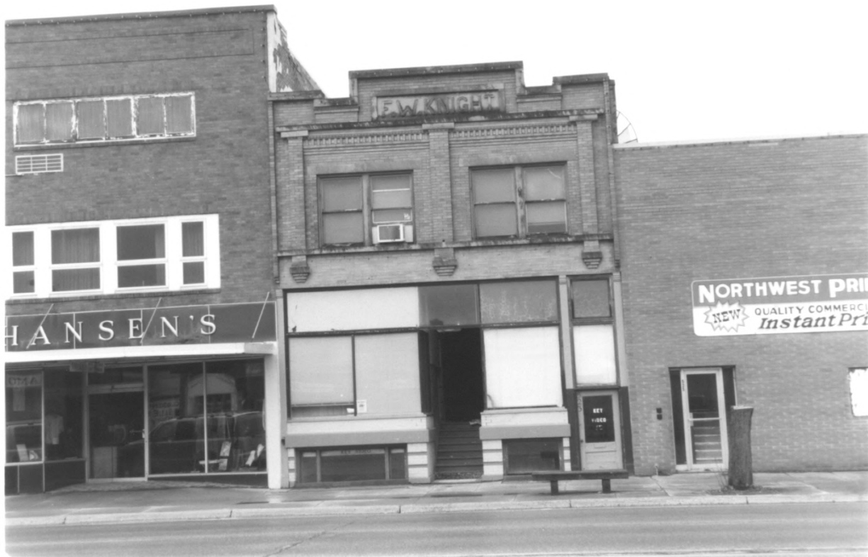
521 Grand Av Hist Commercial Dist Clay County, IA PHOTO # 26
