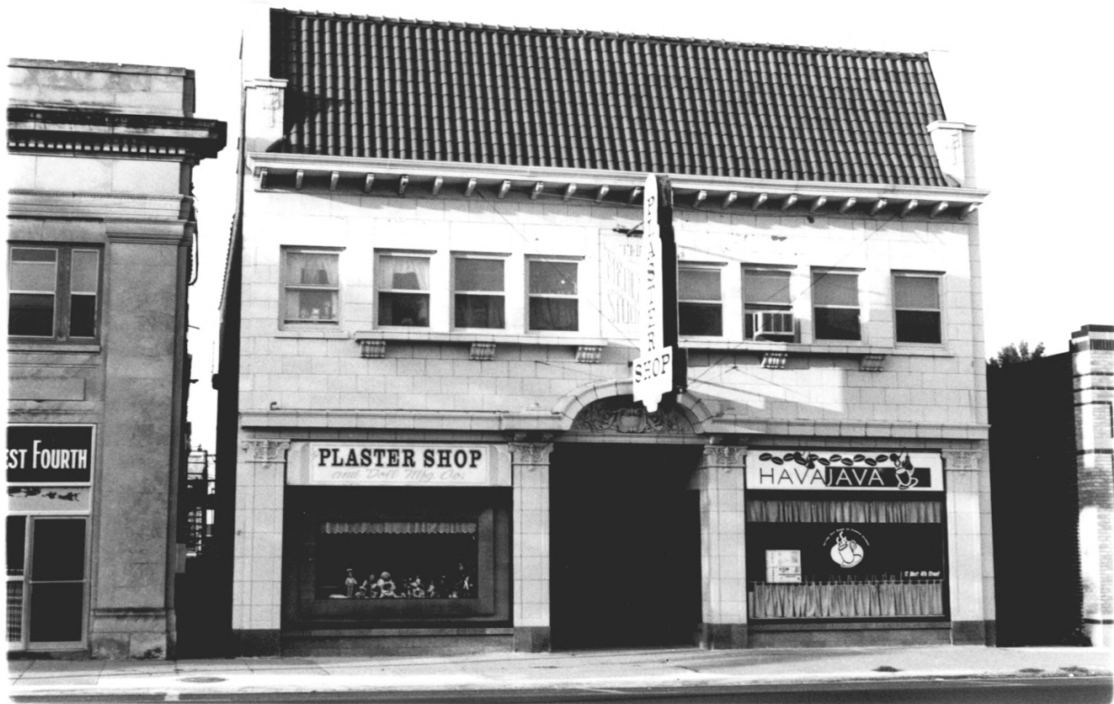
10 W. 4th St, Grand Av Hist Commercial Dist Clay County, IA PHOTO # 8
