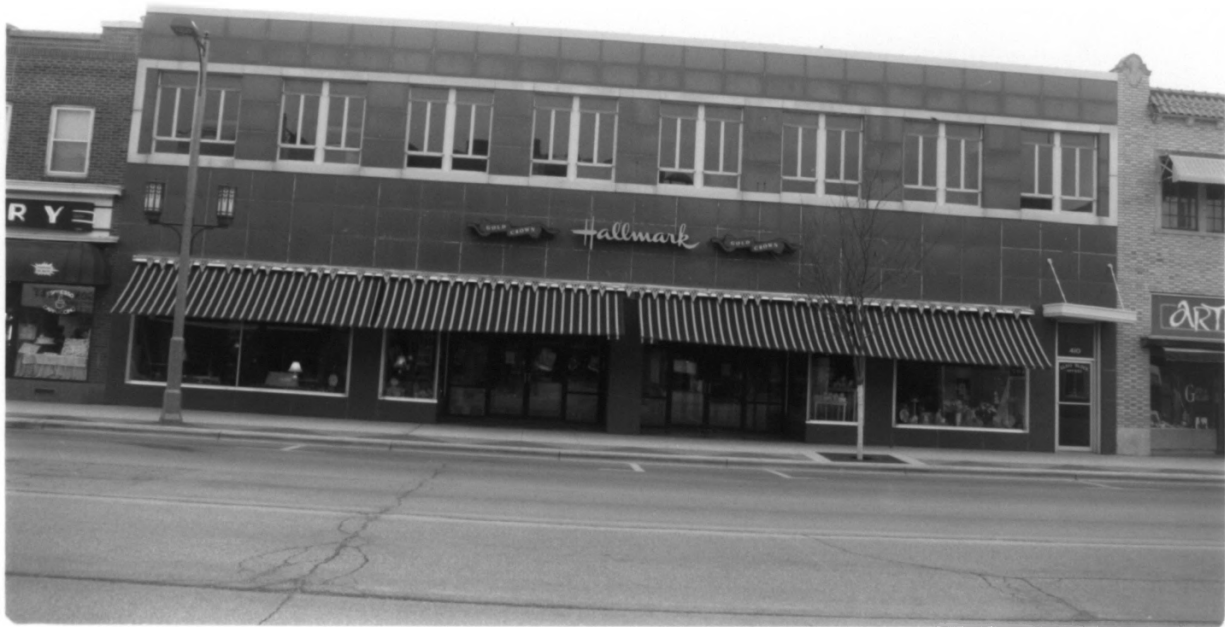
410 Grand Av Hist Commercial Dist Clay County, IA PHOTO #18
