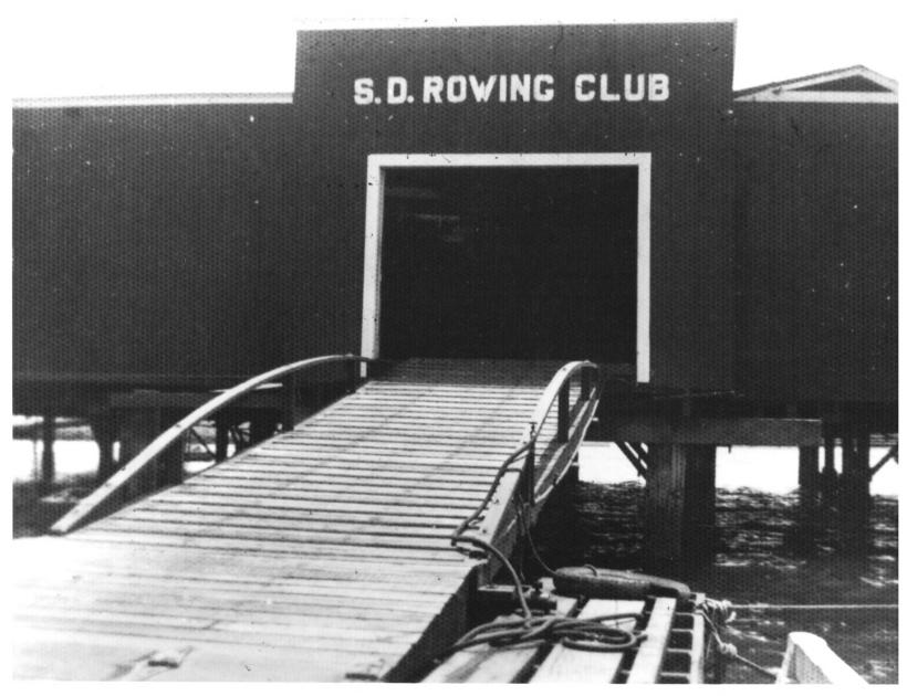
This photo (dated July 12, 1936) shows the 8' extension built in 1932 to accommodate the first 8-cared shells bought by the 6/u.b.
