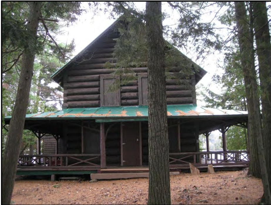
Figure 2: Façade (west elevation) of Dollar Island Camp, 2016.
