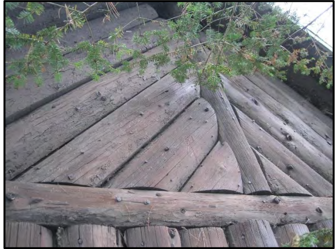
Figure 17: Shed gable end, with decorative pattern, 2016.
