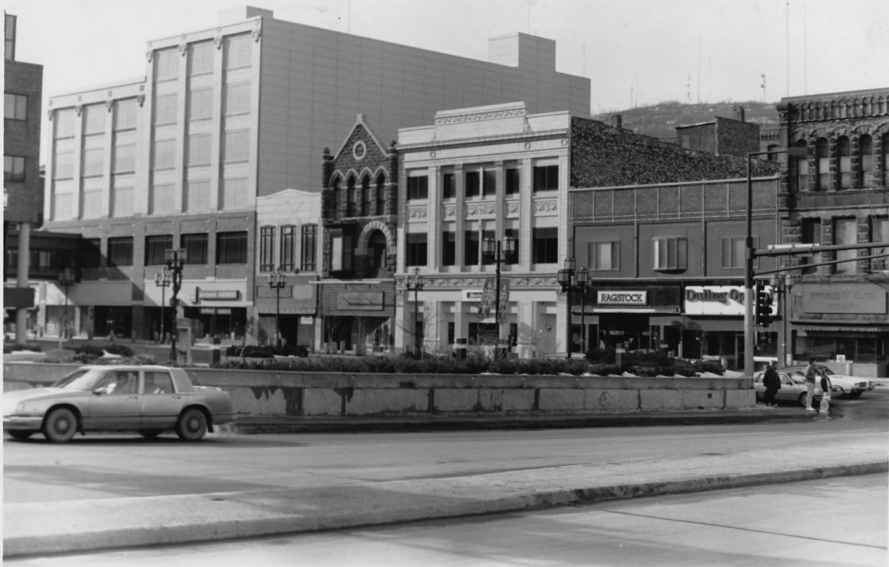
WIRTH BUILDING ST-LOUIS CO., MINNESOTA
