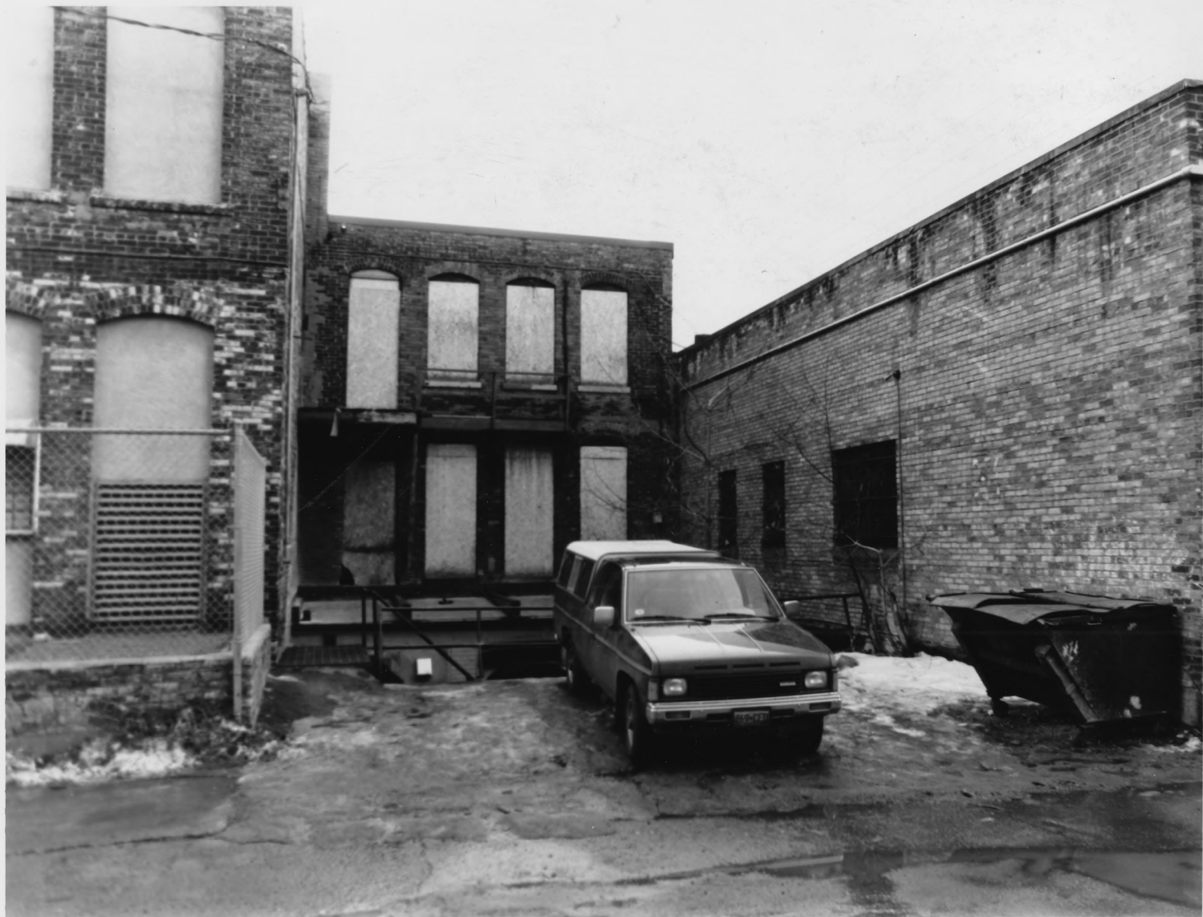
WIRTH BUILDING ST. LOUIS CO., MINNESOTA
