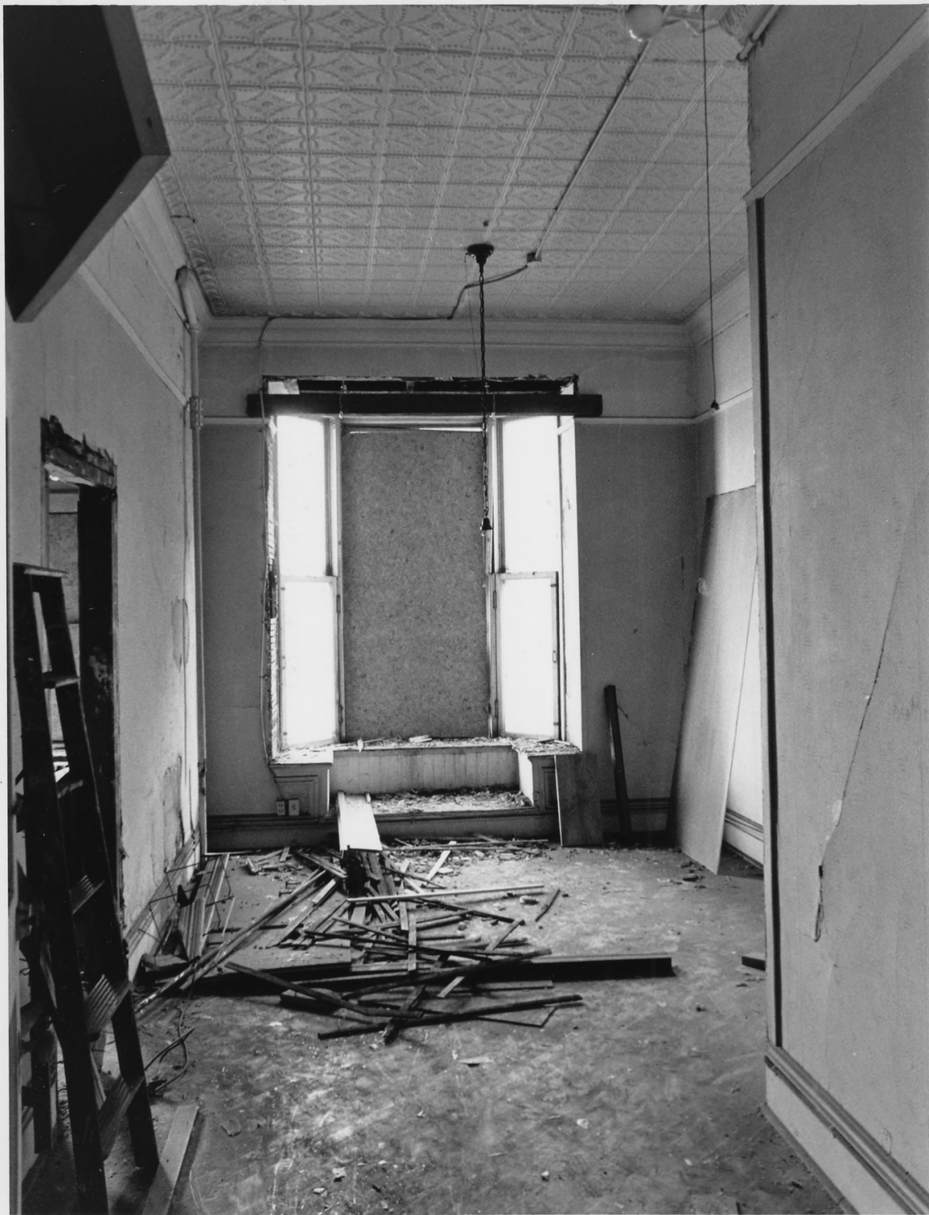
WIRTH BUILDING ST. LOUIS CO., MINNESOTA
