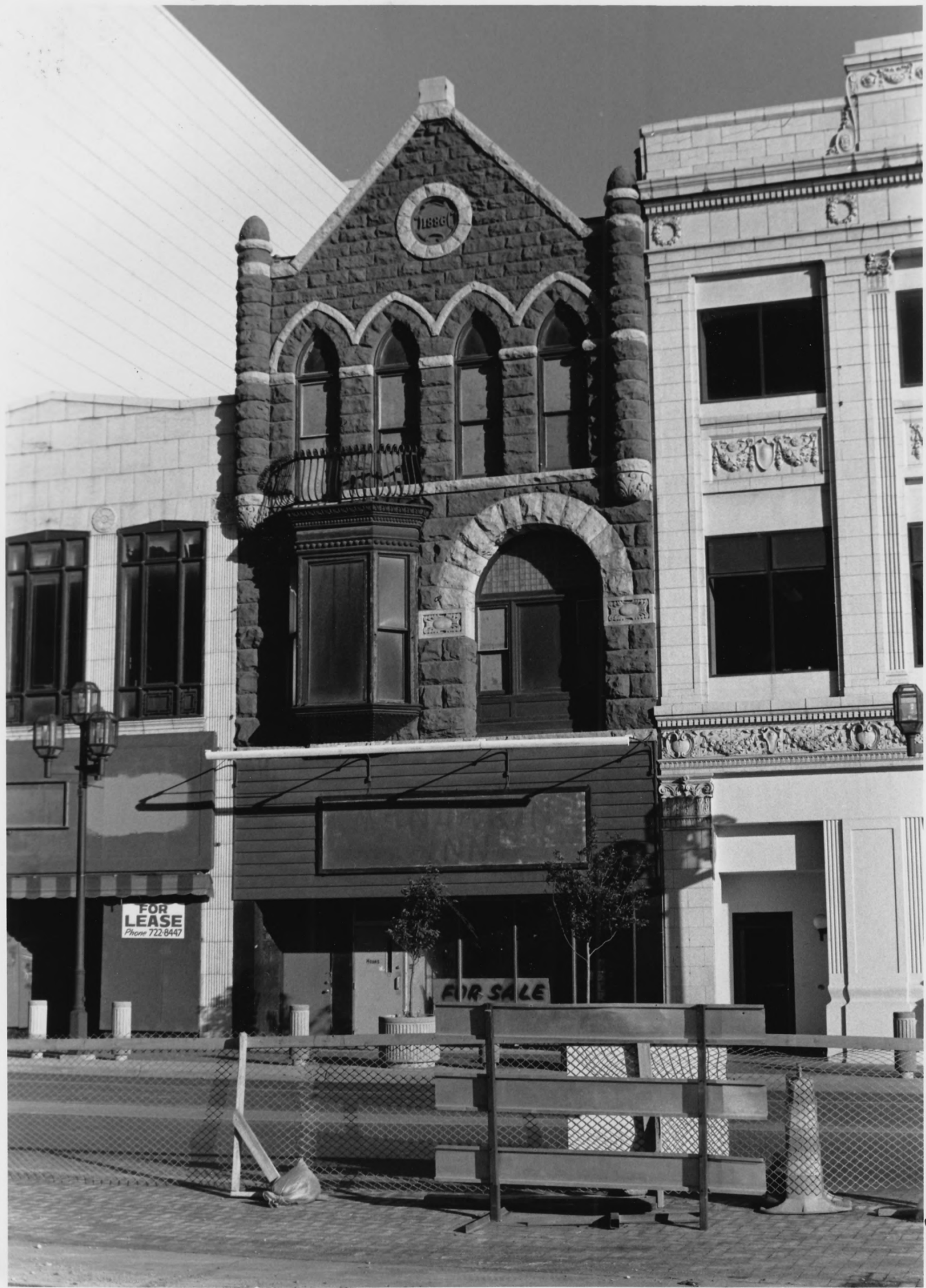
WIRTH BUILDING ST. LOUIS CO., MINNESOTA
