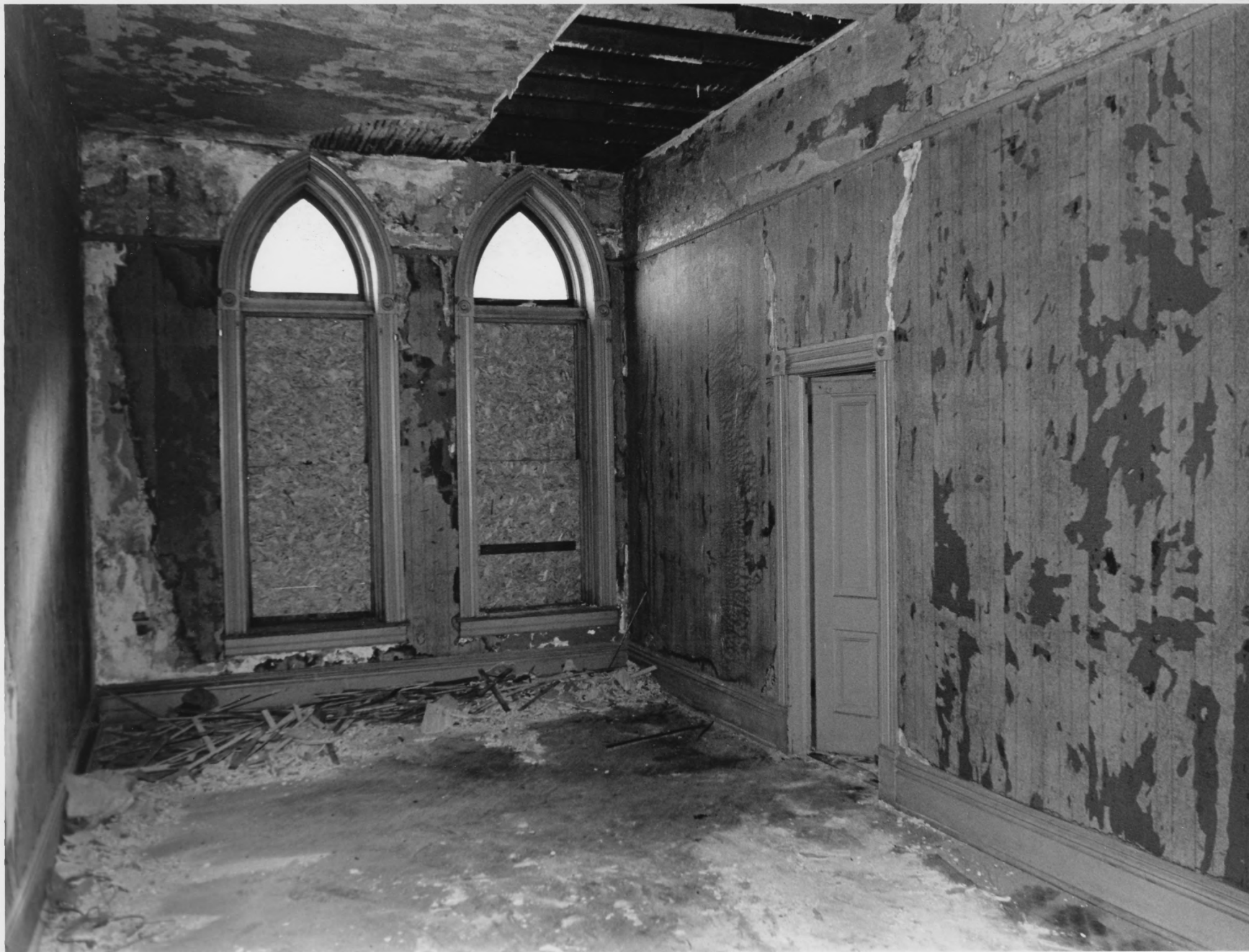
WIRTH BUILDING ST. LOUIS CO., MINNESOTA
