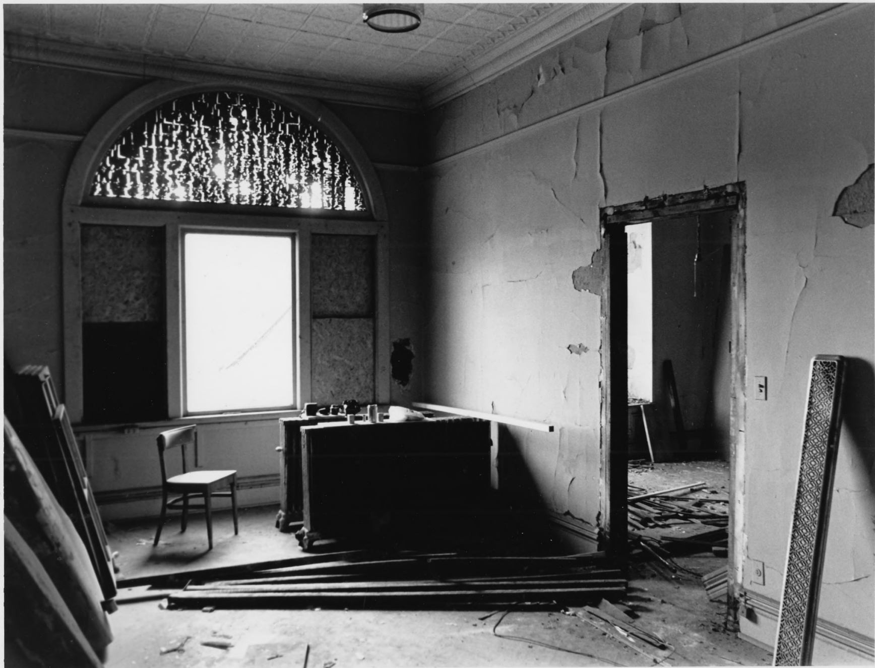
WIRTH BUILDING ST. LOUIS CO., MINNESOTA
