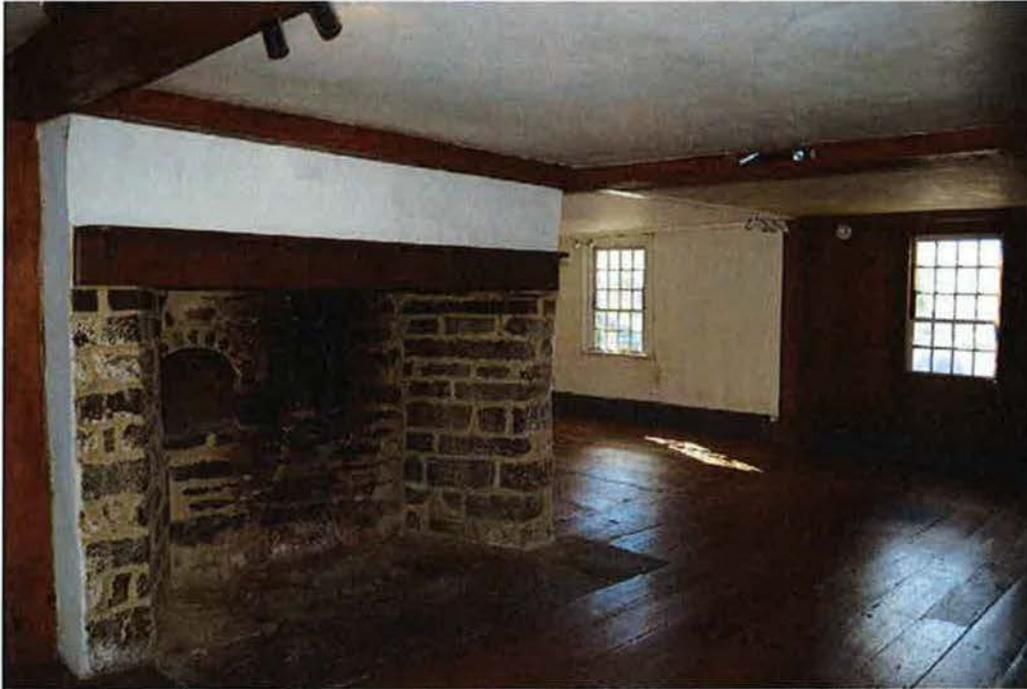
**Photo 18.** Keeping Room looking southwest towards the West Room. The fireplace with bread oven has an original hearthstone. The Keeping Room paneling is historic; the floorboards are replacement.
