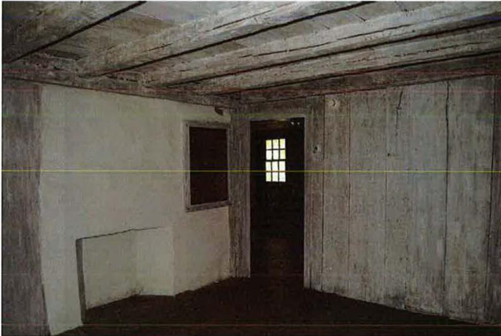
**Photo 16.** East Room looking northwest at the plaster wall with the fireplace and built-in shelving towards the doorway to the Keeping Room. The hearthstone is a replacement from the Old Ferris House on Bedford Street in Stamford.
