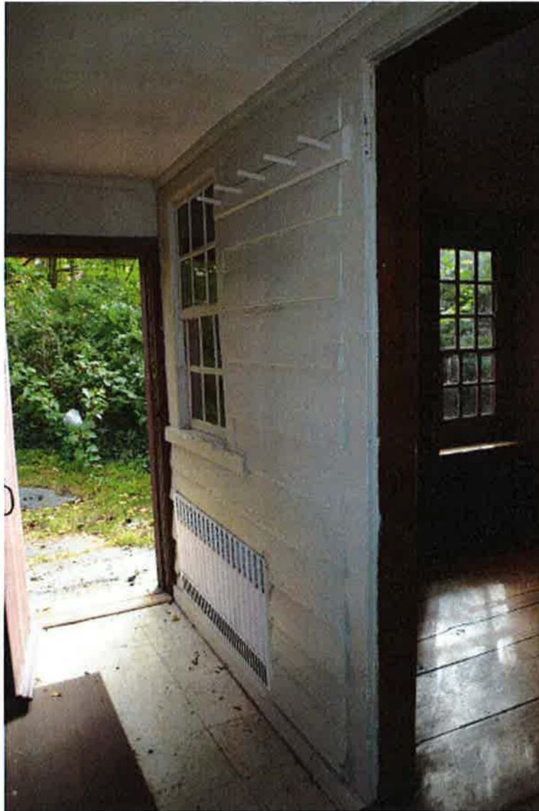
**Photo 21.** Rear ell looking east to the exterior at the east elevation and through an original exterior entrance to the Buttery. The white wall with original clapboards and window was once the original exterior north wall.
