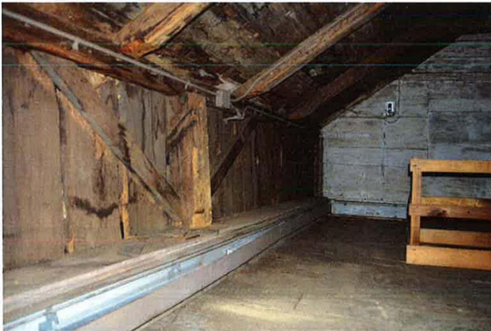
**Photo 23.** Attic looking northeast toward the access stairwell and north and east walls showing exposed roof framing and sheathing and house framing with cross-bracing framing with original sheathing along the north wall. Baseboard heat is also visible along the north wall.
