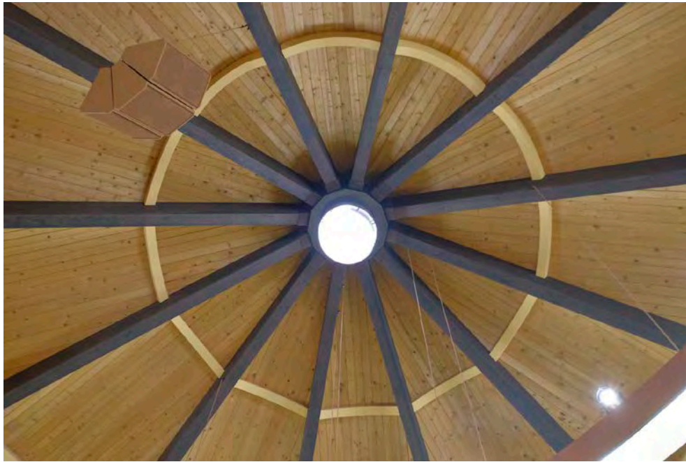
15. Interior, sanctuary, detail of arches, compression ring, and skylight.
