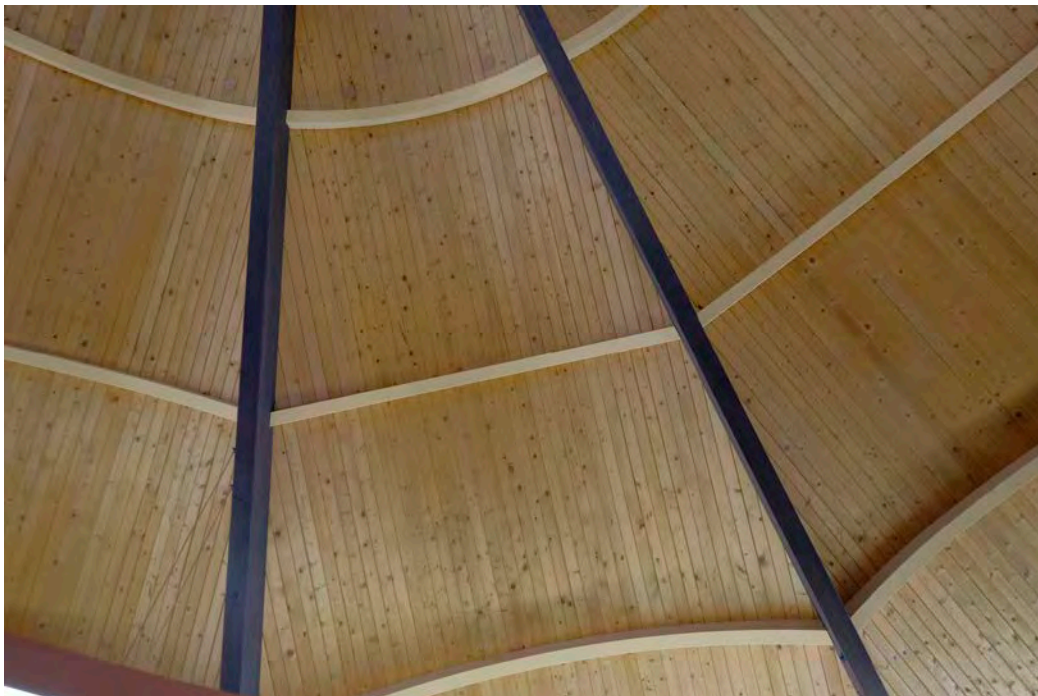
14. Interior, sanctuary, detail of wood vaults and laminated arches and purlins.
