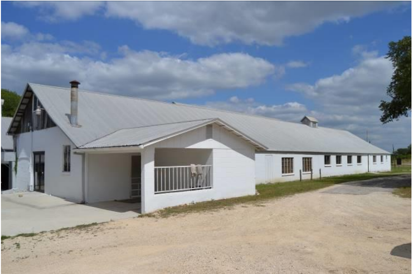
Photo No. 11. Oblique view of side west façade of Anhalt Hall, view facing southeast.
