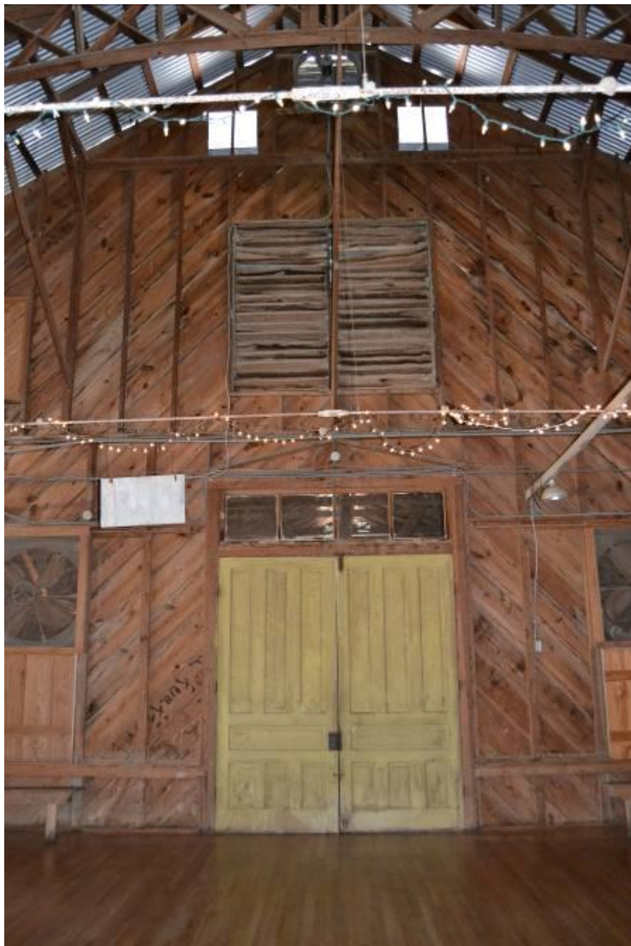
Photo No. 20. View of north wall separating dance hall and bar area inside Anhalt Hall, view facing north.
