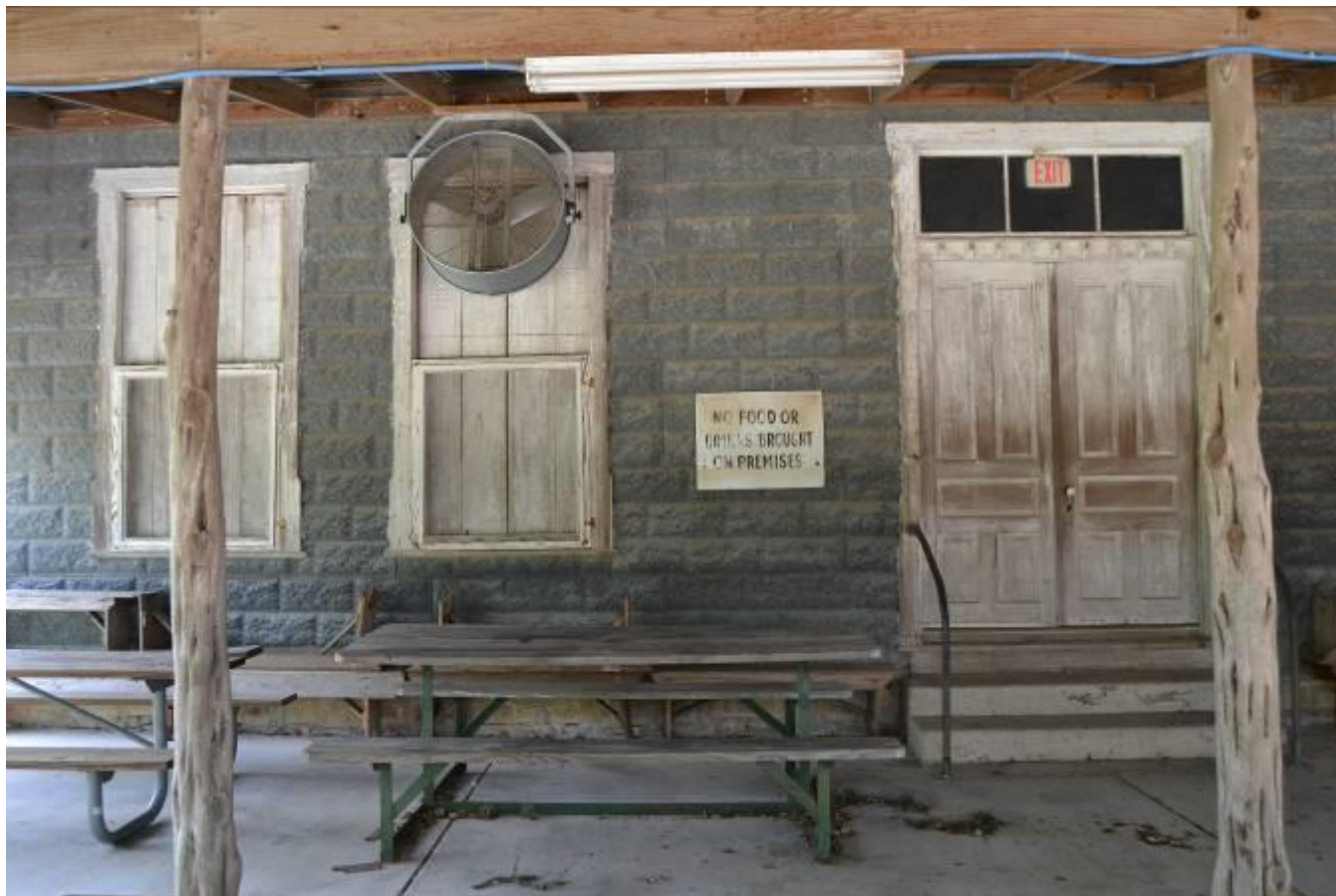
Photo No. 9. Detailed view side east façade of Anhalt Hall, view facing west.
