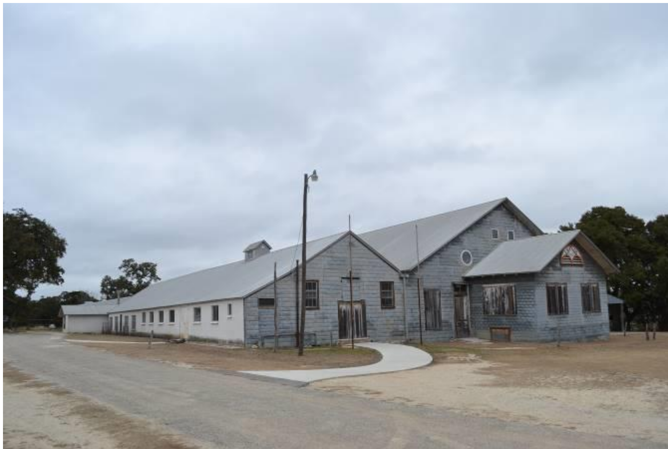
Photo No. 3. Oblique view of Anhalt Hall, view facing northeast.
