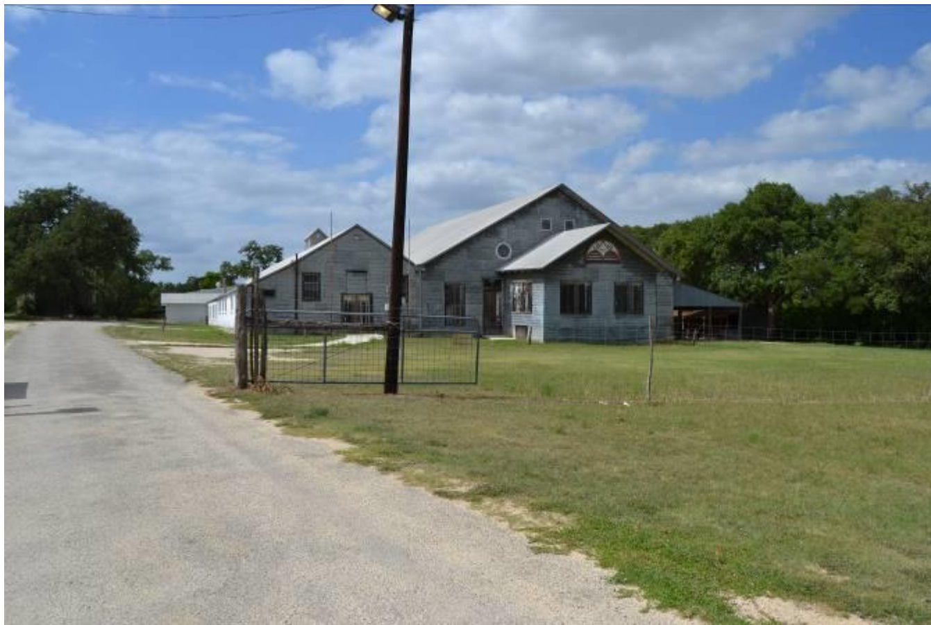
Photo No. 2. Contextual view of drive coming in from southeast and running along west side of Anhalt Hall, view facing northeast.
