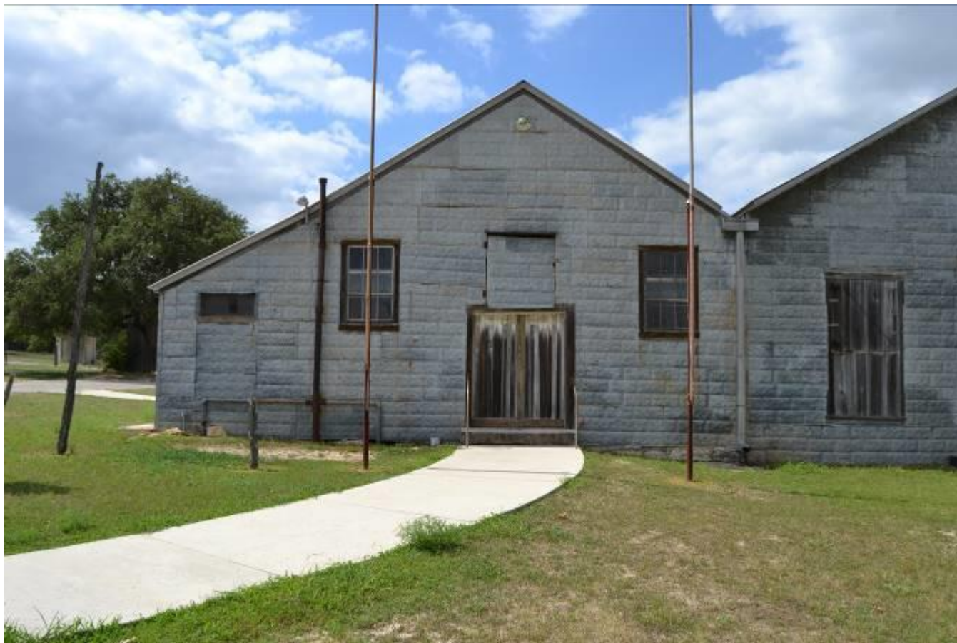
Photo No. 6. View of western half of main south façade of Anhalt Hall, view facing north.
