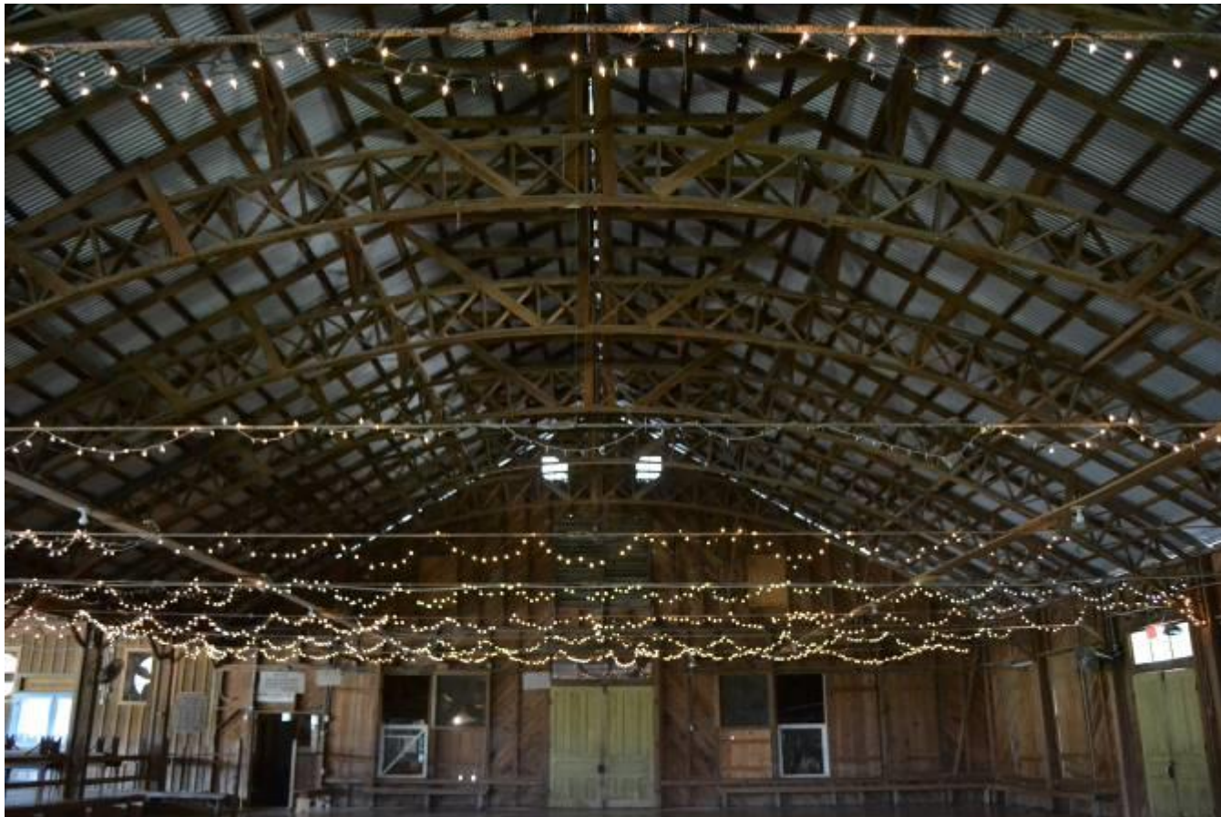
Photo No. 25. View of arched trusses in dance hall inside Anhalt Hall, view facing north.
