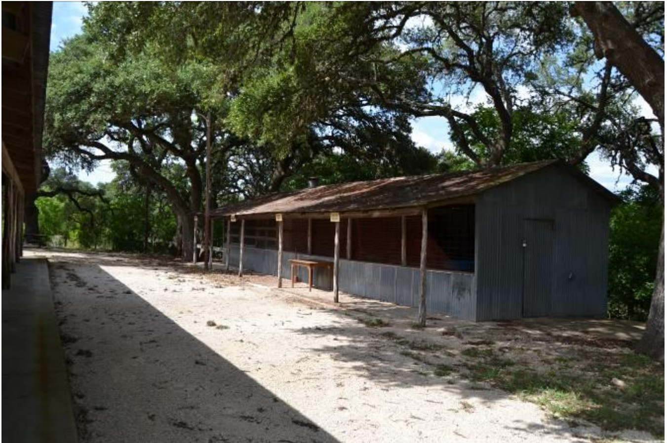
Photo No. 31. View of bar stand (Resource e), view facing northeast.
