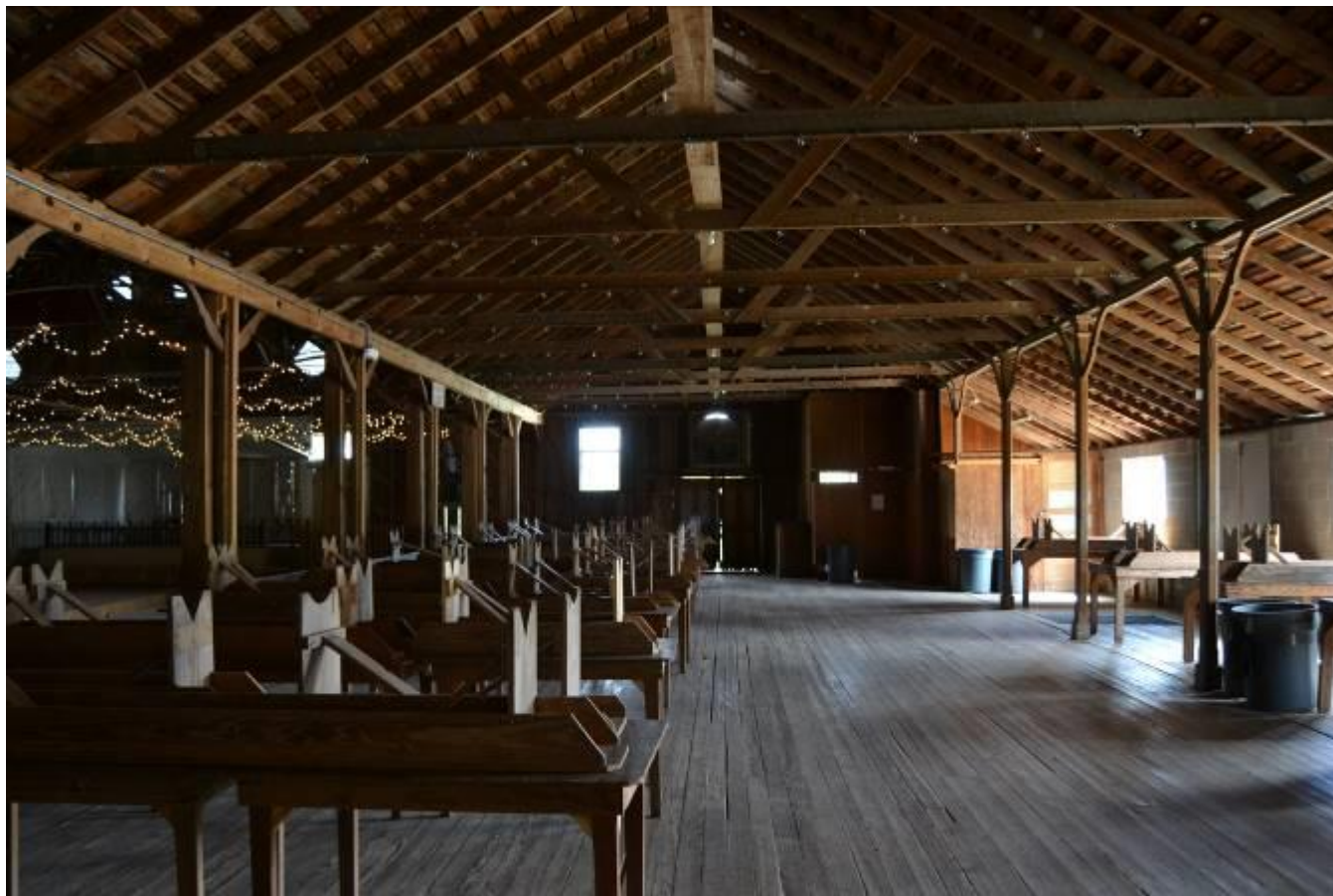
Photo No. 13. View of seating area inside Anhalt Hall, view facing south.
