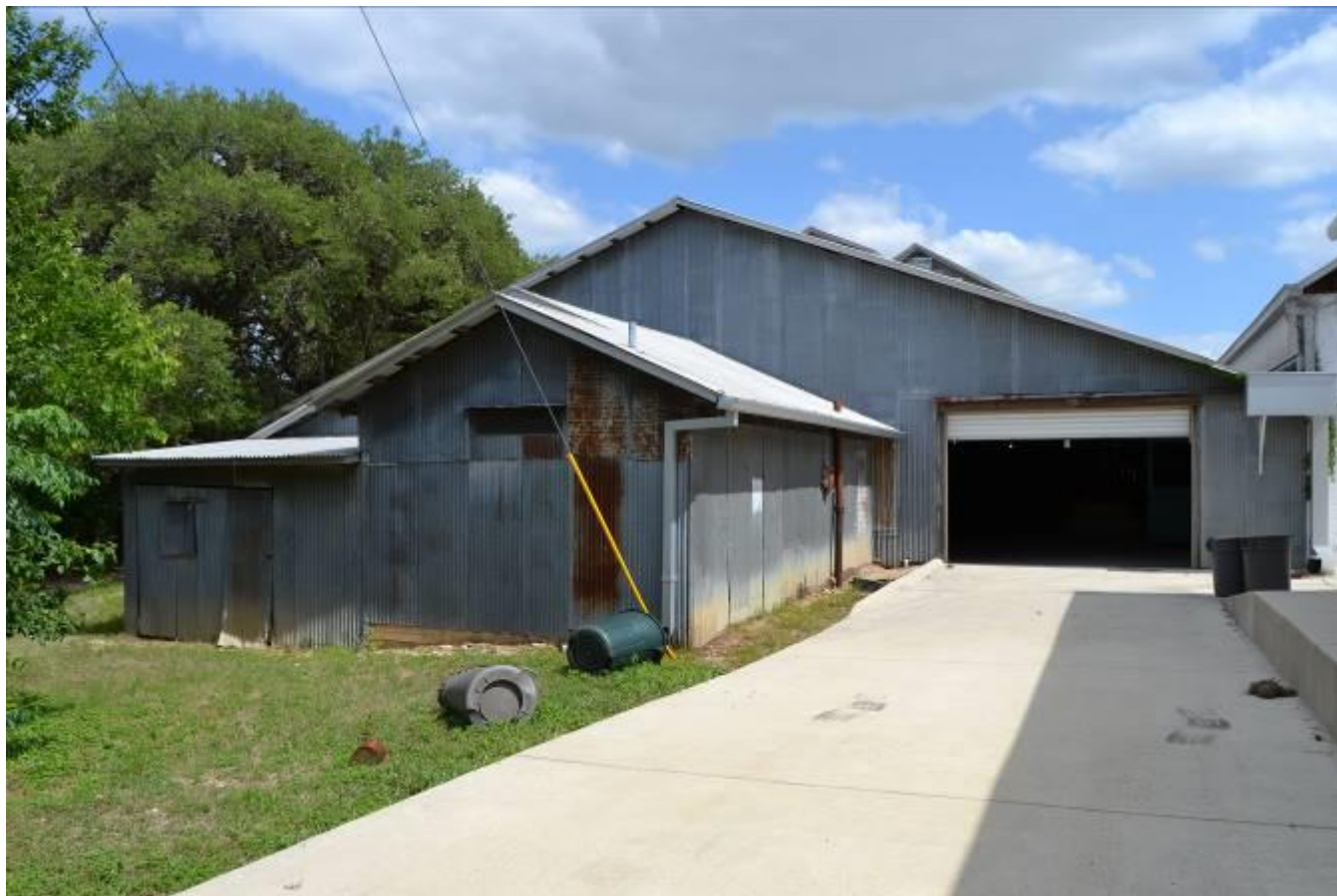
Photo No. 12. View of eastern half of rear façade of Anhalt Hall, view facing south.
