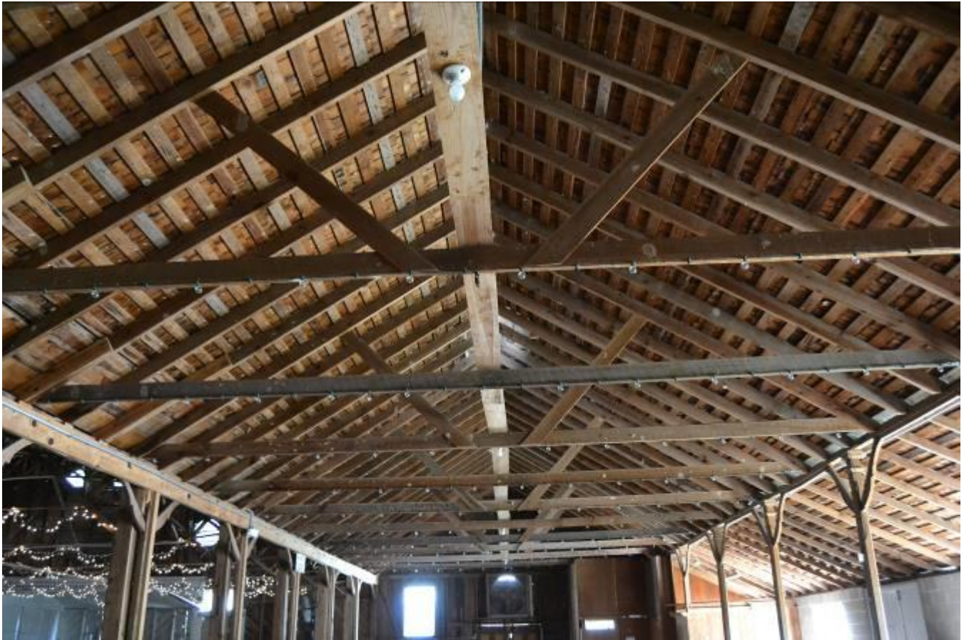
Photo No. 21. Detailed view of roof trusses in seating area inside Anhalt Hall, view facing south.
