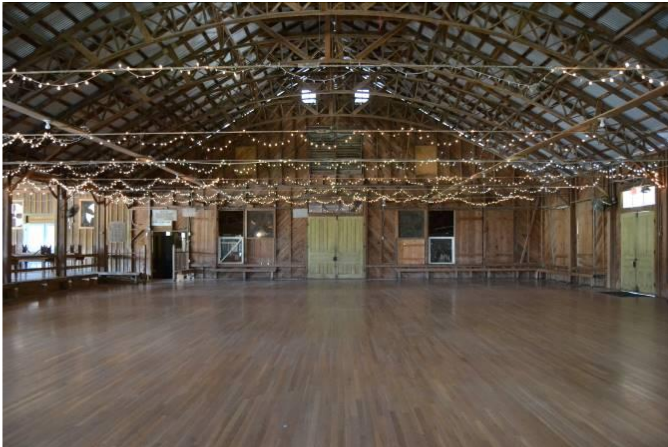
Photo No. 14. View inside dance hall at Anhalt Hall, view facing north.
