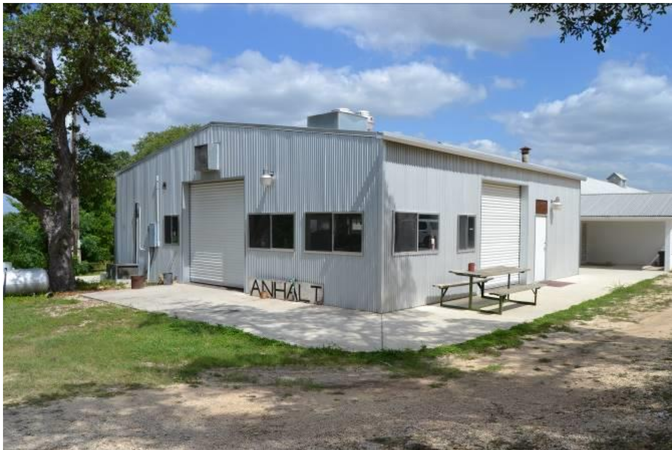
Photo No. 33. View of kitchen building (Resource b), view facing southeast.
