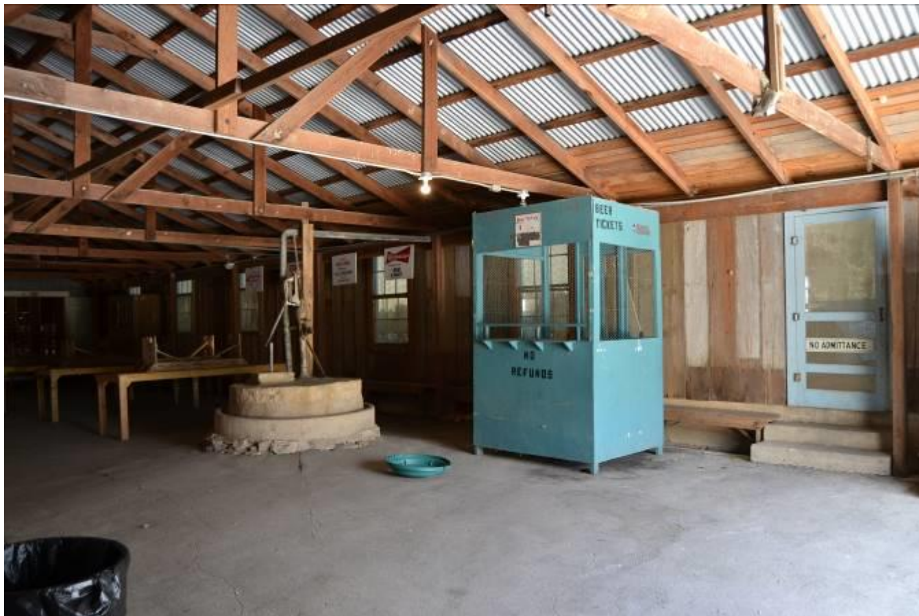
Photo No. 28. View of cistern in bar area inside Anhalt Hall, view facing southwest.
