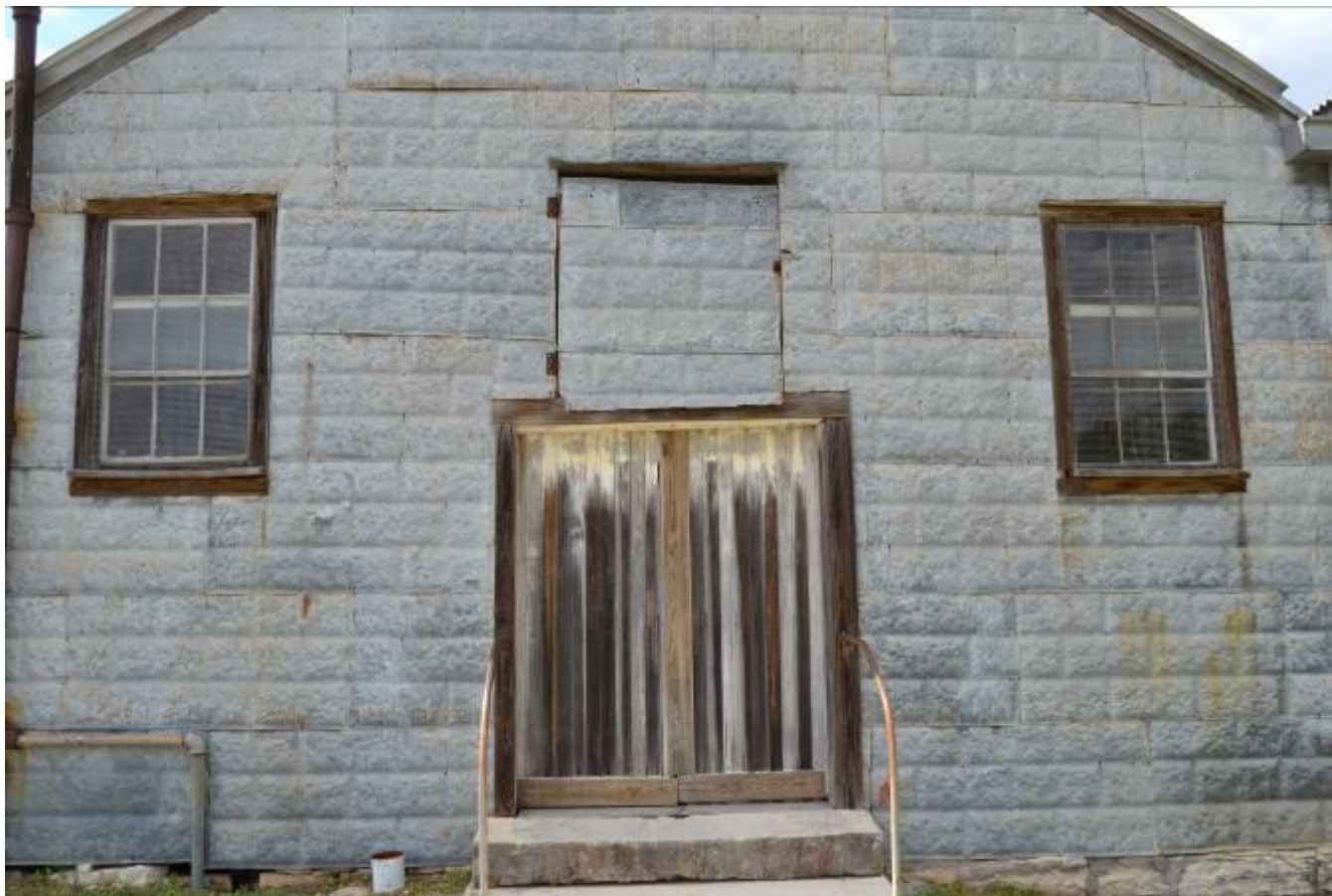
Photo No. 4. Detailed view of pressed metal sheets on main south façade of Anhalt Hall, view facing north.
