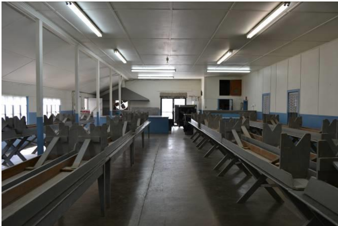
Photo No. 29. View of kitchen and dining area inside Anhalt Hall, view facing north.
