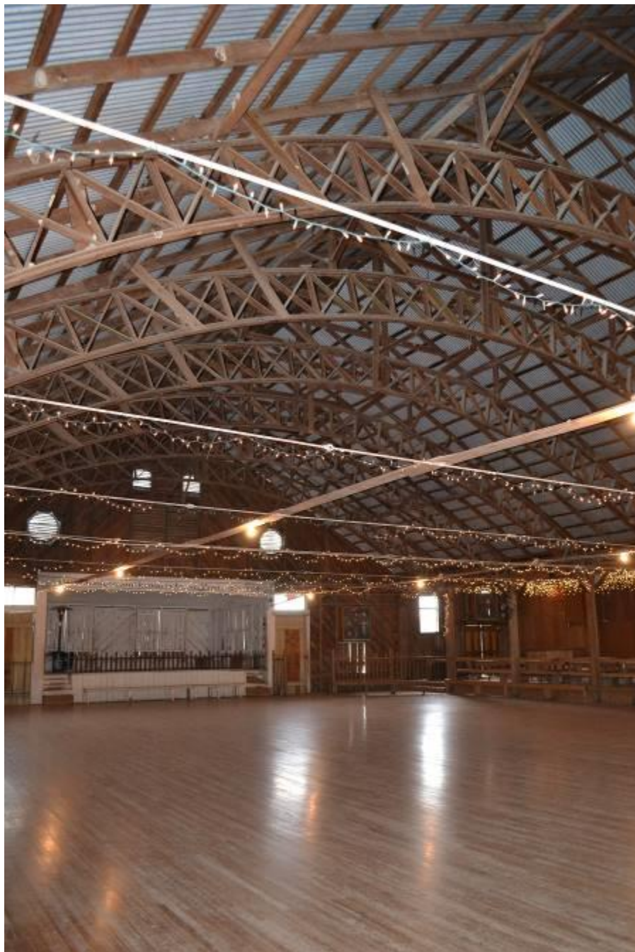
Photo No. 24. View of arched trusses in dance hall inside Anhalt Hall, view facing southwest.
