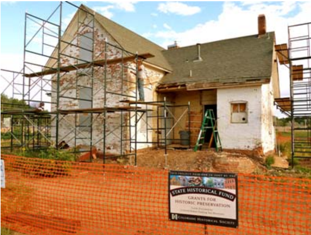
Fig. 11 2010 Southeast Façade, during restoration
