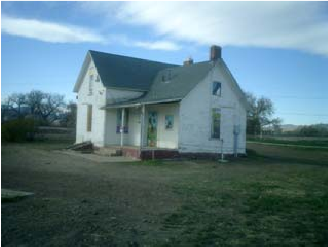
Fig. 10 2009 Northeast-facing side, prior to restoration
