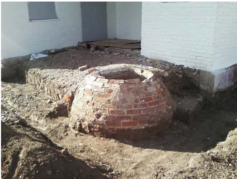
Fig. 17 2011 Cistern Uncovered (Northeast -facing side), during restoration
