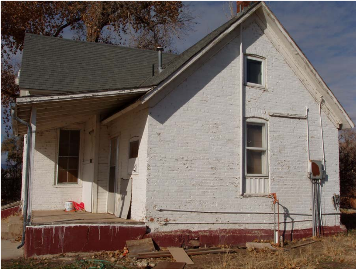
Fig. 8 2009 Northeast Façade, prior to restoration
