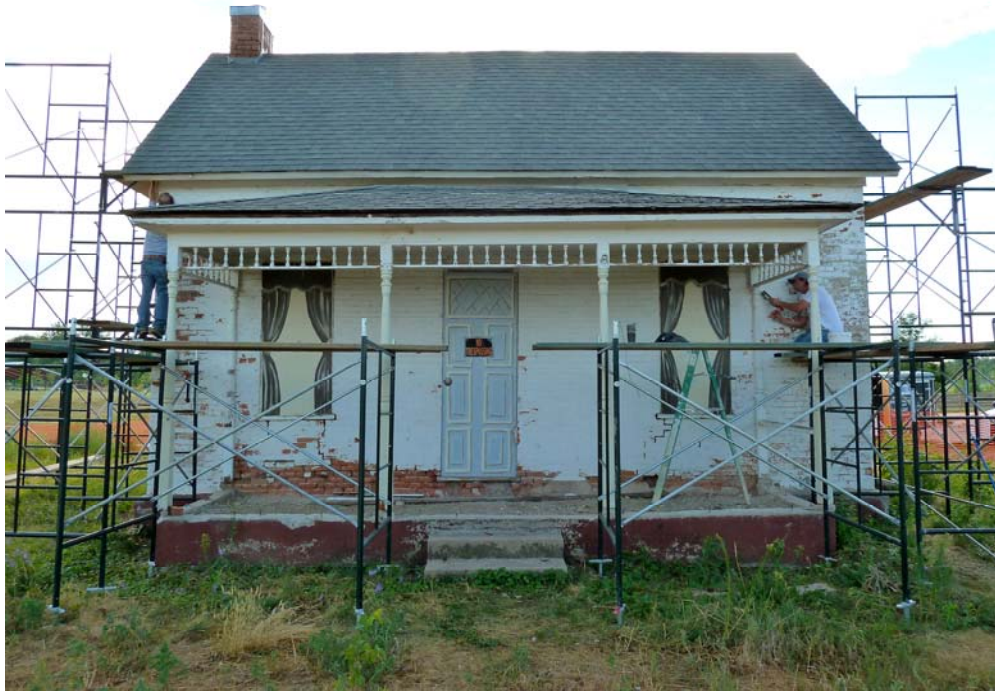
Fig. 12 2010 Southwest Façade, during restoration
