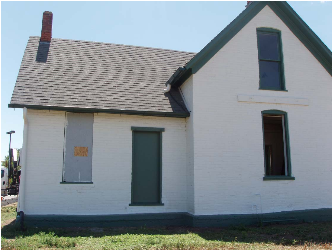
Fig. 15 2011 Northwest-facing side, during restoration
