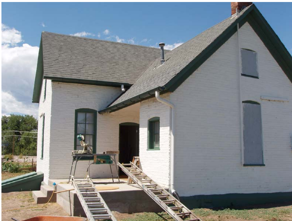
Fig. 19 2011 Northwest-facing side, during restoration
