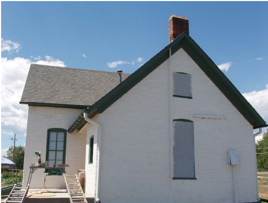
Fig. 18 2011 Northwest-facing side, during restoration
