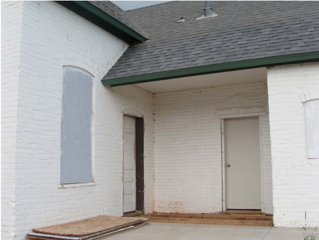
Fig. 14 2011 Southeast Porch, during restoration
