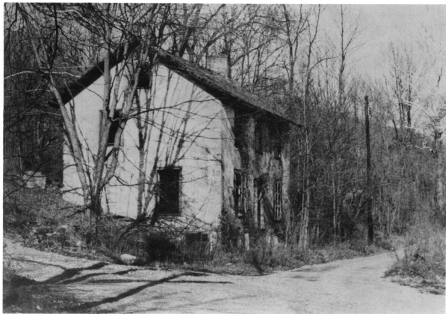
OFFICE & STORE #2 IN 1957 (V.I.R.)
