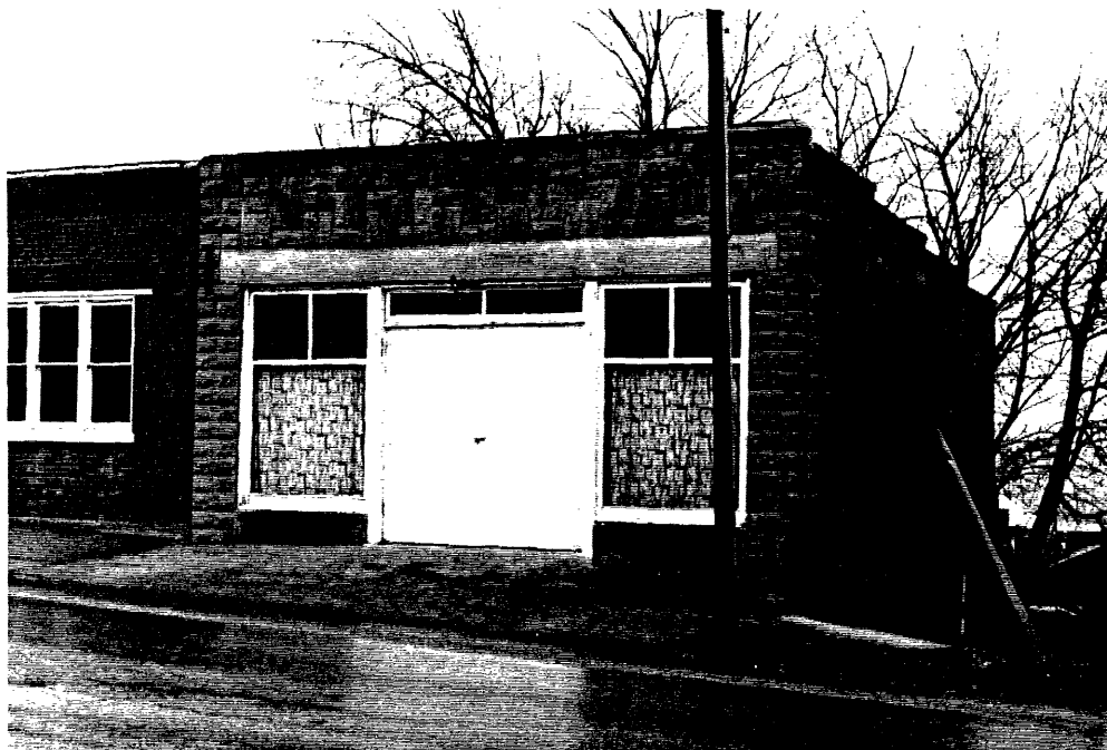
Type III Building (#28), View to the ENE.
