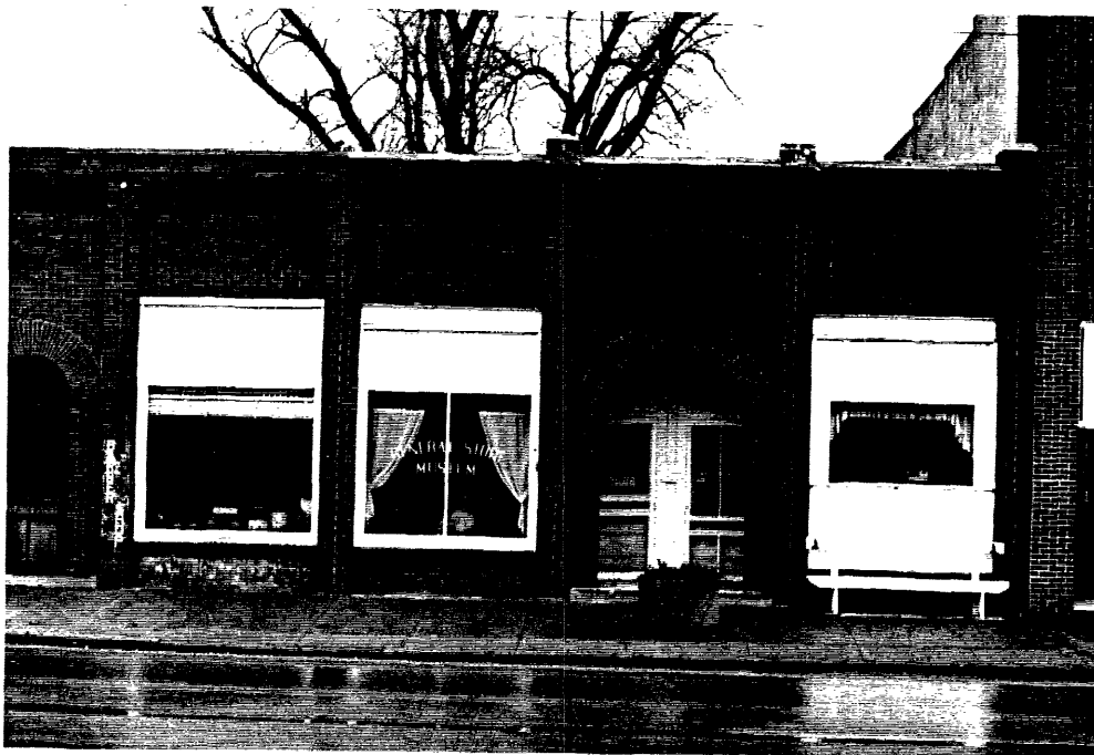
Type III Building (#24a-b), View to the East.
