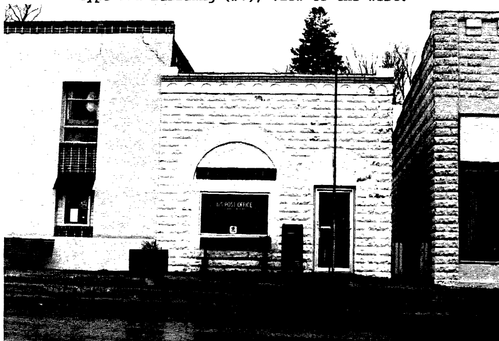
Type III Building (#2), View to the West.
