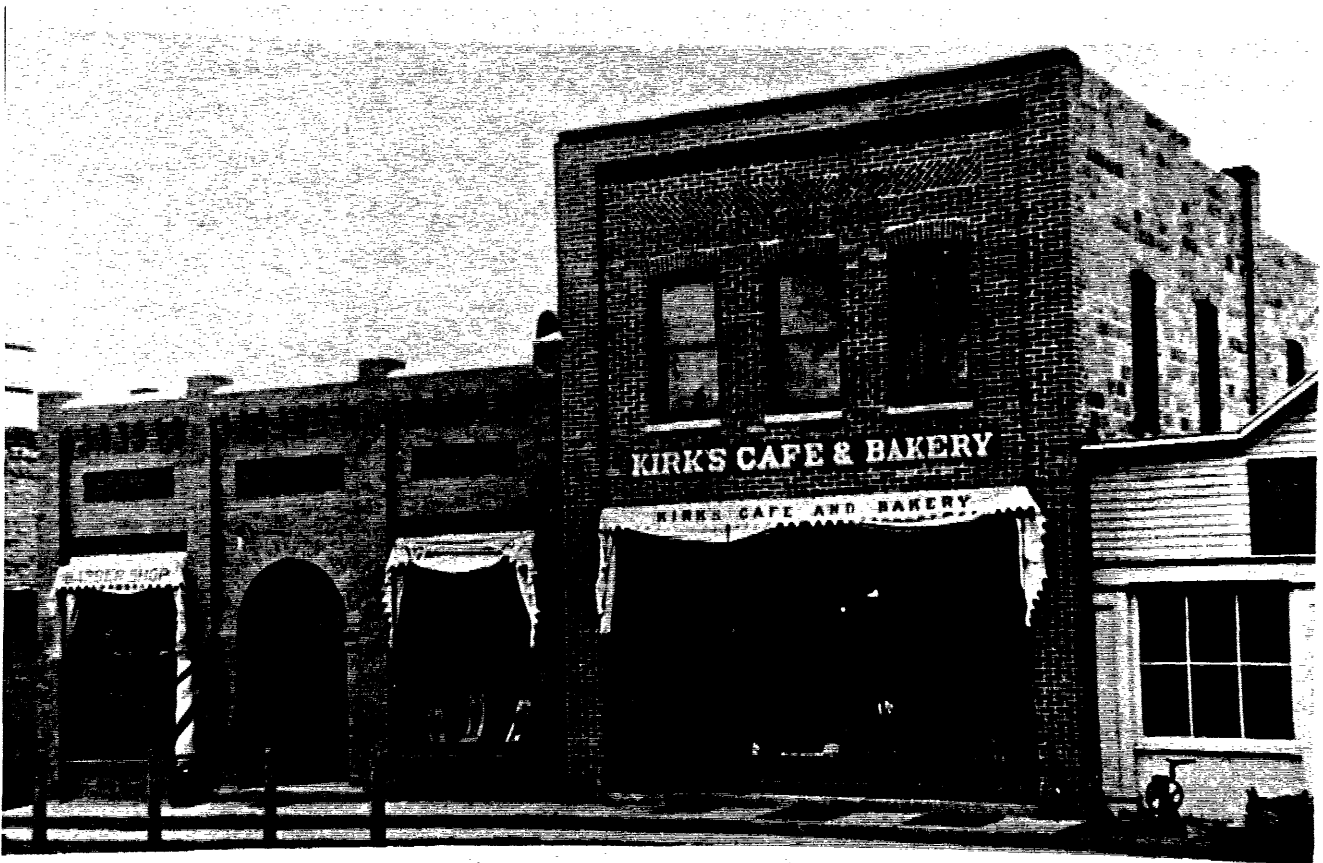
Historic Photo of Buildings 24a-b and 25, c.1913-1920, View to the NE.
