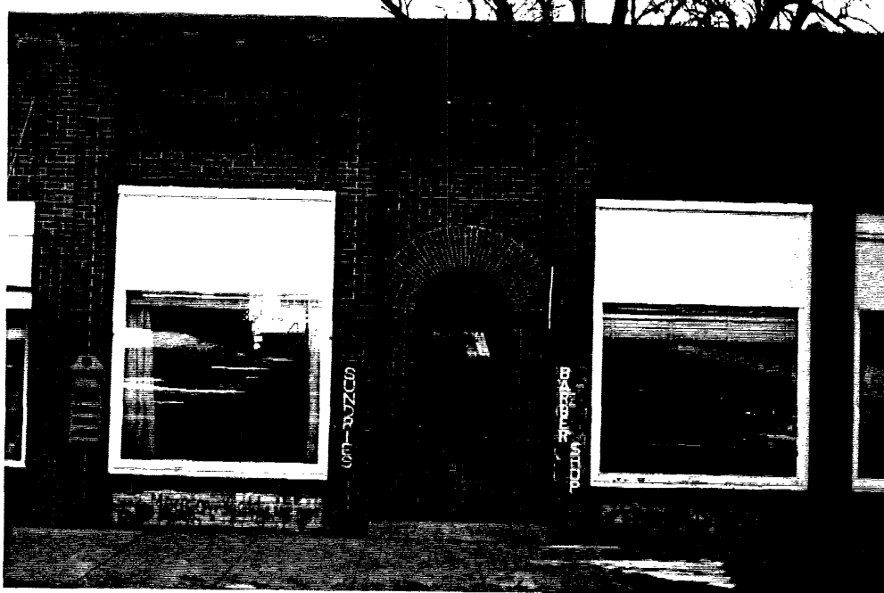
Type III Building (#23), View to the East.
