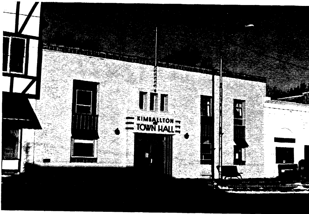
Photo 7-8. WPA Town Hall (Building 3) View to the WNW
