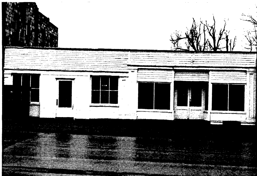
Present Configuration of Building 26a-b, View to the East.
