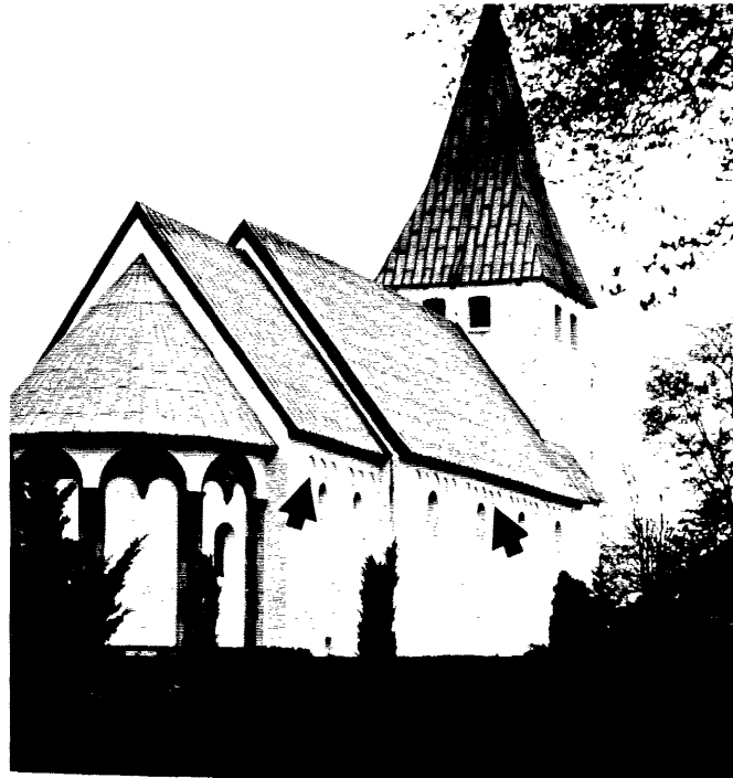
Photo 7-4. Church (upper) in Lintrup and Commercial Building (lower) in Ribe, Denmark, showing scalloped moldings and corbeling.
