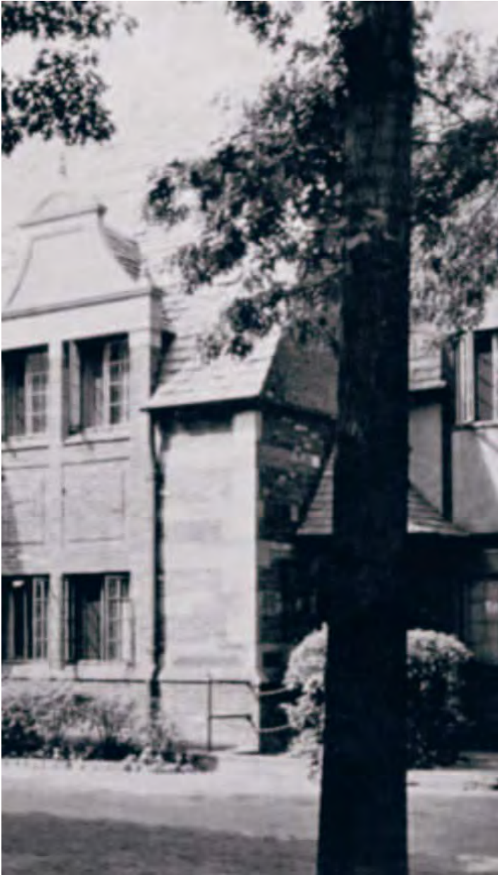
Entrance - Original Configuration
