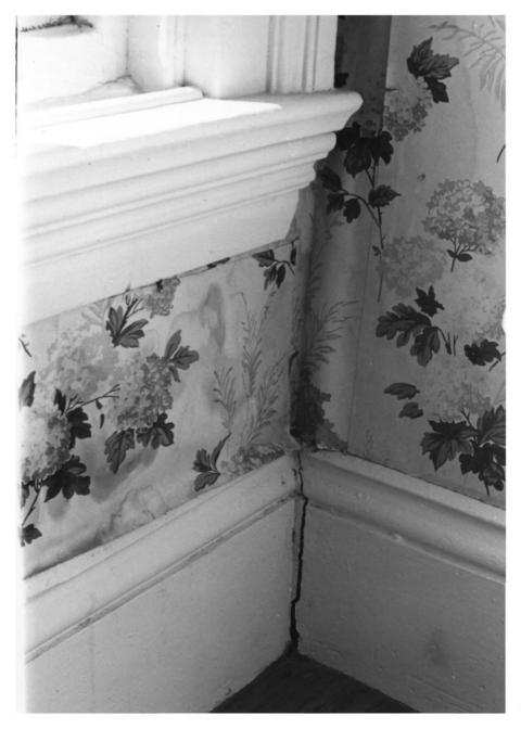
James Moore House JUL 3 1 1978 Woodland, CA Photo by A. L. Hurtado Negative at CA OHP Detail, interior window moulding and base board showing deterioration and mold. #13 NOV 1 6 1978
