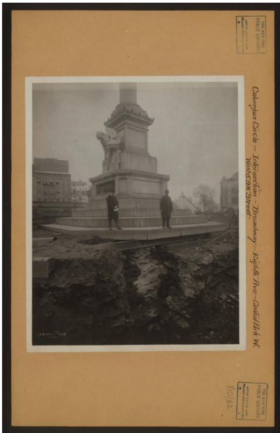
Figure 4. "Columbus Circle-Intersection-Broadway-Eighth Avenue-Central Park W. West 59th Street" Base of Columbus Monument, in the Center of Columbus Circle, at the intersection of Broadway, Eighth Ave., Central Park West and West 59th Street. Foreground shows work in progress for the I.R.T. Subway. William B. Parsons Collection.
