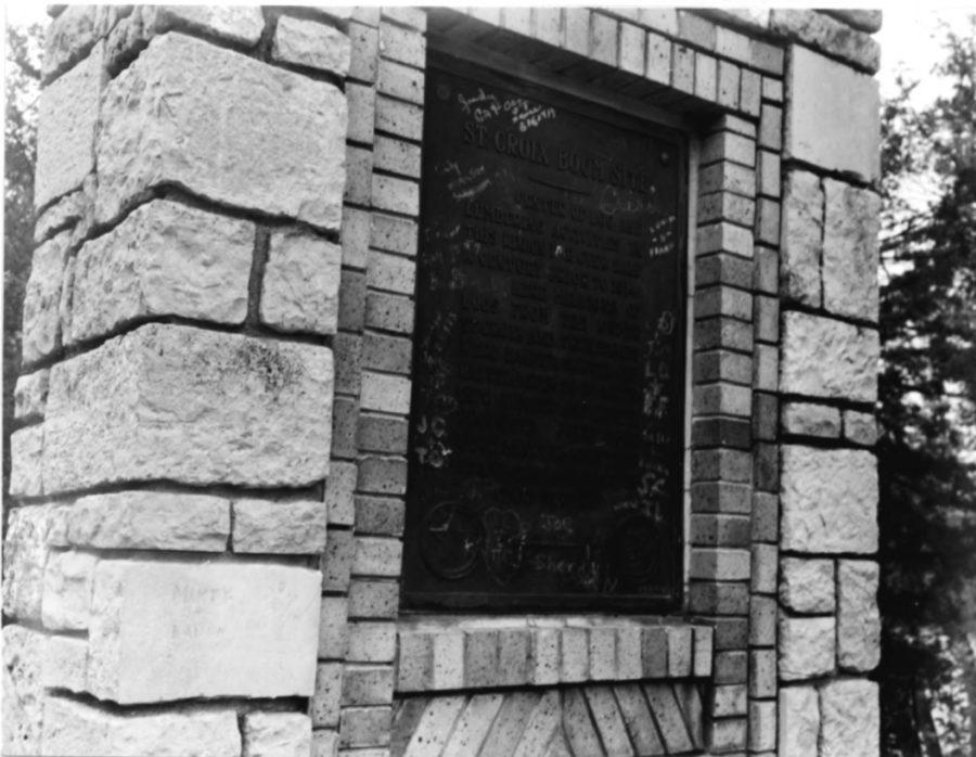
Marker located at St. Croix boom site, showing text.
