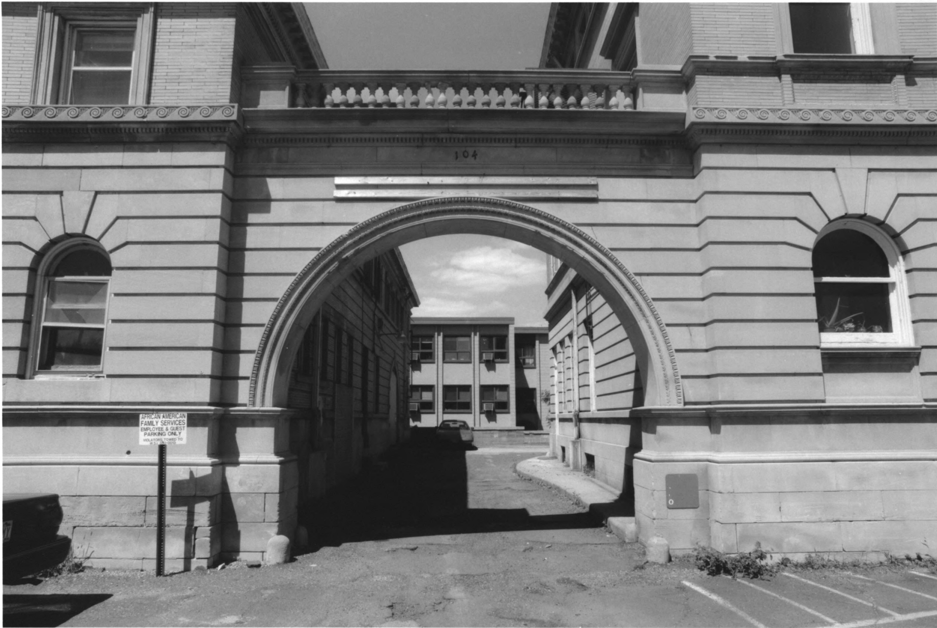
Semple, Anne C. and Frank B., House 100-104 West Franklin Ave., Minneapolis Hennepin Co., MN 013245-12/12A
