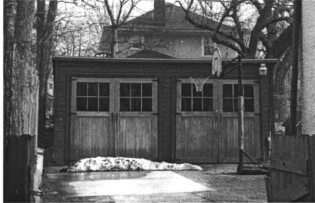
Garage, 719 33 rd Street (*) (photo by James Jacobsen, February 23, 2000)
