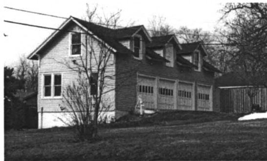
Garage, 701 31 st Street (1929) (photo by James Jacobsen, February 23, 2000)
