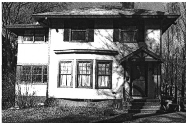
676 32nd Street, Foursquare with solarium
