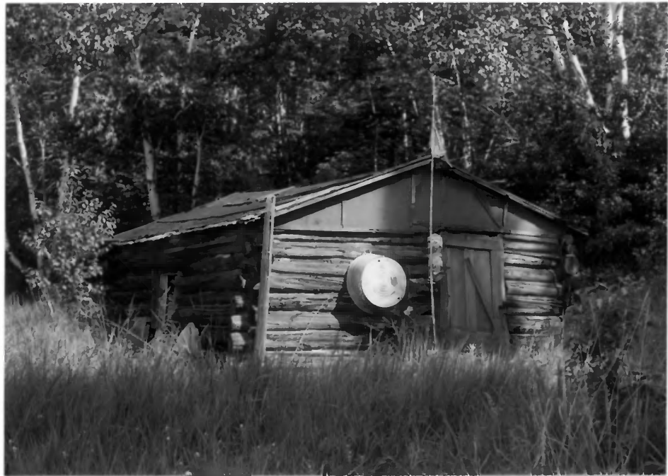
Bunkhouse (HS 14-104C) Manitou Camp Manitou Island, WI
