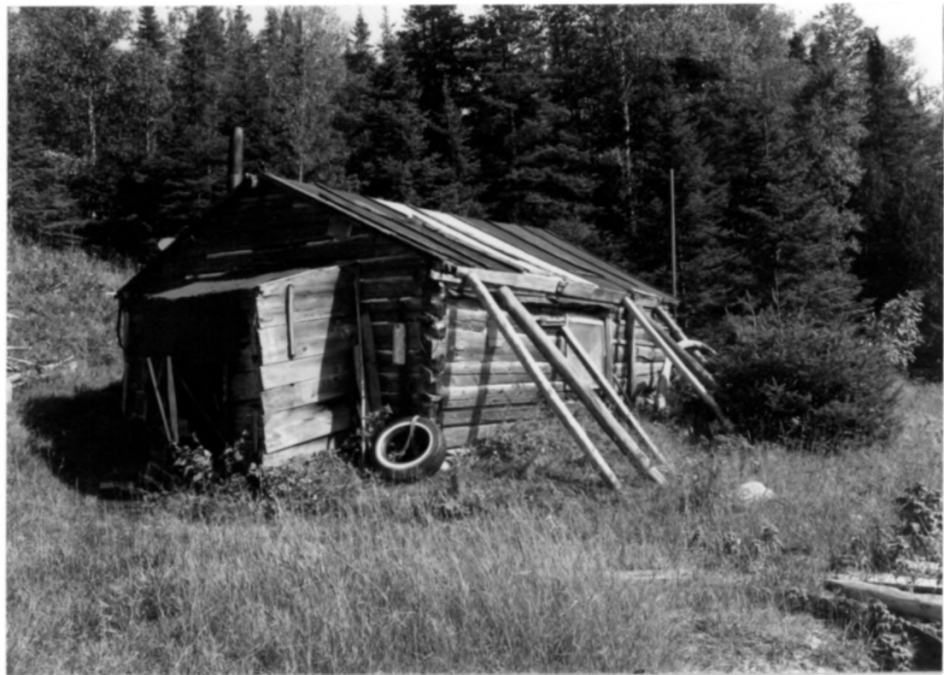
Log Cabin (HS 14-104A) Manitou Camp Manitou Island, WI
