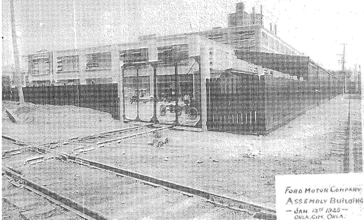
Figure 11. Historic photograph, west and south elevations and train shed, 1925. From the Collections of The Henry Ford, Oklahoma City Branch vertical file. Gift of the Ford Motor Company.
