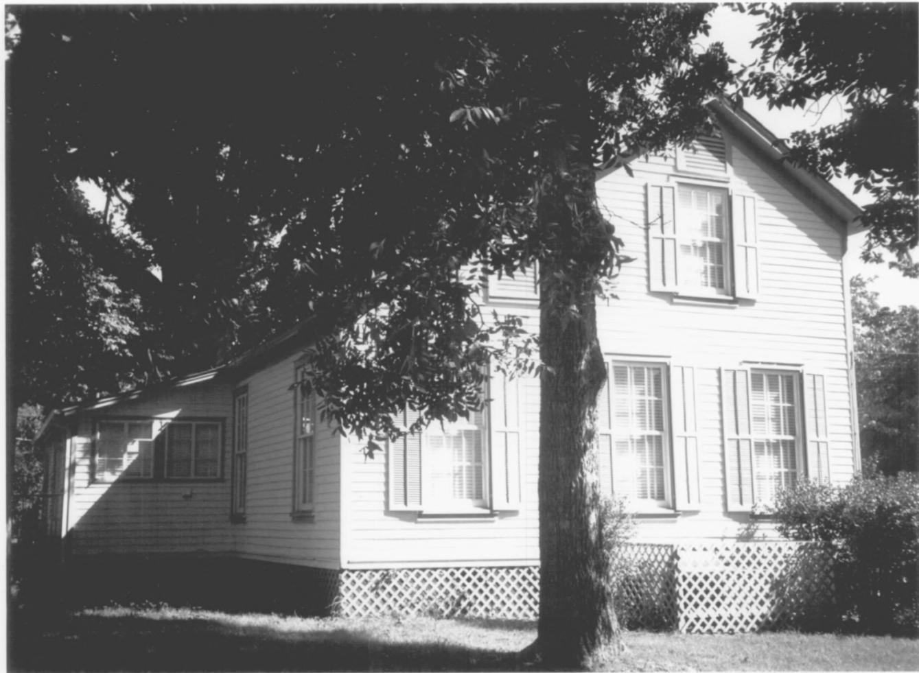
GOTTEN, NICHOLAS, HOUSE SHELBY COUNTY, TN
