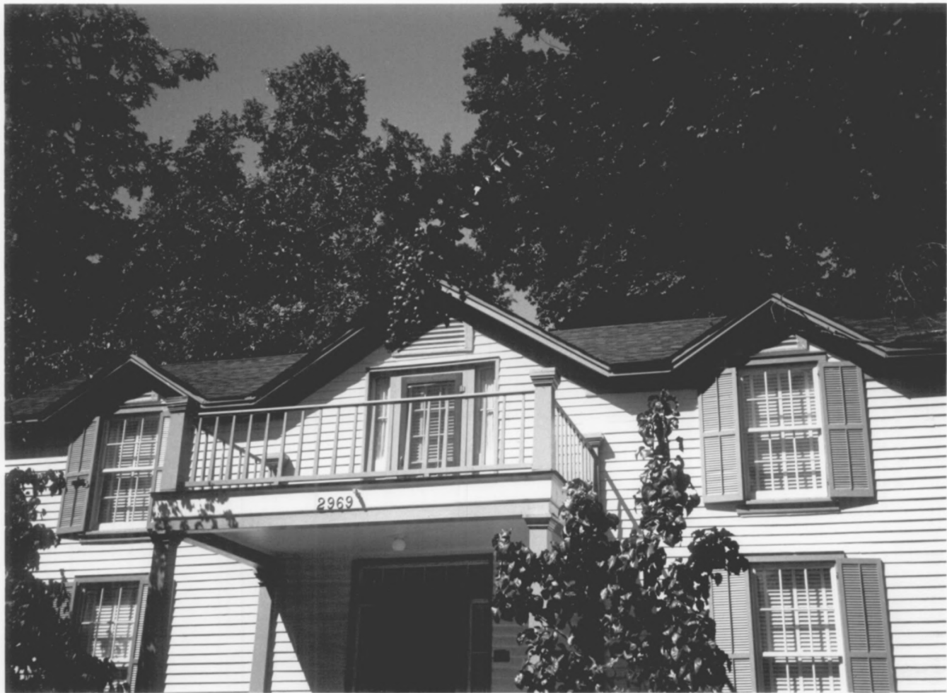
GOTTEN, NIKOLAS, HOUSE SHELBY COUNTY, TN
