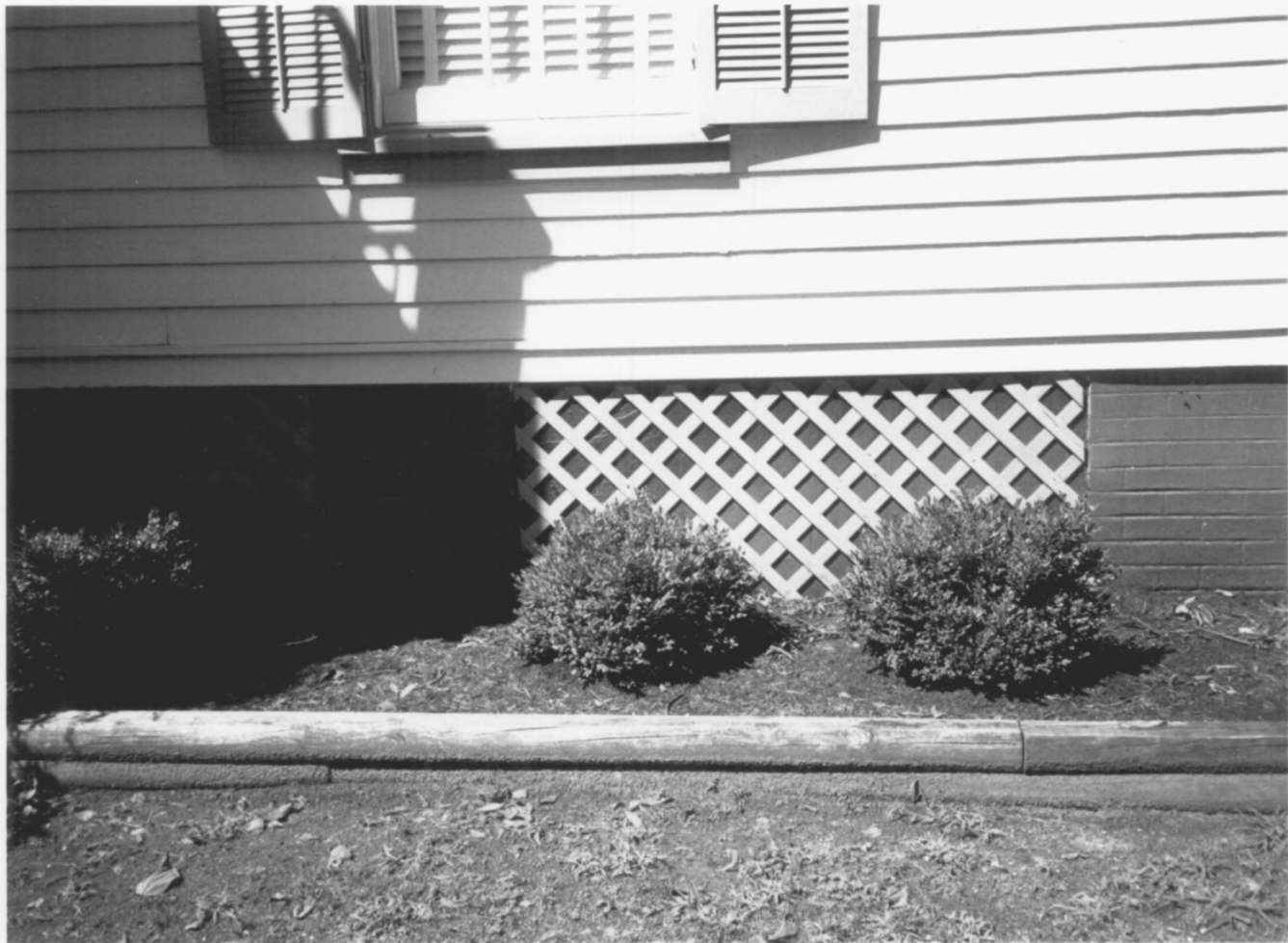
GOTTEN, NICHOLAS, HOUSE → SHELBY COUNTY, TN
