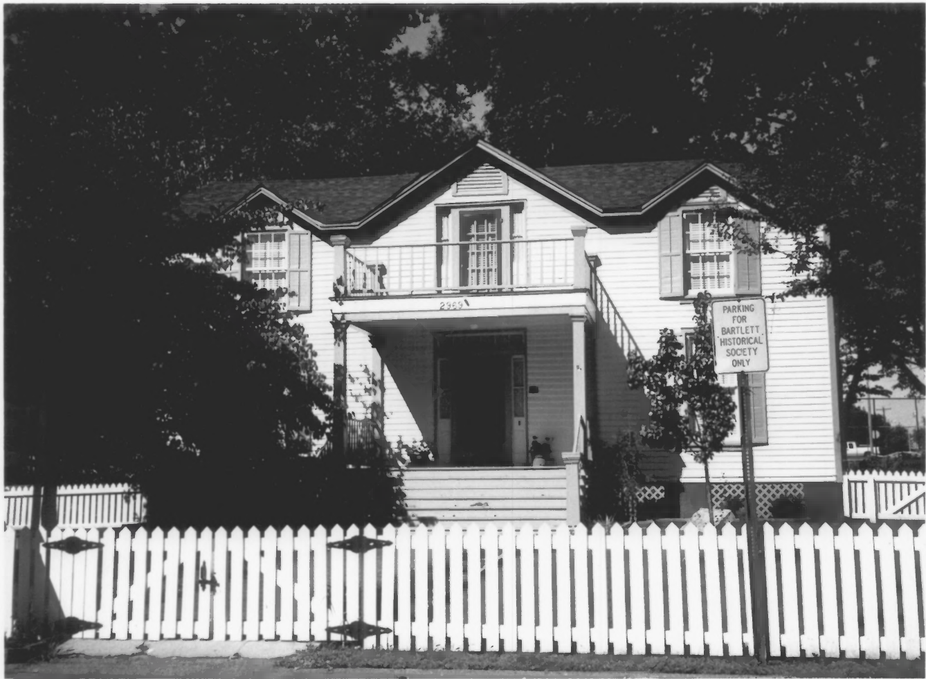
GOTTEN, NICHOLAS, HOUSE SHELBY COUNTY, TN
