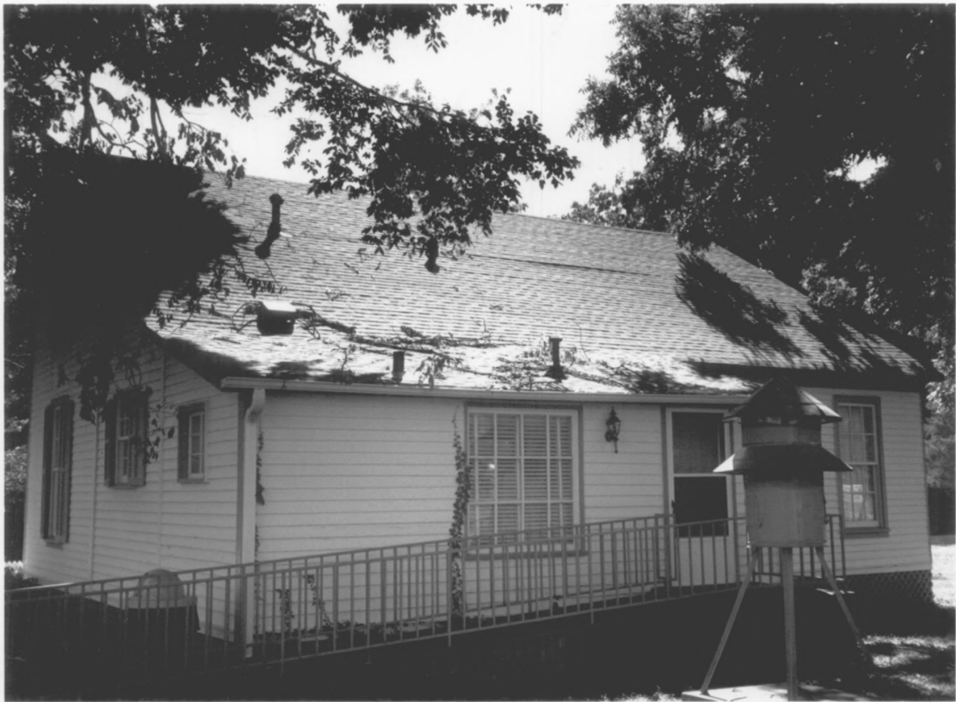
GOTTEN, NICHOLAS, HOUSE SHELBY COUNTY, TN
