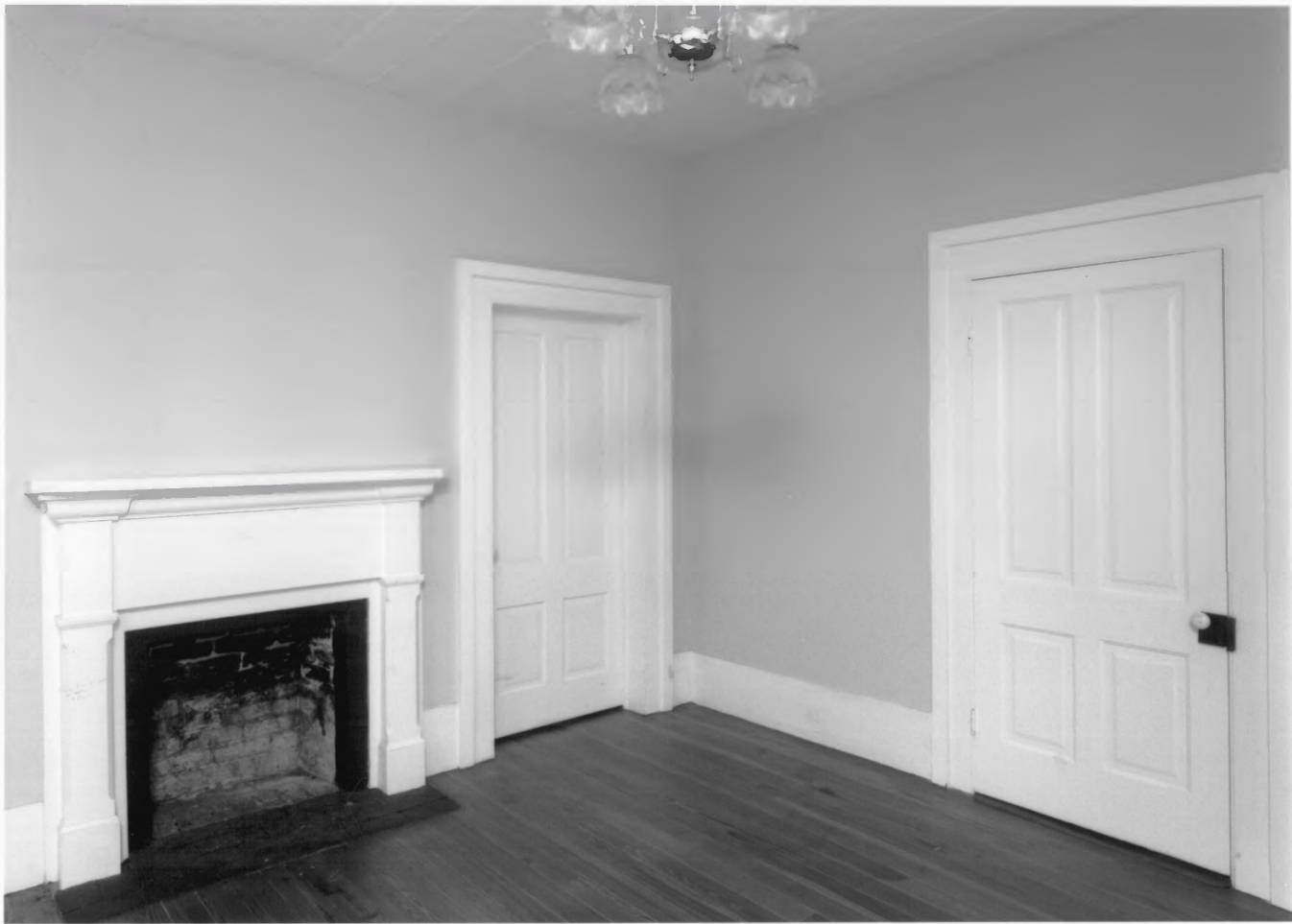
CHAPMAN-STEED HOUSE CRAWFORDVILLE, TALIAFERRO COUNTY, GEORGIA PHOTOGRAPH 8 OF 14
