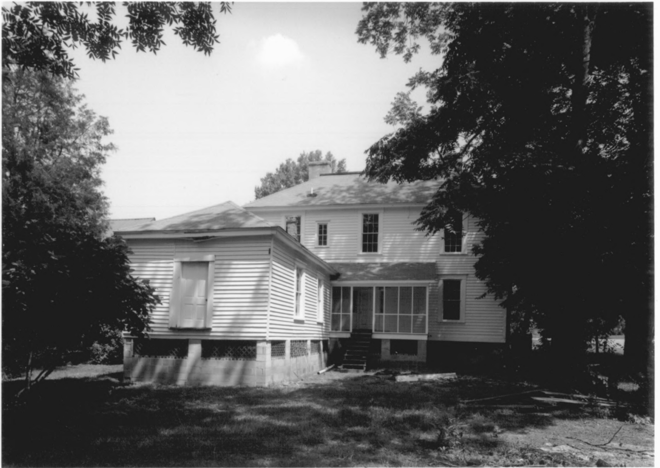
CHAPMAN-STEED HOUSE CRAWFORDVILLE, TALIAFERRO COUNTY, GEORGIA PHOTOGRAPH 3 OF 14
