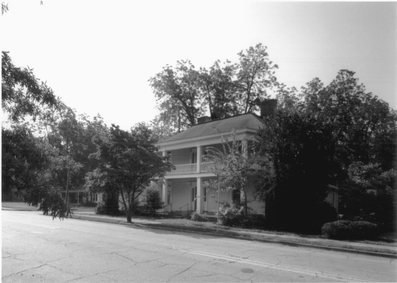
CHAPMAN-STEED HOUSE CRAWFORDVILLE, TALIAFERRO COUNTY, GEORGIA PHOTOGRAPH 14 OF 14
