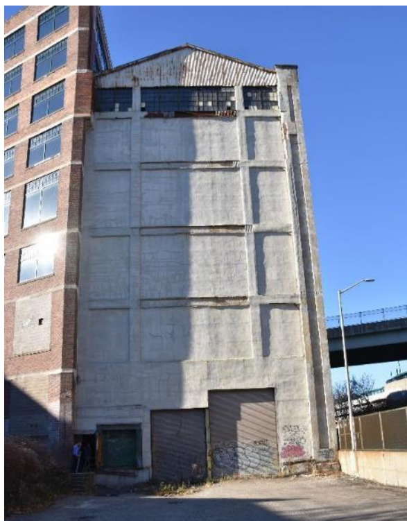
Photo 7: Ford Motor Company Assembly Plant, South elevation of Crane Shed
