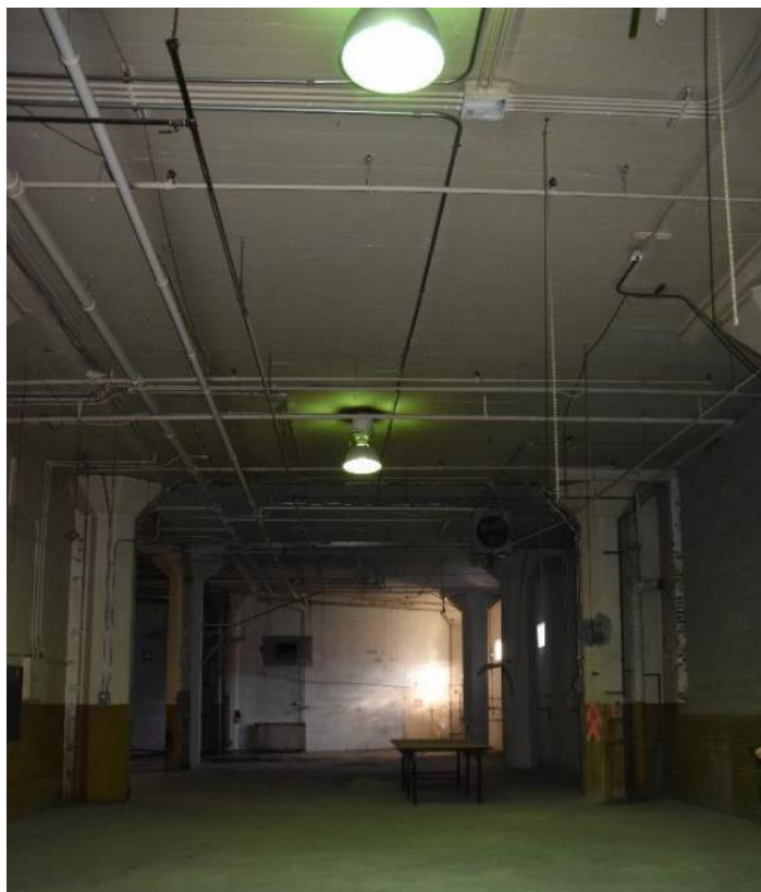
Photo 18: Ford Motor Company Assembly Plant, Basement interior
