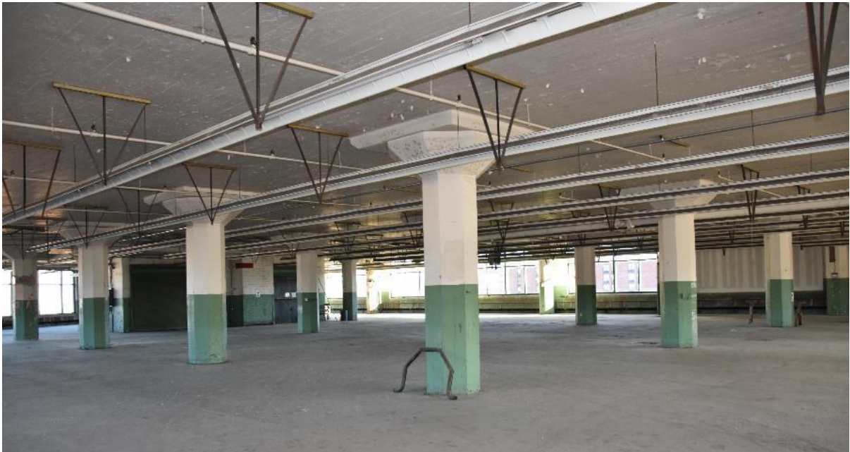
Photo 16: Ford Motor Company Assembly Plant, Fifth floor interior
