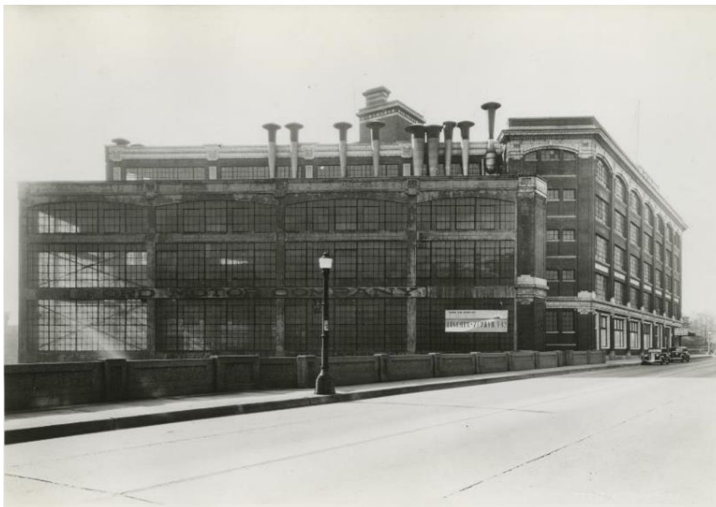
Figure 23: 1942 view of Crane Shed east elevation (left) and Main Building north elevation (right).
