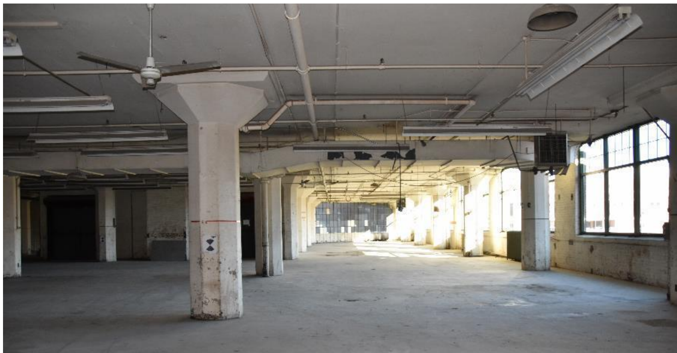
Photo 10: Ford Motor Company Assembly Plant, Second floor interior
