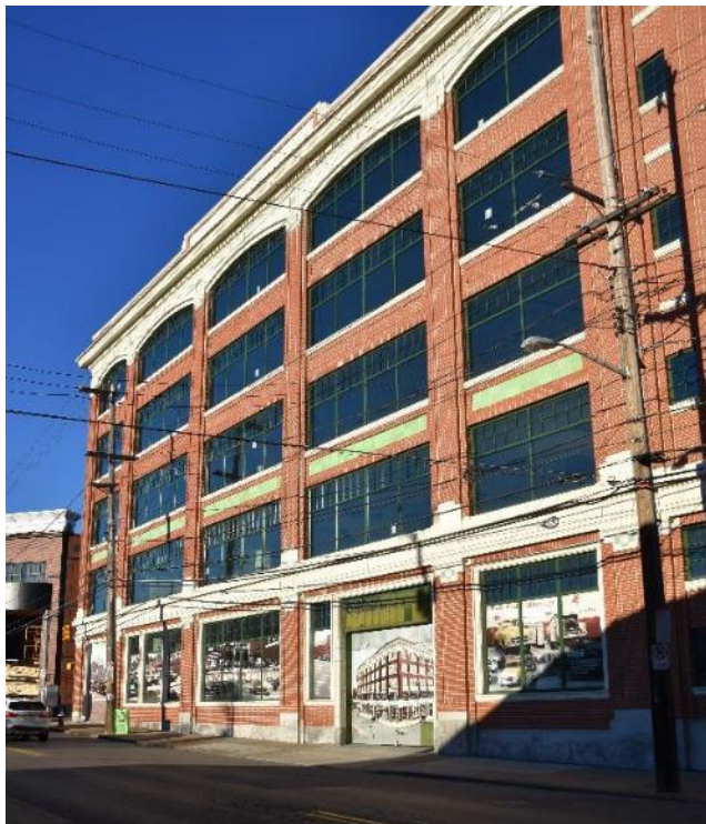
Photo 6: Ford Motor Company Assembly Plant, East elevation
