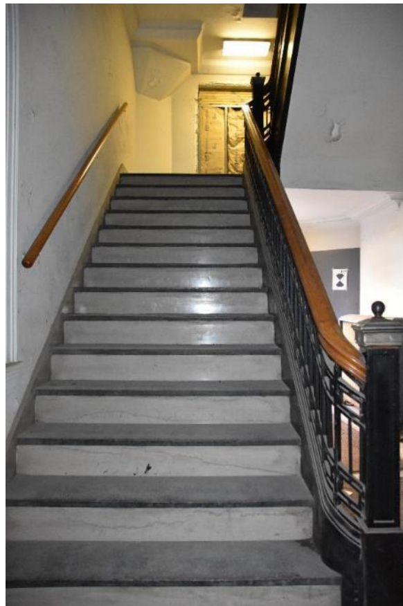
Photo 17: Ford Motor Company Assembly Plant, Main stair
