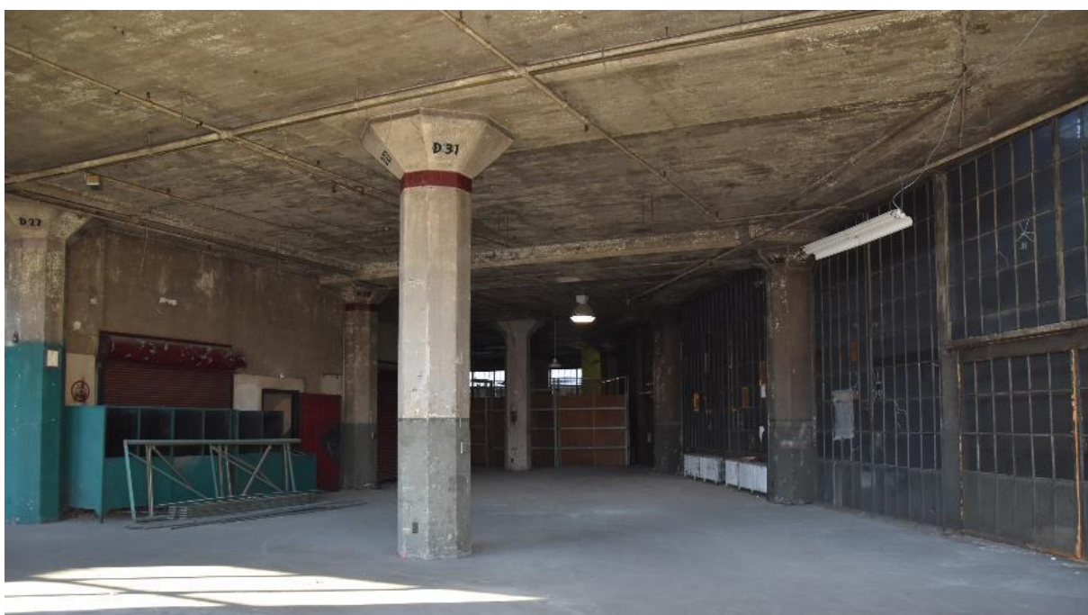
Photo 9: Ford Motor Company Assembly Plant, First floor interior
