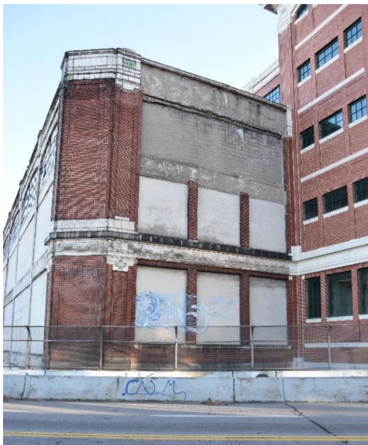
Photo 5: Ford Motor Company Assembly Plant, North elevation of Crane Shed
