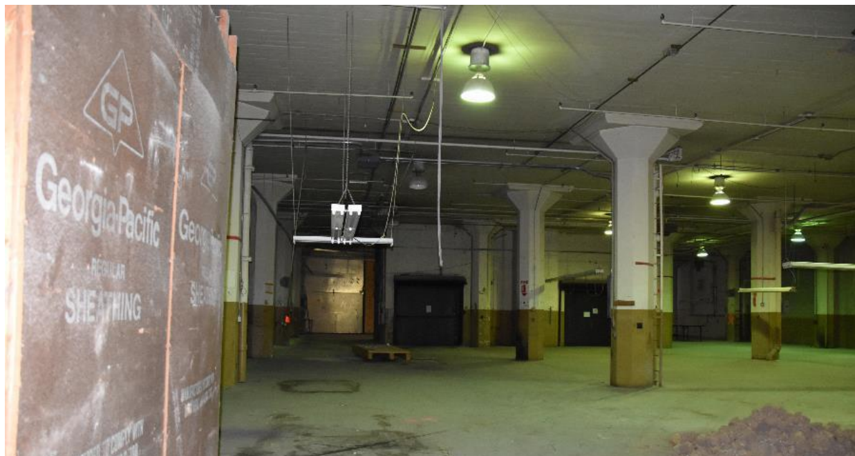
Photo 19: Ford Motor Company Assembly Plant, First subbasement interior
