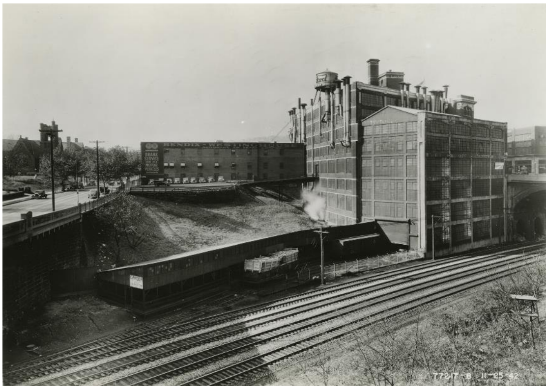
Figure 24: 1942 view south (left) and east (right) elevations.
