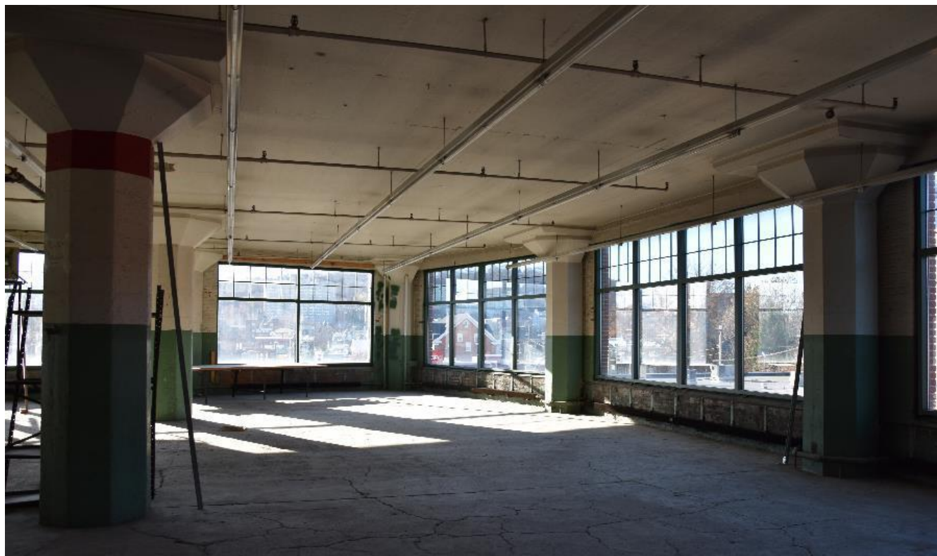
Photo 11: Ford Motor Company Assembly Plant, Third floor interior
