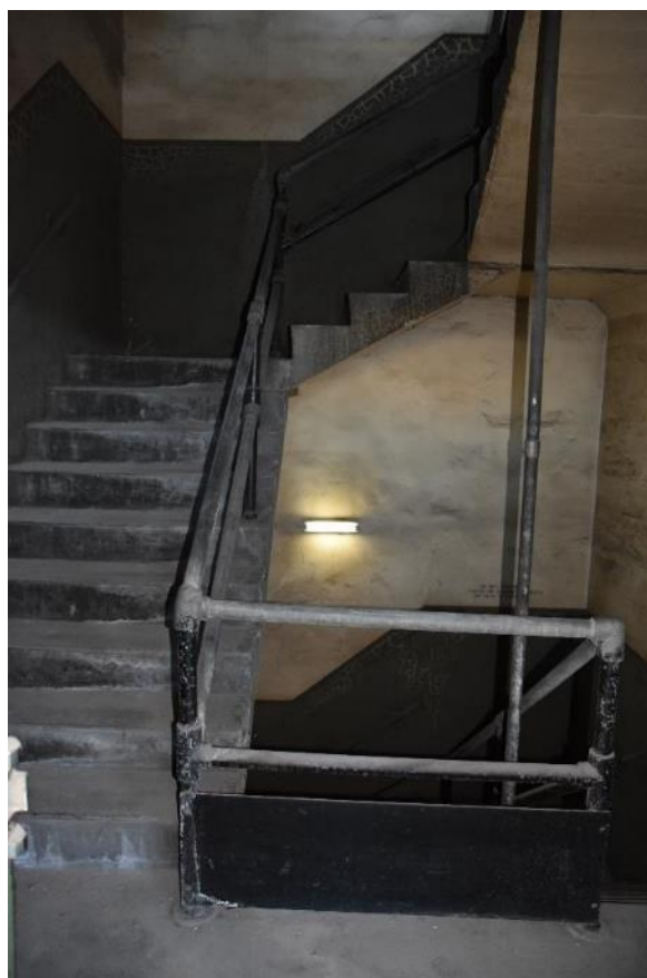
Photo 13: Ford Motor Company Assembly Plant, Secondary stair
