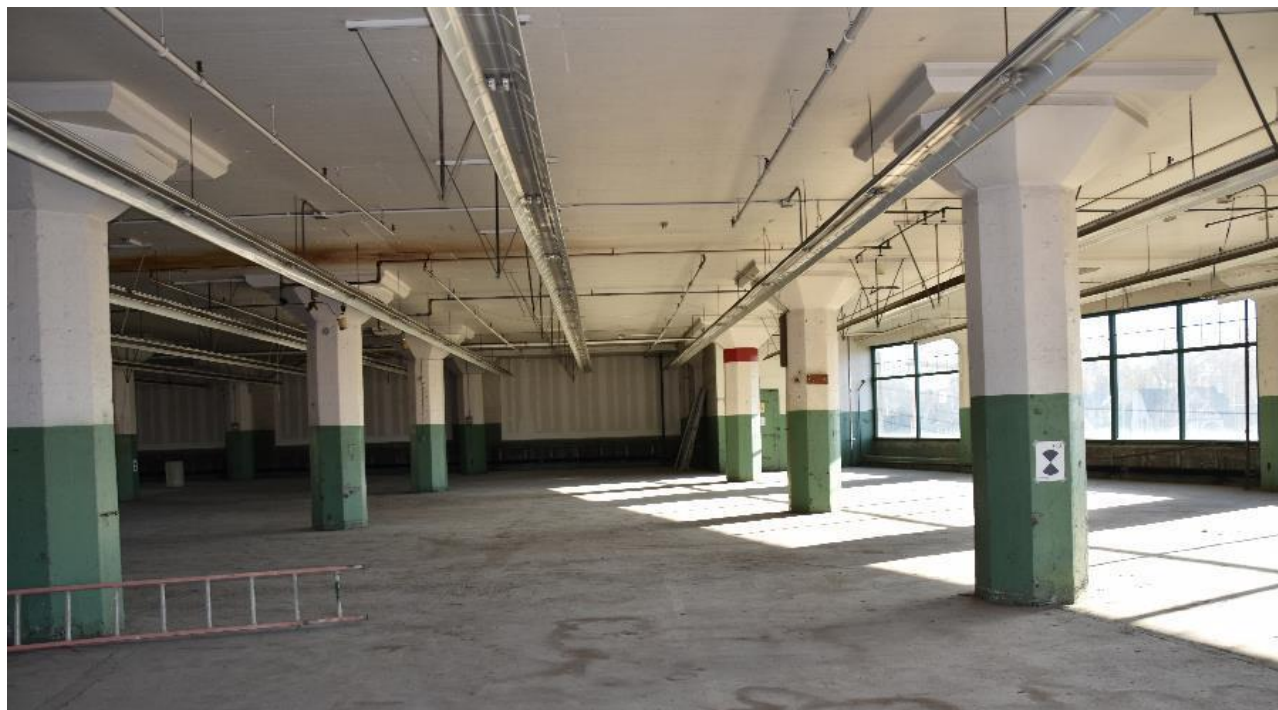
Photo 14: Ford Motor Company Assembly Plant, Fourth floor interior
