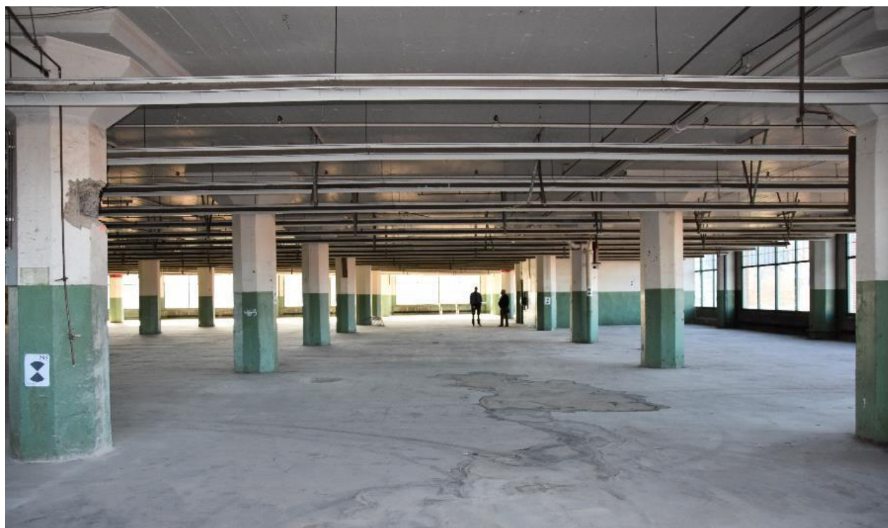
Photo 15: Ford Motor Company Assembly Plant, Fourth floor interior
