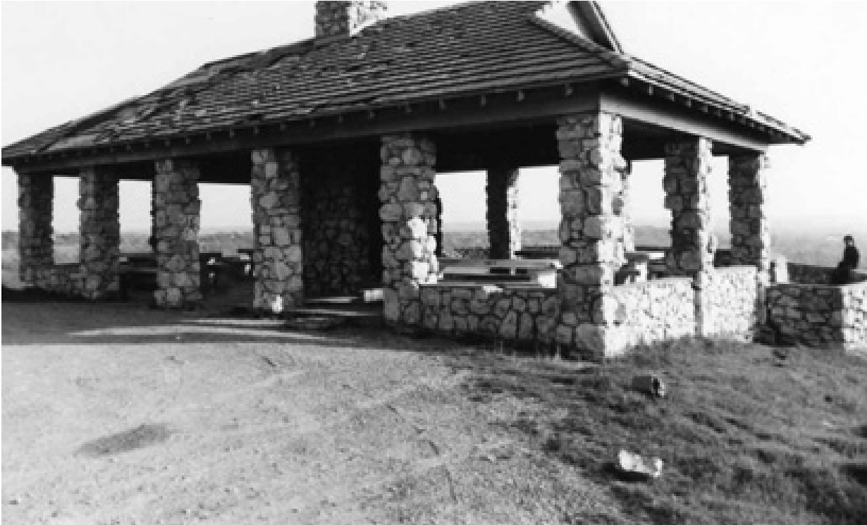
Figure 6: Undated historic photo, taken prior to the 1986 fire which left the shelter house without its roof.
