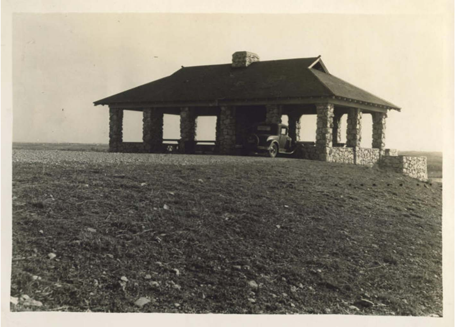
Figure 4: Inspiration Point Shelter House, as viewed from the northwest, shortly after construction, c. 1927.
