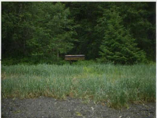
Figure 3b: Windfall Harbor Shelter Cabin from Beach (FS 2006 Photo 06170022.JPG)
