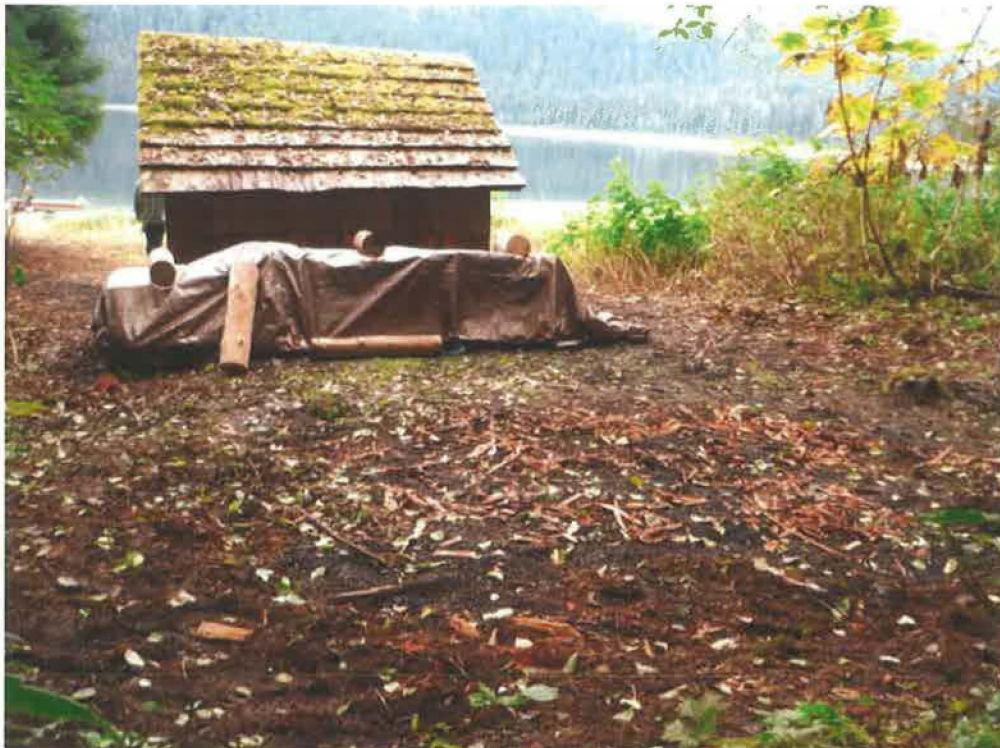
Photo taken September 2014 following the shelter move. View of the rear façade of the shelter moved to the more exposed beach location.
