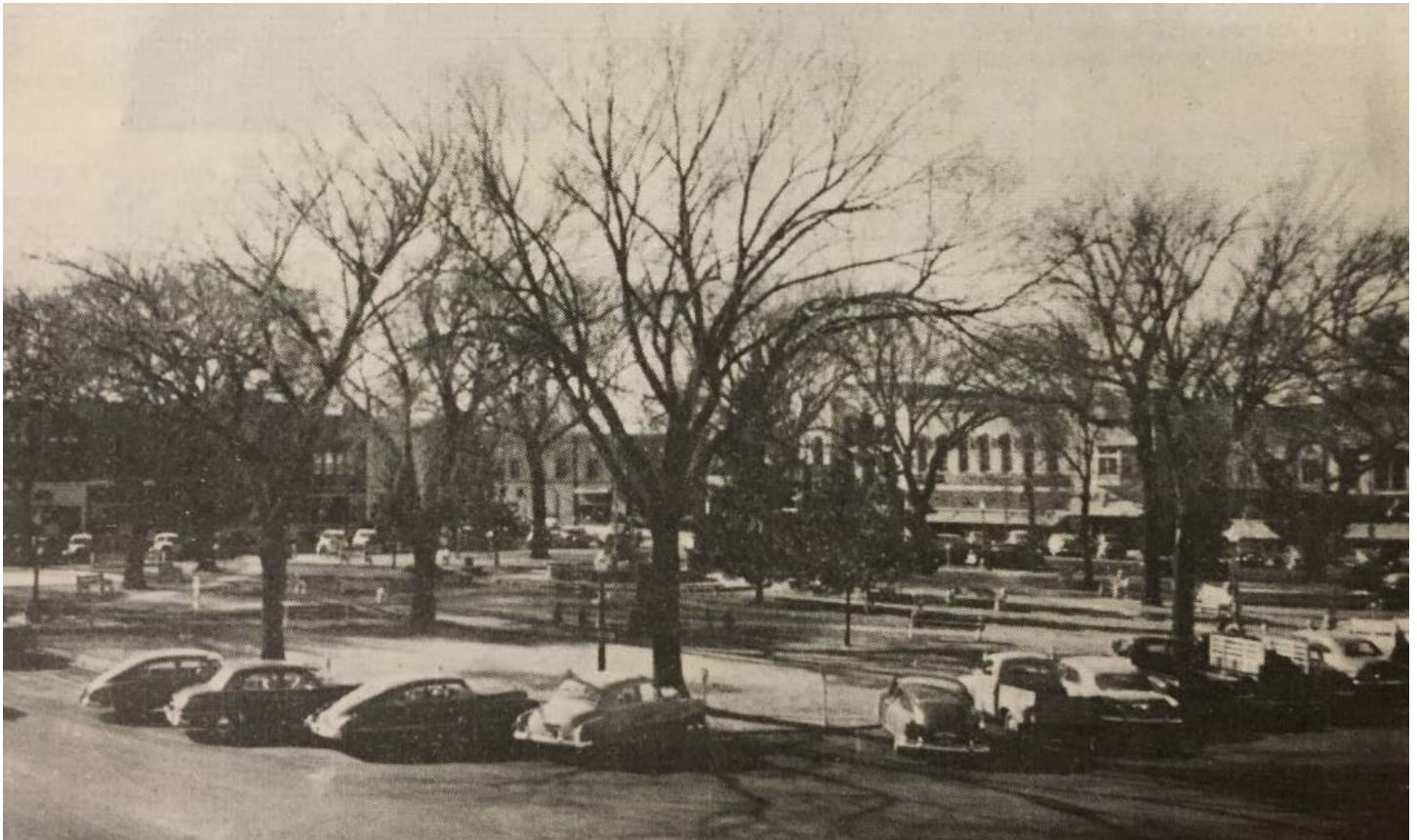
Figure 15: Looking across Fountain Square. Reprinted from SAC-GCC Counselor December 1952
