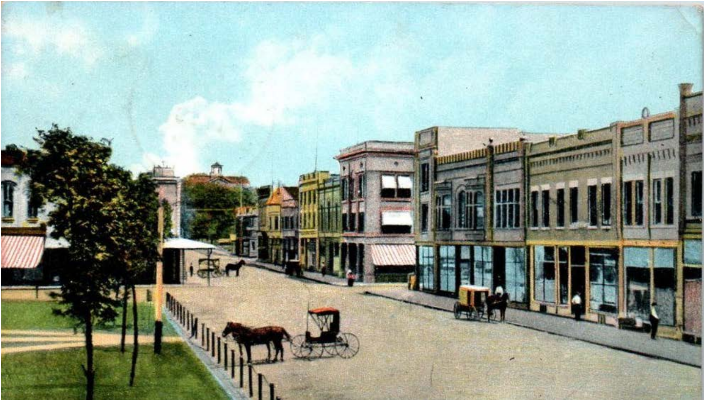
Figure 9: A Postcard View of the South Side of the Square looking east on Coolbaugh Street in 1908, after reconstruction.
