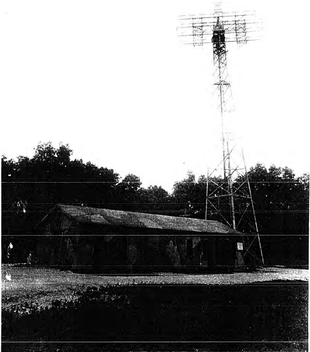
28. Radio Set SCR-271-D at the Evans Signal Laboratory showing shelter for components and operating personnel, 100ft. tower, and antenna modified for PPI display. IFF antenna is shown top-center on radar antenna.
