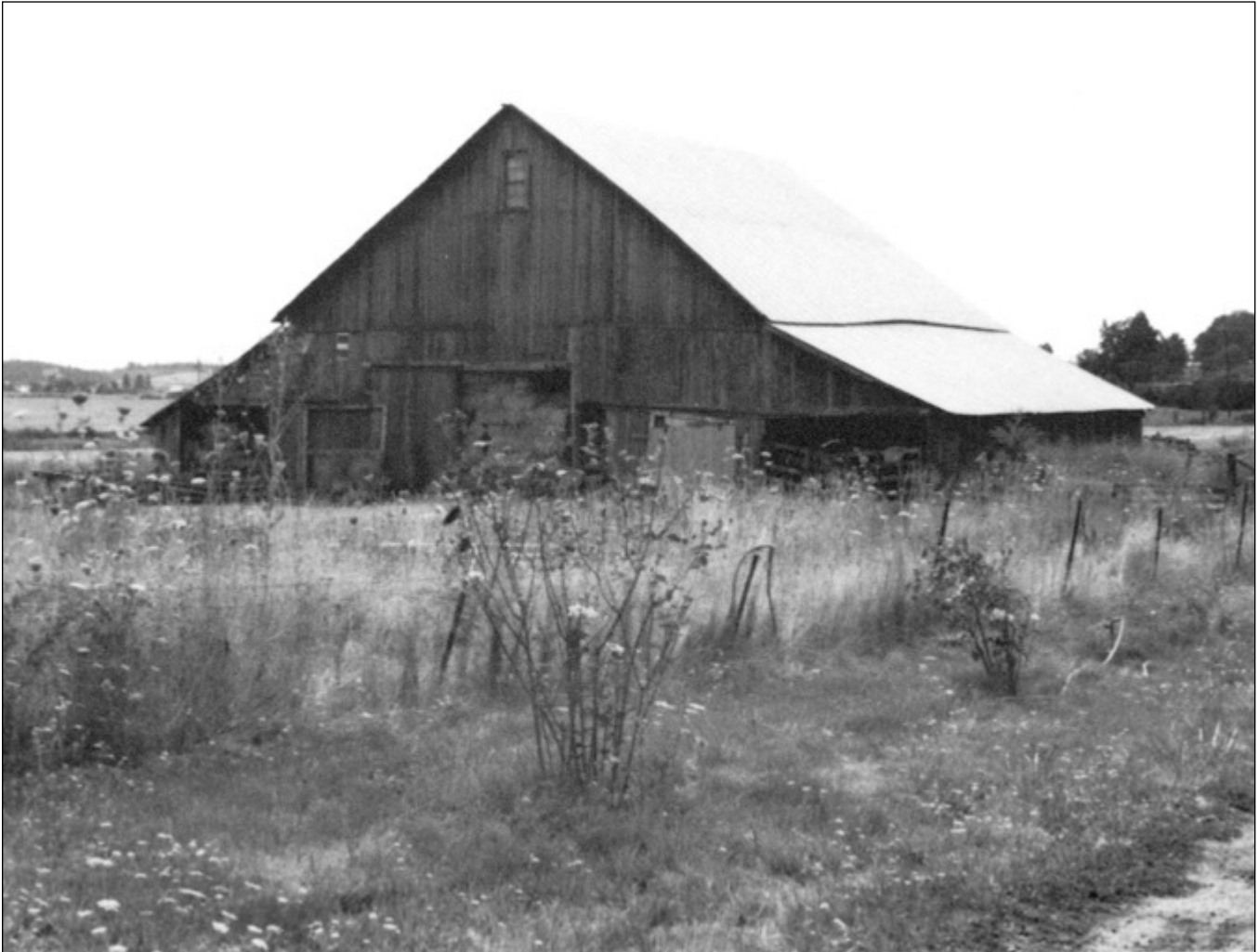
Figure 35: The W.D. Clark Barn (now demolished), as it appeared in 1984.
