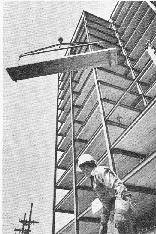
A section of concrete floor planking reaches for destination.
