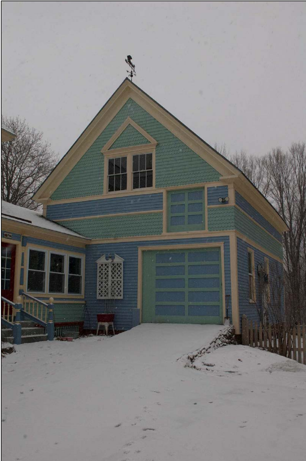
Photo 0003: George Washington Noyes House, showing south façade of barn. Facing north.
