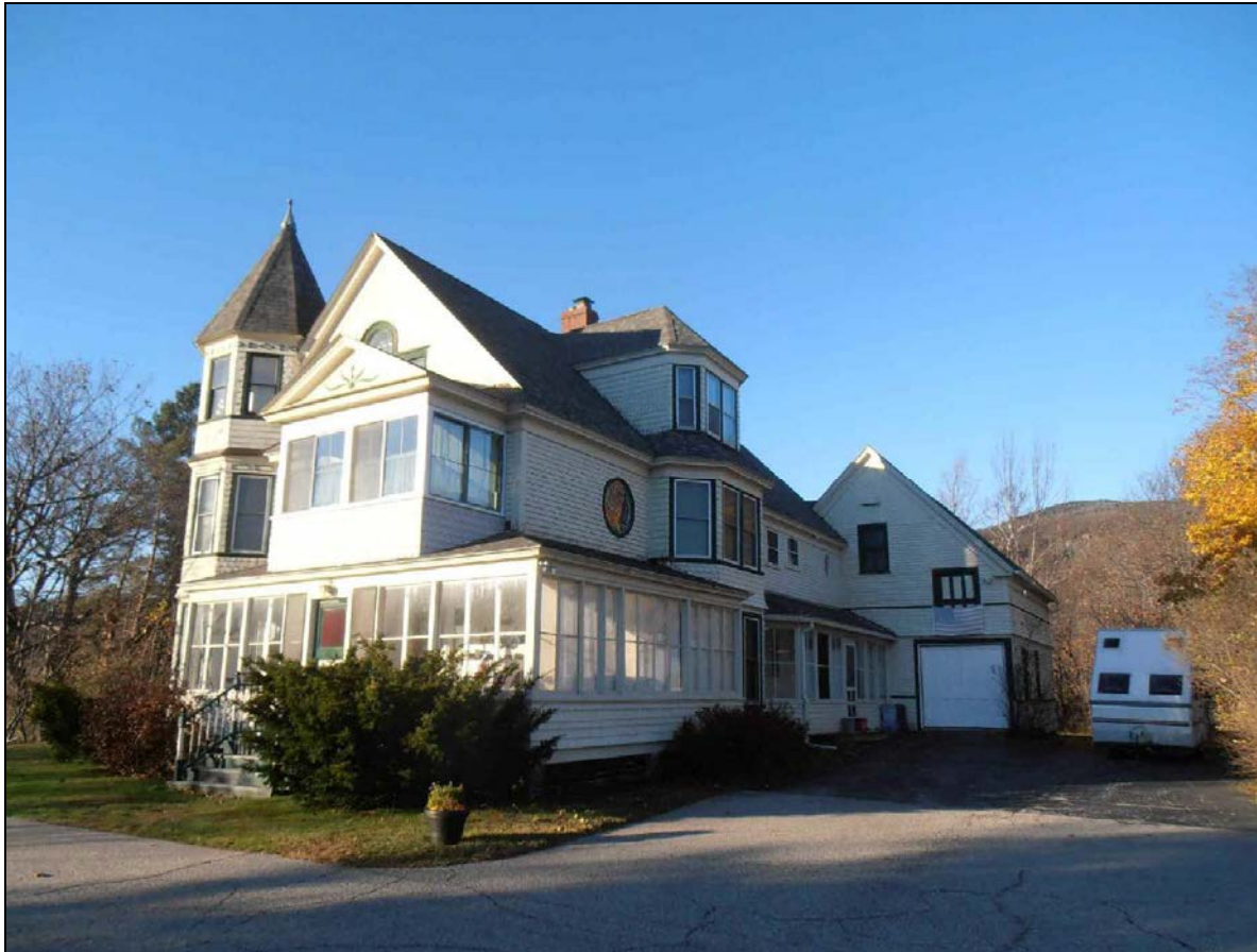
Figure 3: A. B. Libby House, 6 Prospect Terrace 1892 A. B. Libby House, also designed by F. P. Burbank and constructed near the George Washington Noyes House. Photograph from 2015 Tax Card.
