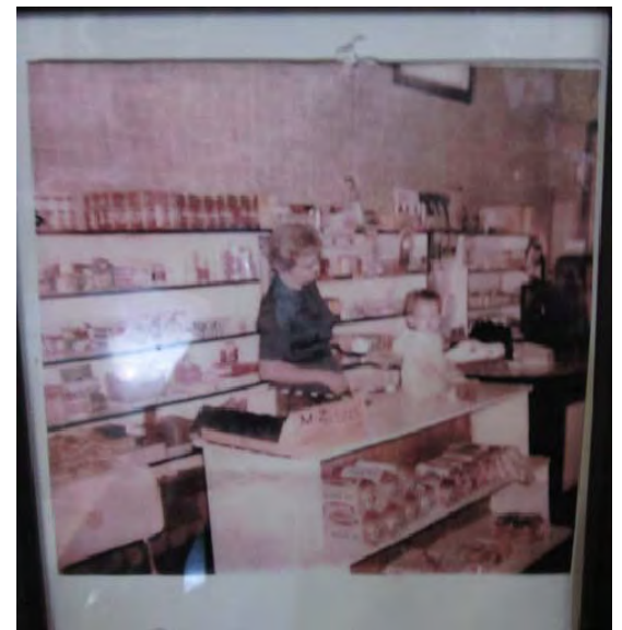
Pottsville General Store and Gulf Gas Station ca. 1960, on display at Marcy Jo’s Mealhouse
