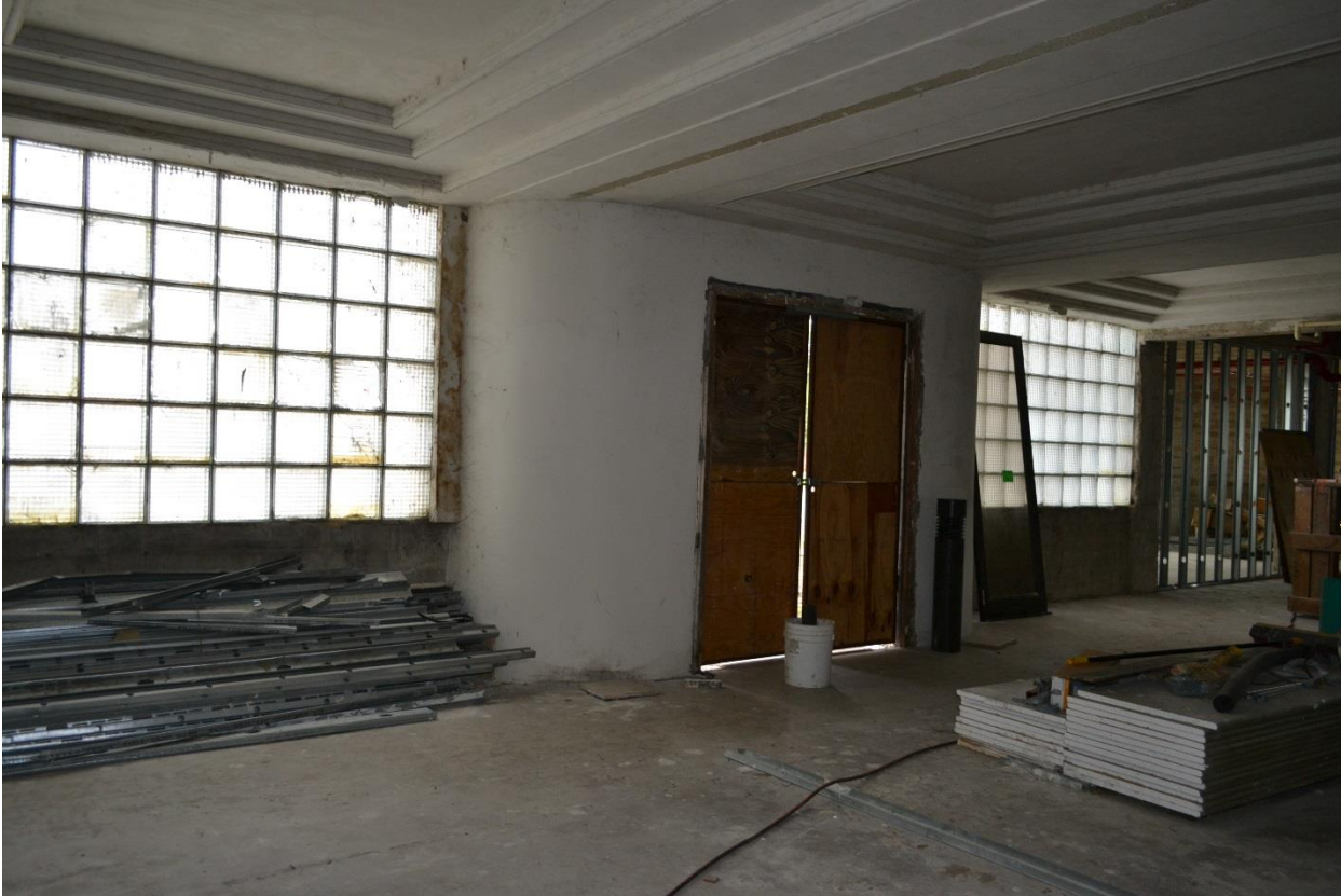
Photo 7 – First floor lobby, view northeast. Original recessed ceiling details and front door openings remain in place with the glass block.
