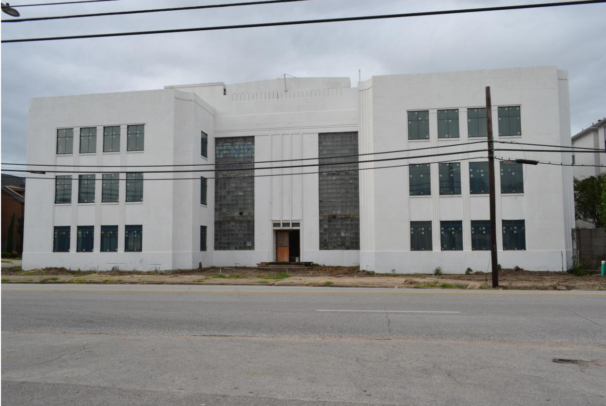
Photo 1 – North façade, view south, with original glass block, exterior fluting, and fenestration pattern.
