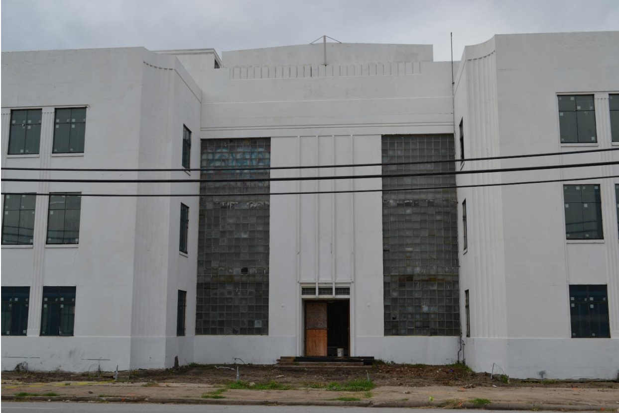
Photo 5 – Detail of entrance on north façade, view south. Original fluting, glass block, dentils, and flag pole remain in place.
