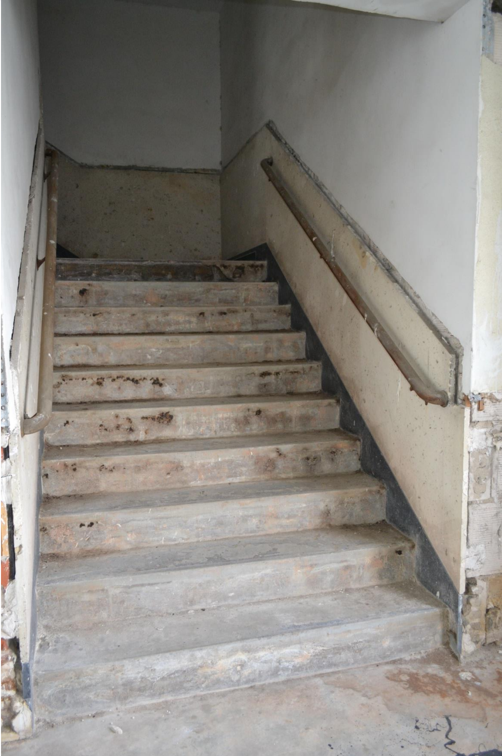
Photo 9 – Stair detail, view east. Original handrails, fossilized limestone wainscot, and black stone stringers remain in place.
